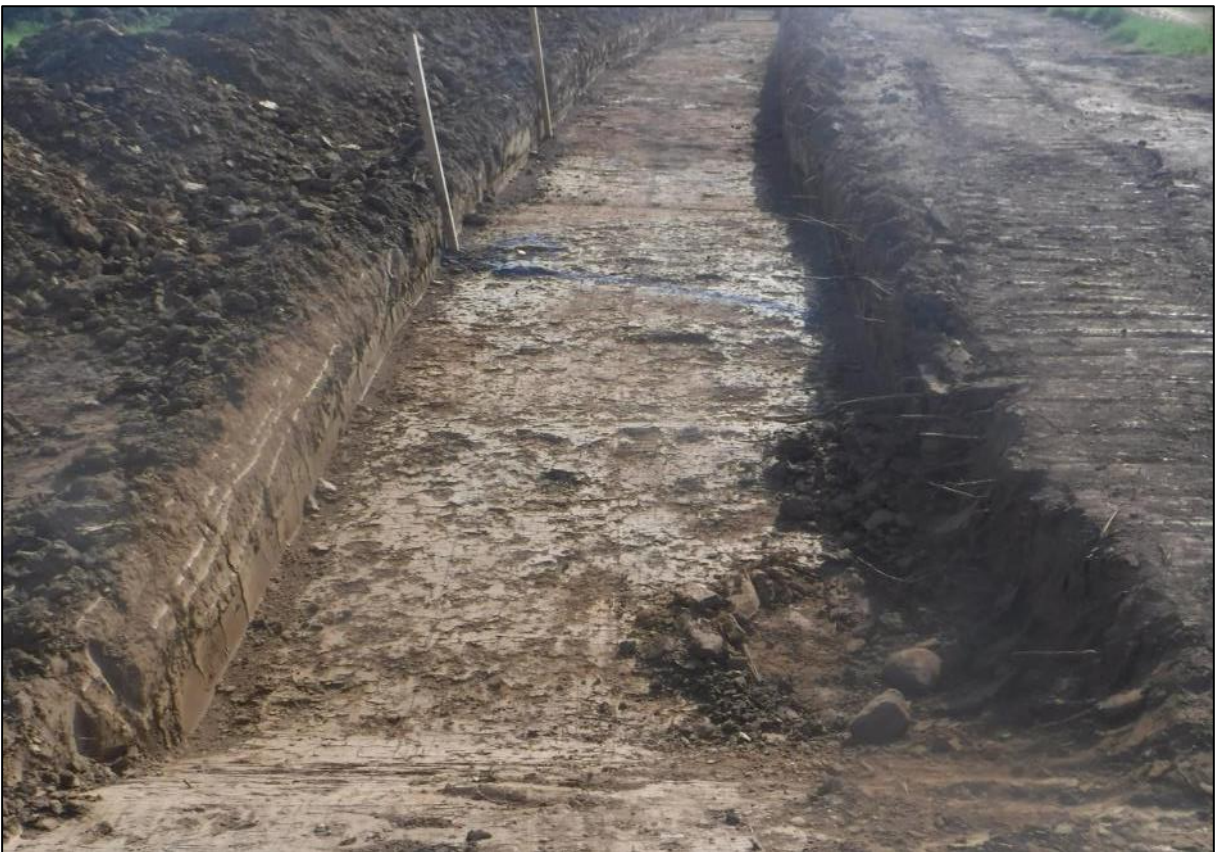
Plate 20. Area C, looking east-northeast.
