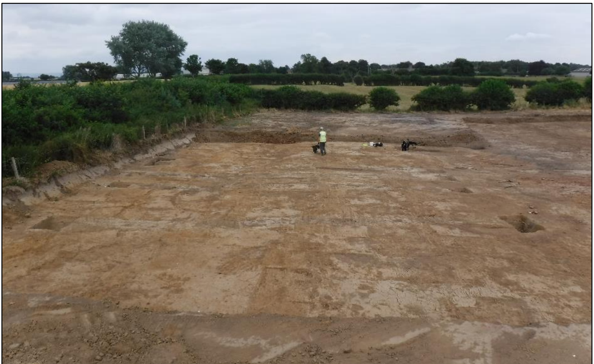
Plate 12. Working shot of northern part of Area A showing northwest-southeast aligned ditches, looking northeast.
