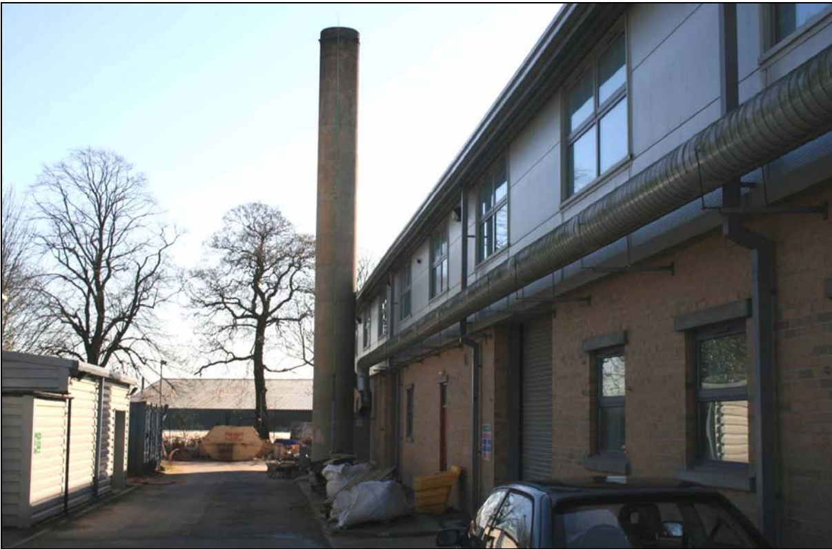
Plate 3. Example of College building, with boiler room chimney.
