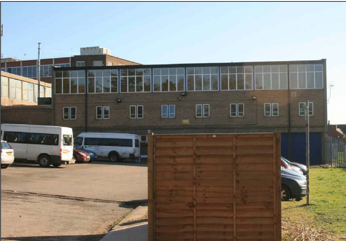
Plate 4. College building and car park.
