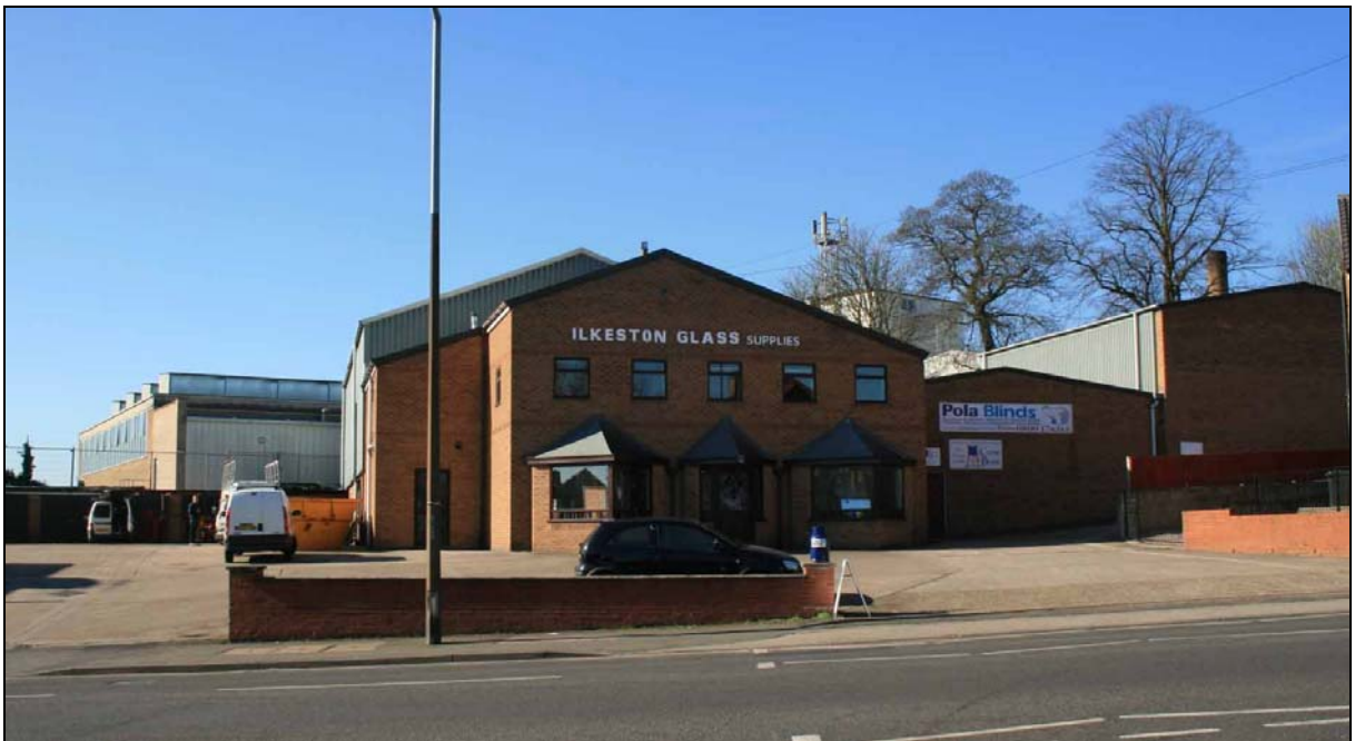
Plate 10. Ilkeston Glass with College buildings beyond.
