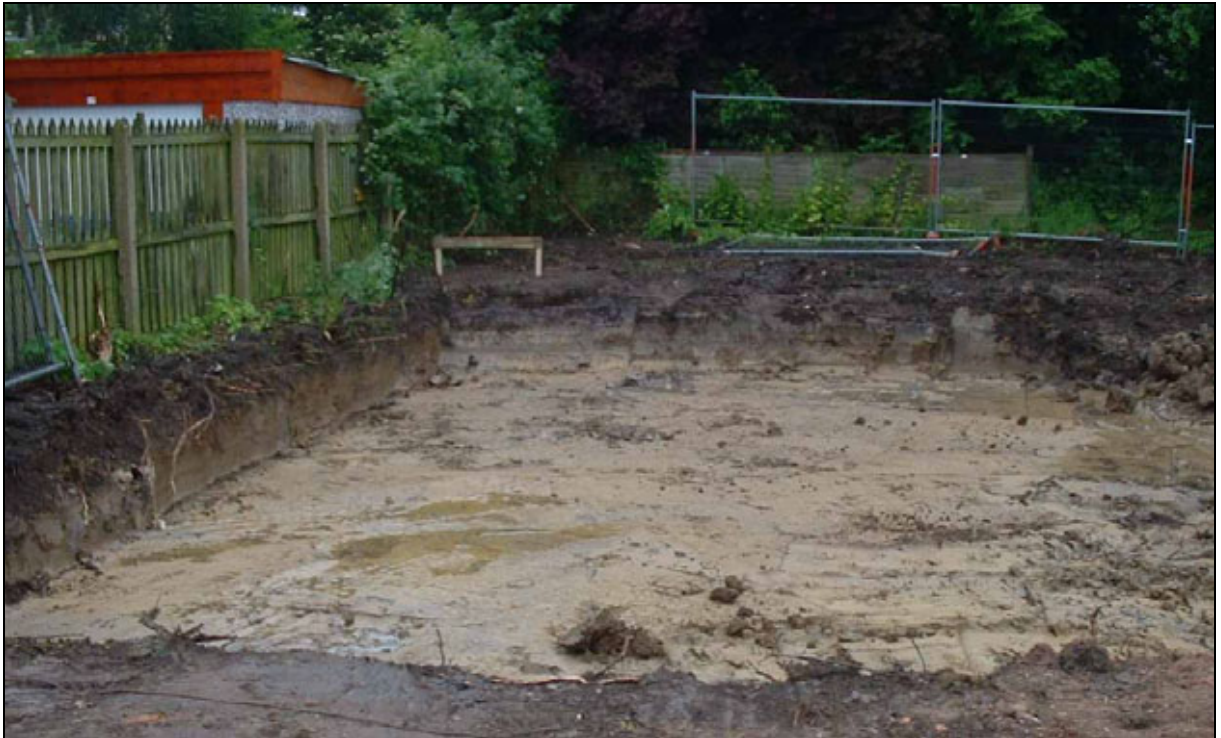
Plate 1. General view of site looking south
