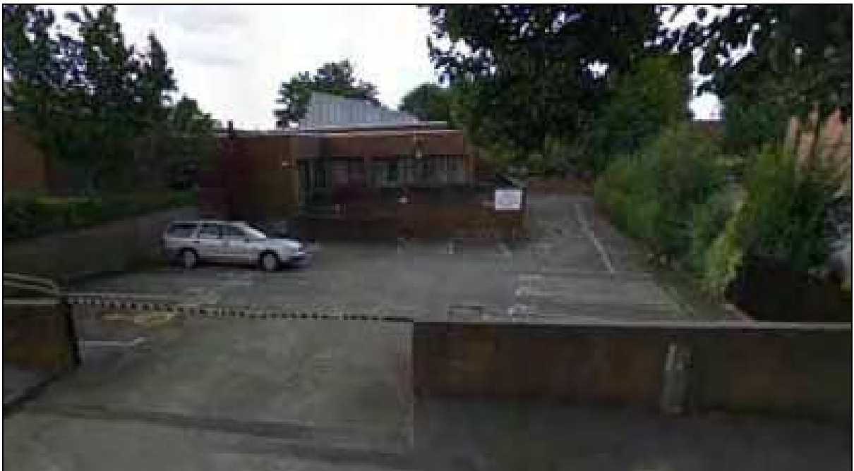
Plate 6. Car park at northern end of site.
