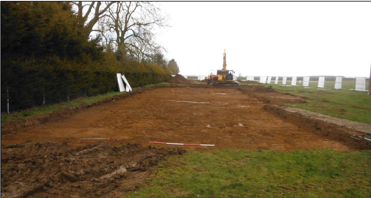
Plate 3. Block A, looking east.
