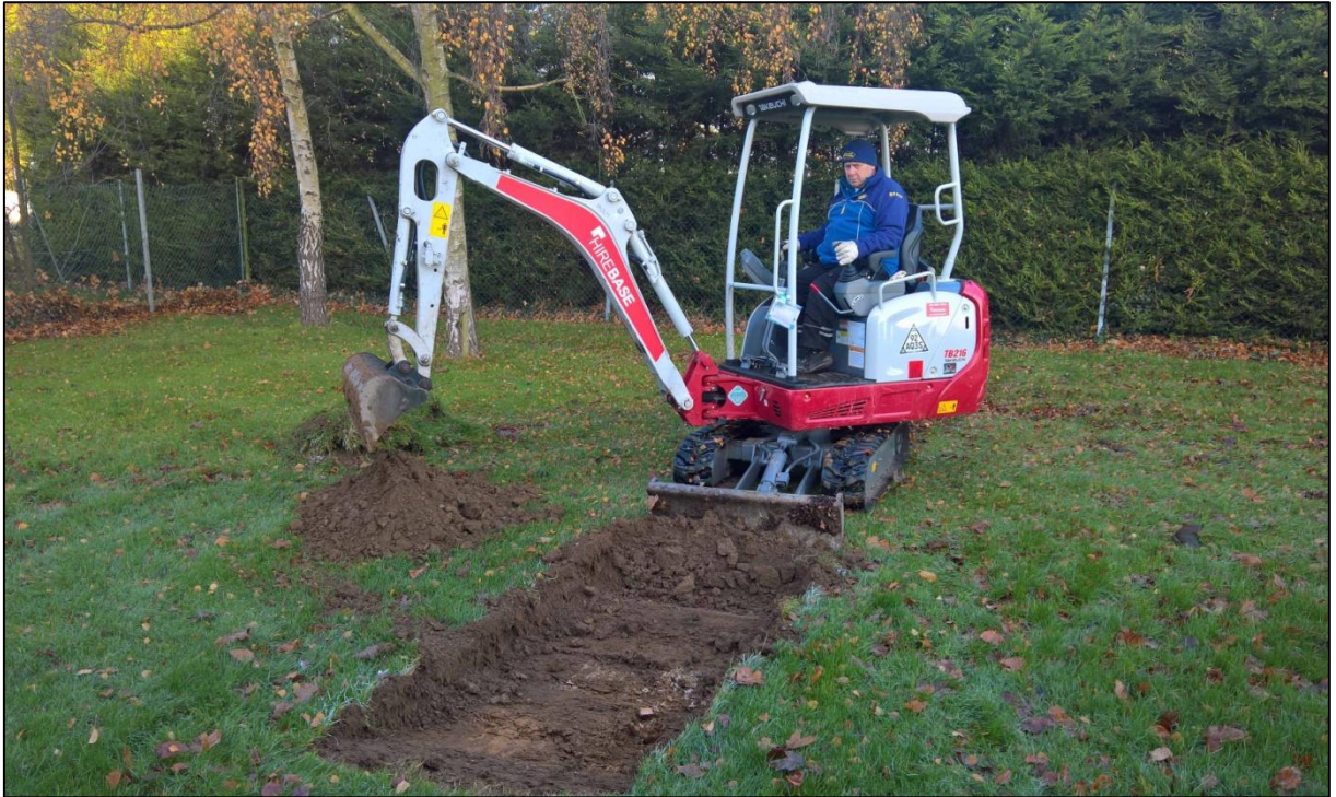
Plate 1. Test pit excavation, working shot.
