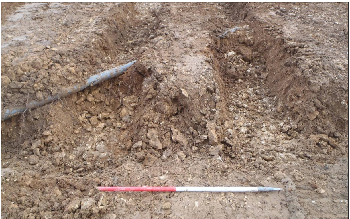
Plate 6. Block B, foundation trenches showing natural and modern service duct.
