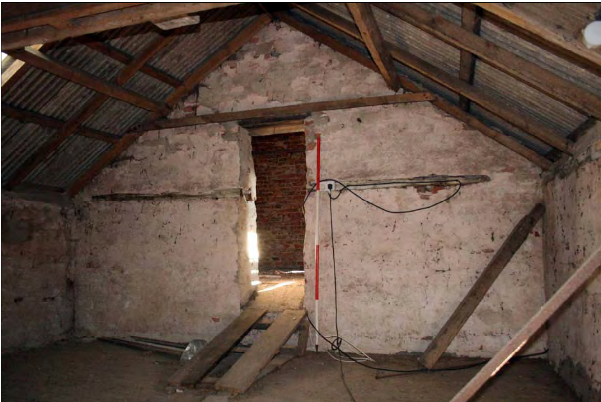
Plate 42. B3 interior first floor looking SW (image no. 044).
