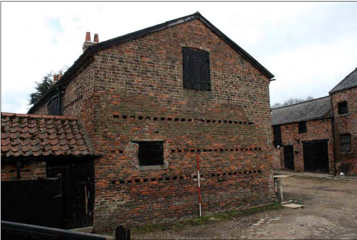
Plate 53. B5 exterior looking west (image no. 426).
