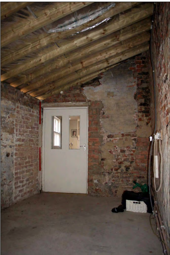
Plate 30. B2 interior SE bricked up doorways looking southeast (image no. 217).
