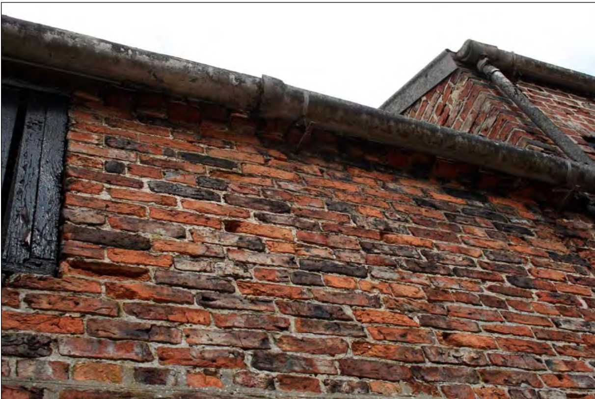
Plate 34. B3 and B4 exterior dentilated eave looking NE (image no. 371).
