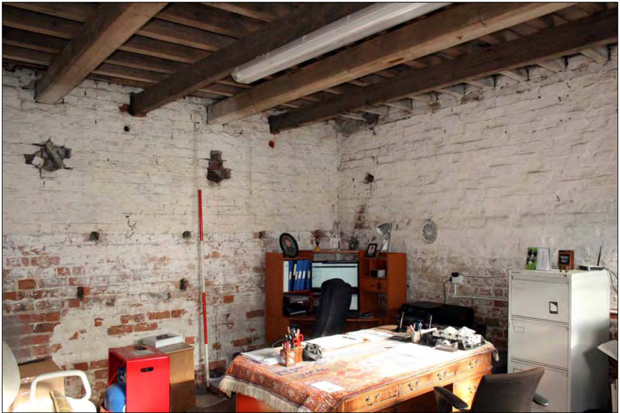
Plate 15. B1 interior ground floor looking north (image no. 124).
