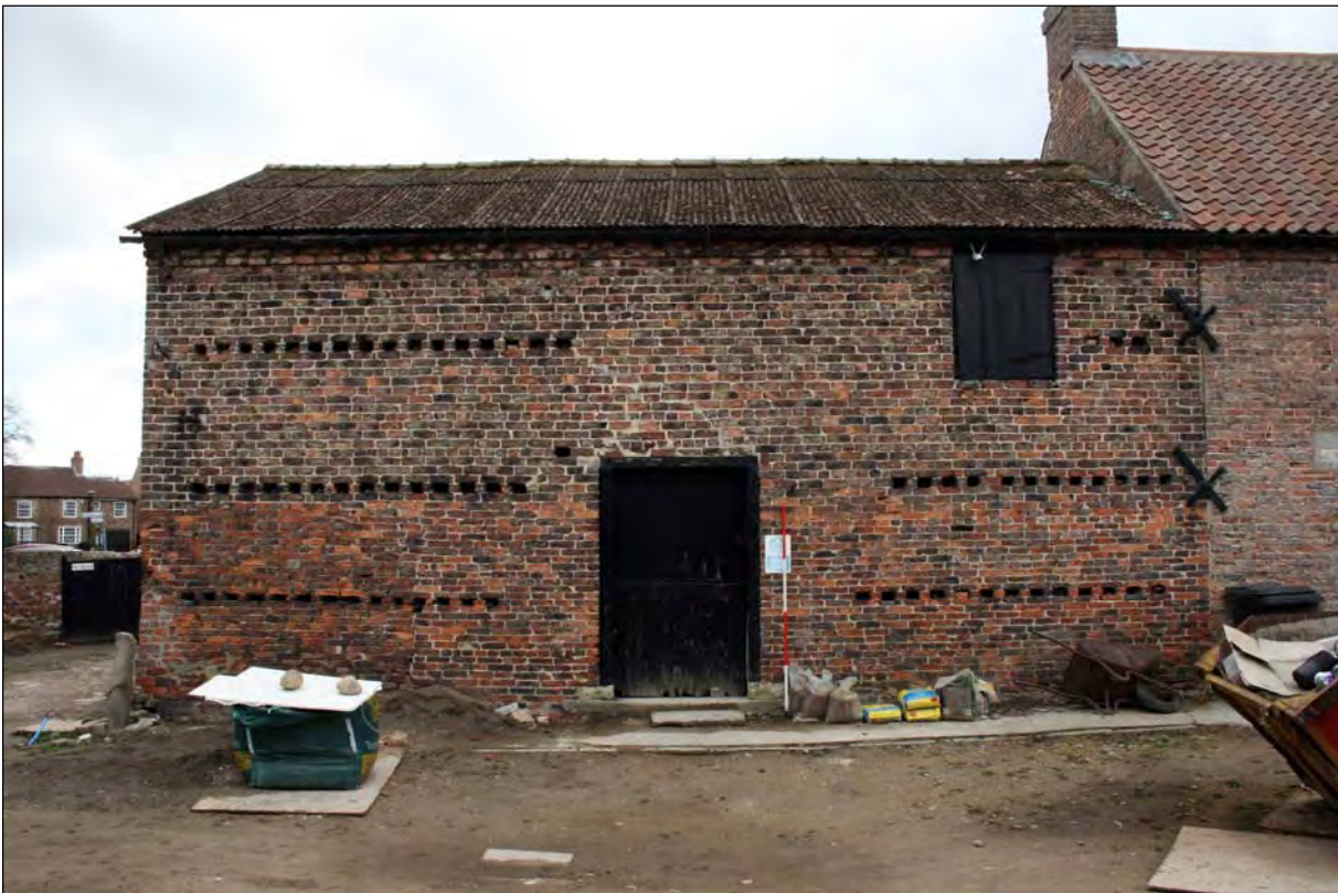
Plate 54. B5 exterior looking southeast (image no. 410).
