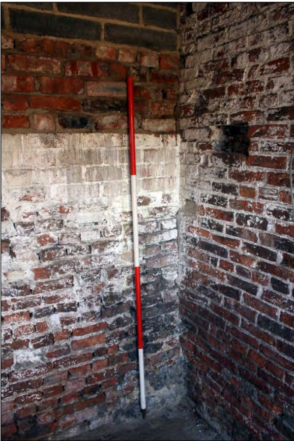
Plate 29. B2 interior NW looking west (image no. 249).
