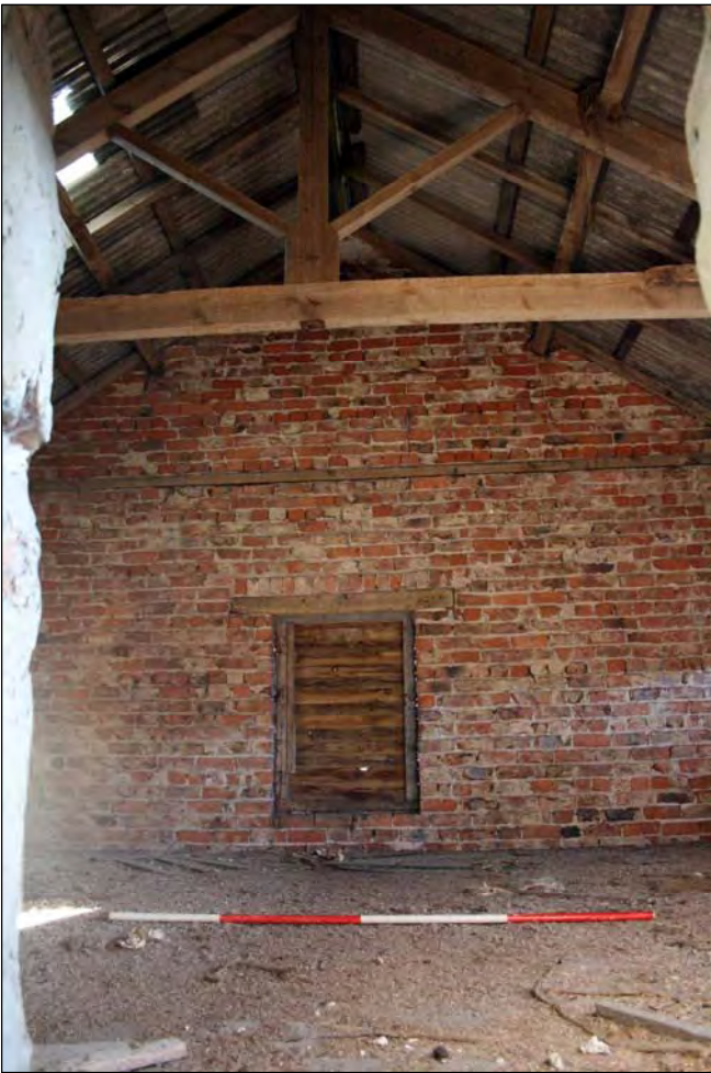
Plate 9. B1 interior looking NE (image no. 002).
