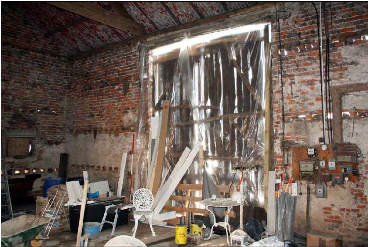
Plate 57. B5 interior looking east (image no. 296).
