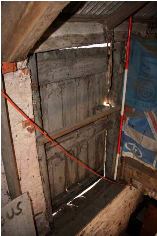
Plate 43. B3 interior first floor loft door looking south (image no. 080).
