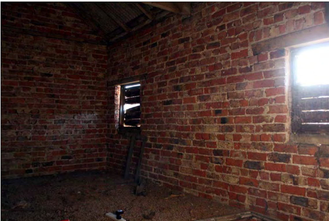
Plate 10. B1 interior looking east (image no. 014).
