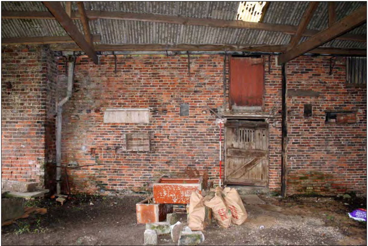
Plate 39. B3 and B4 exterior NE looking southeast (image no. 337).
