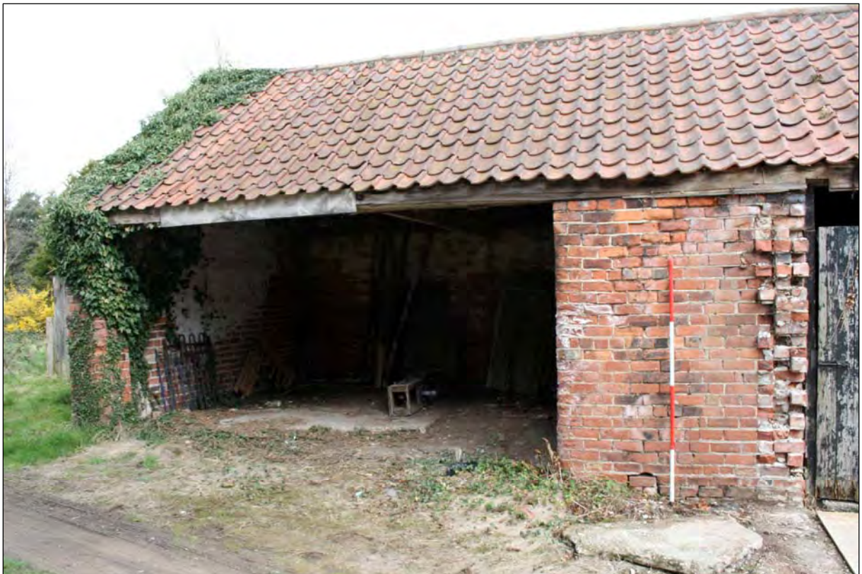
Plate 60. B6 exterior NW looking north (image no. 458).
