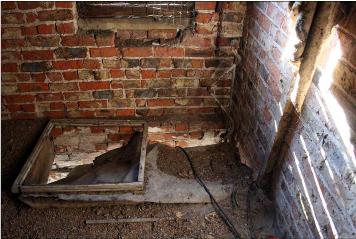
Plate 13. B1 interior first floor. Floor opening looking SE (image no. 035).
