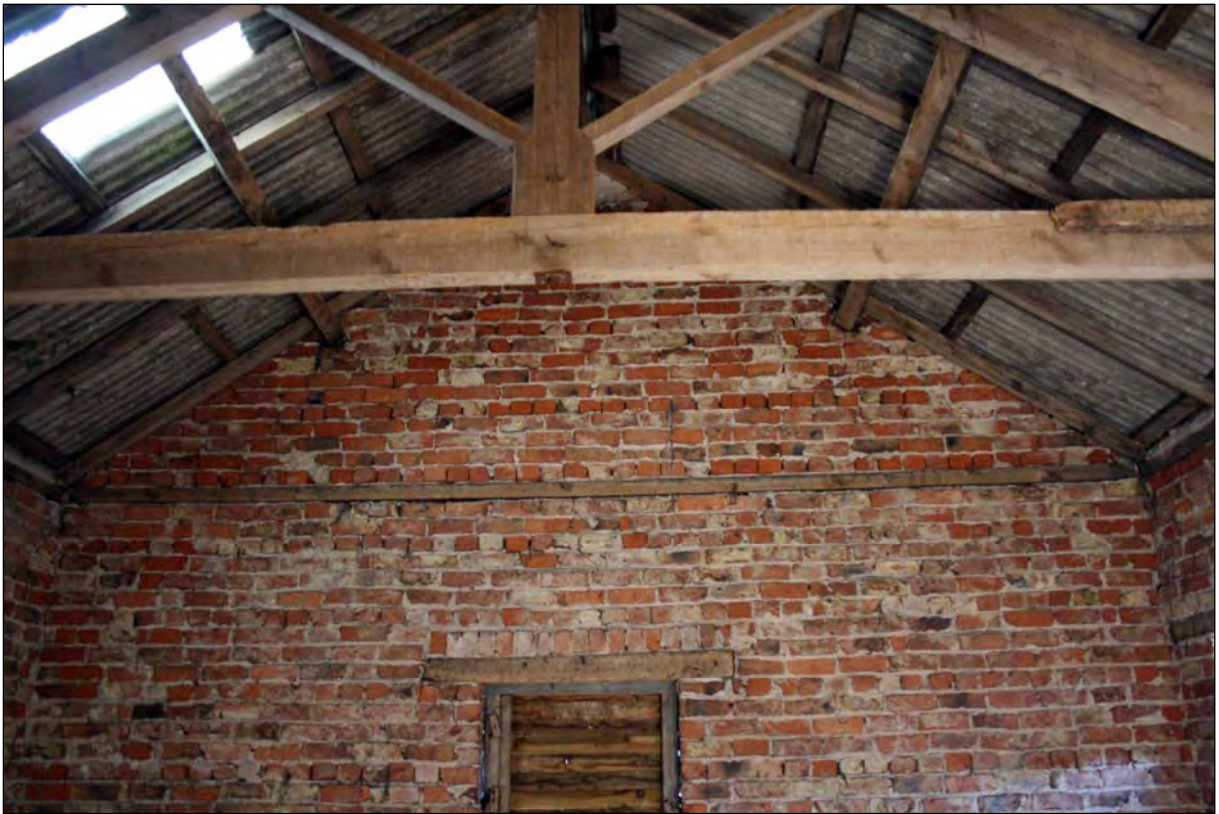
Plate 7. B1 interior looking NE (image no. 008).
