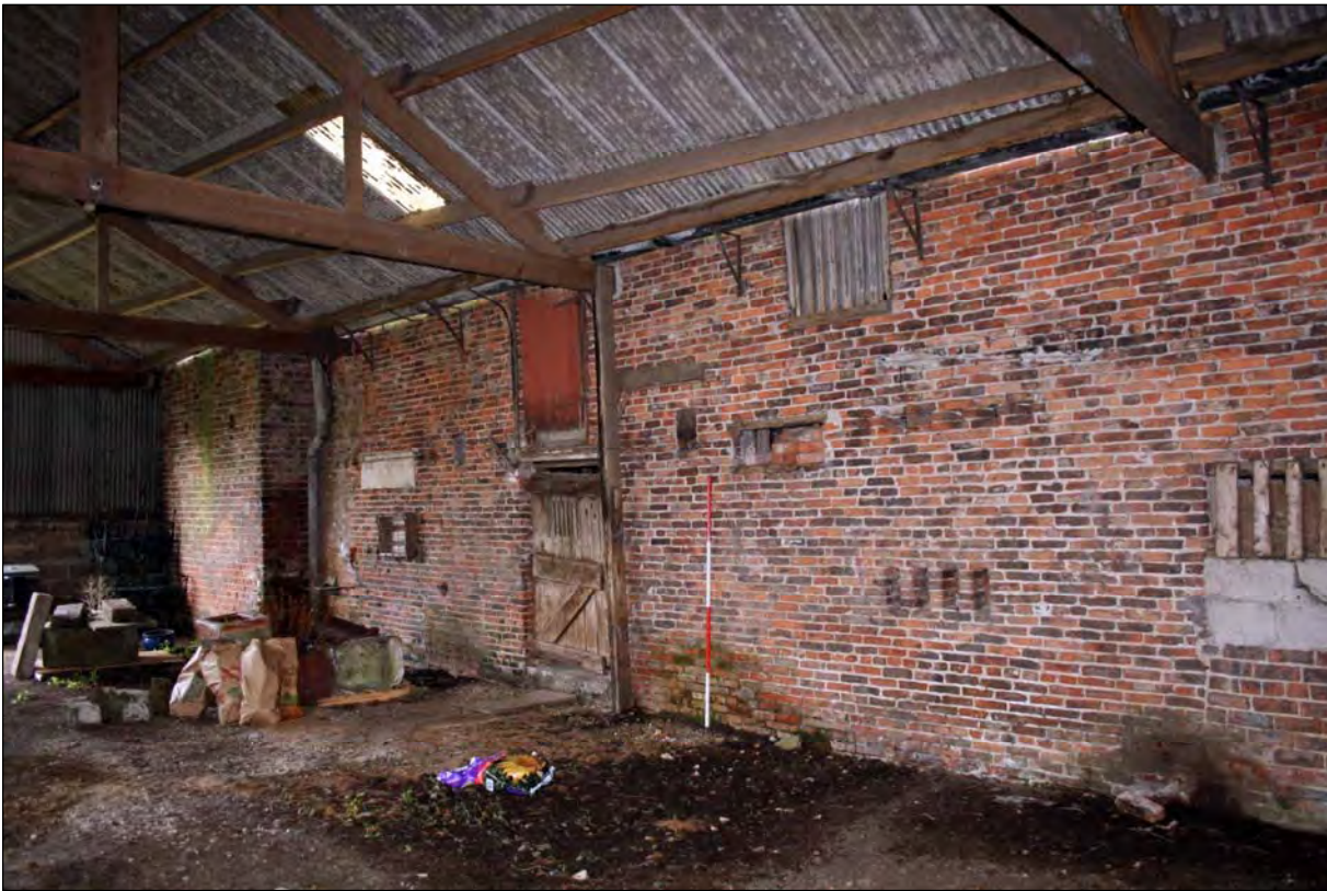
Plate 37. B3 and B4 exterior looking NE (image no. 332).
