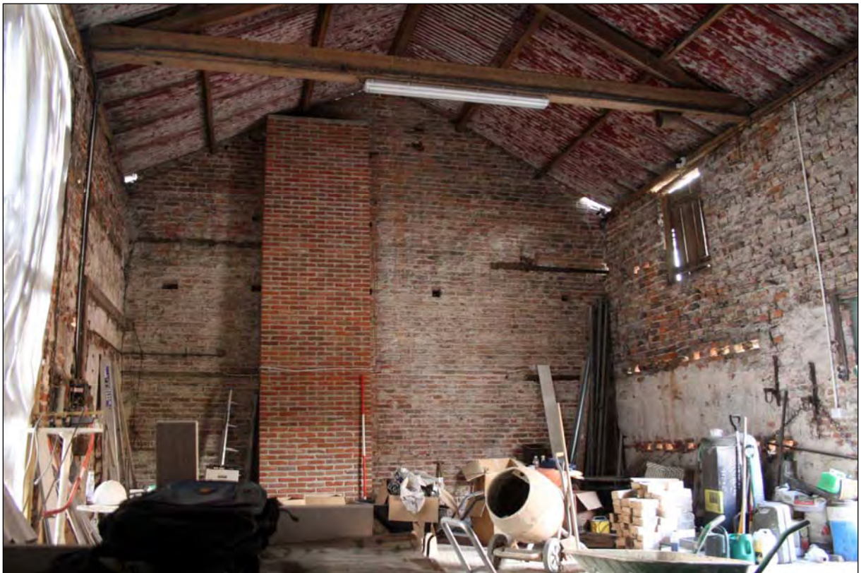
Plate 56. B5 interior looking SW (image no. 296).
