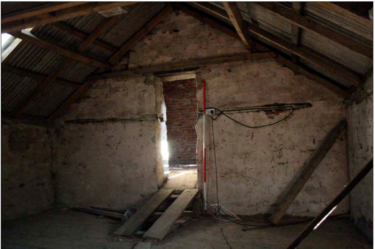
Plate 12. B1 interior doorway looking SE (image no. 058).
