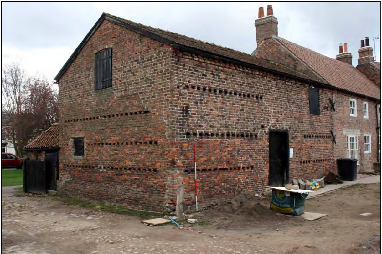
Plate 51. B5 exterior looking south (image no. 406).
