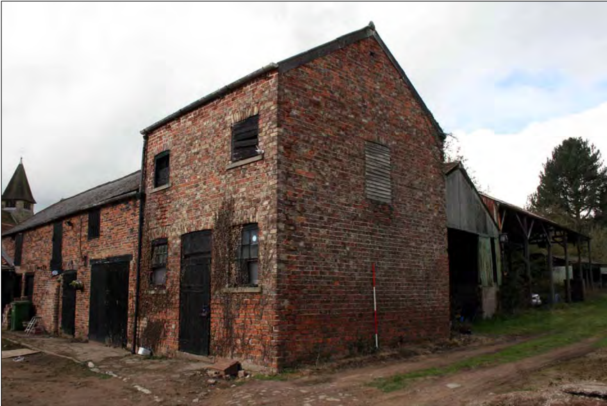
Plate 1. B1 exterior looking west (image no. 298).
