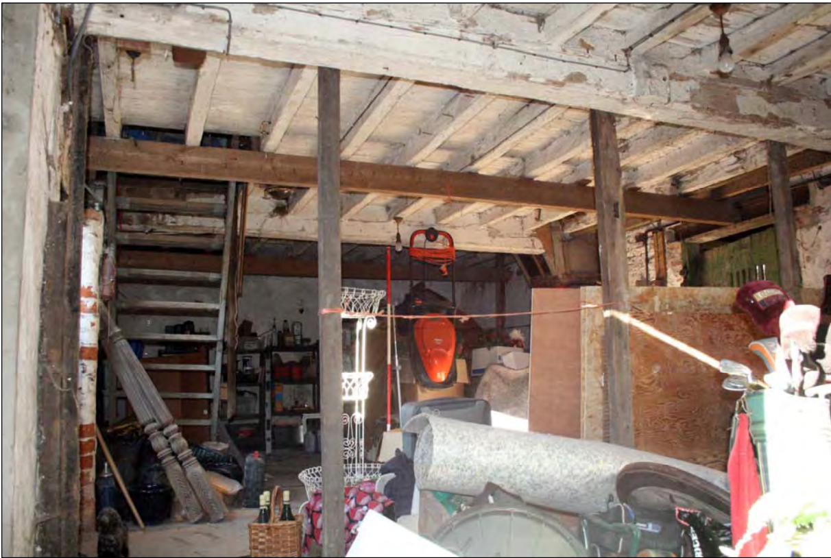
Plate 45. B3 interior ground floor looking SW (image no. 091).
