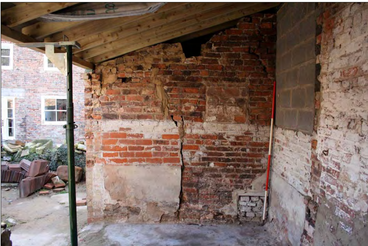
Plate 26. B2 interior NW looking southeast (image no. 240).
