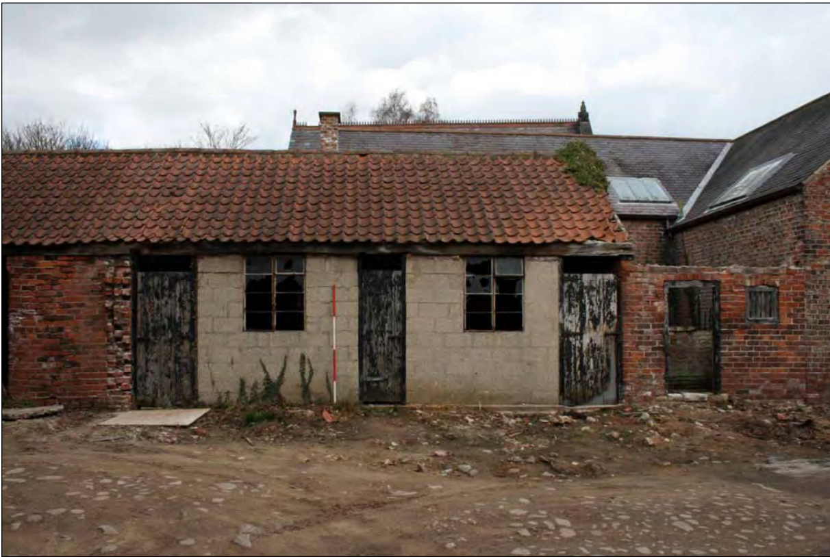
Plate 61. B6 exterior SE looking northeast (image no. 459).
