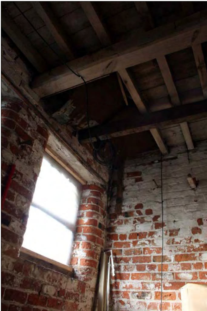
Plate 17. B1 interior ground floor opening in ceiling looking south (image no. 157).
