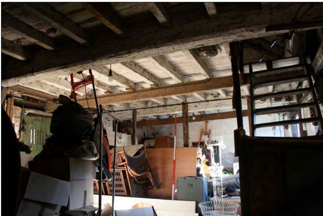
Plate 44. B3 interior ground floor looking north (image no. 081).
