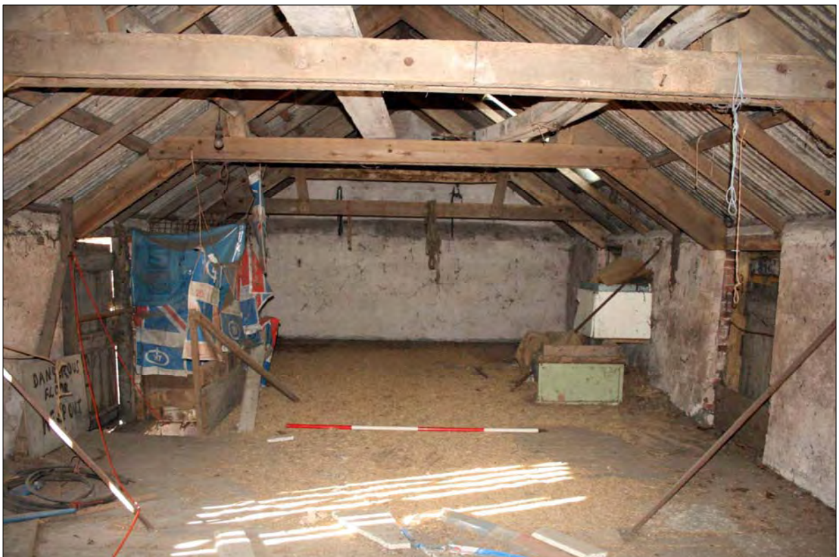
Plate 40. B3 interior first floor looking SW (image no. 044).
