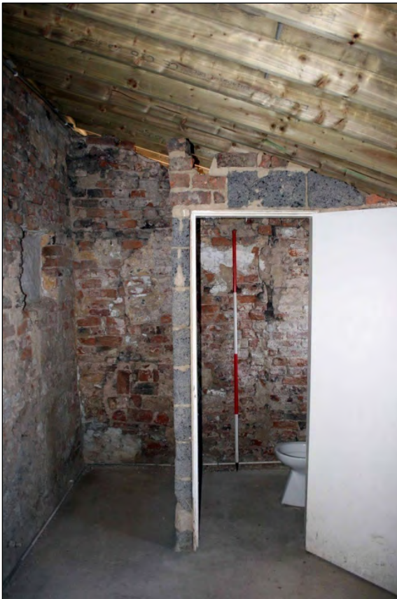
Plate 31. B2 interior SE bricked up doorway/window looking NW (image no. 223).
