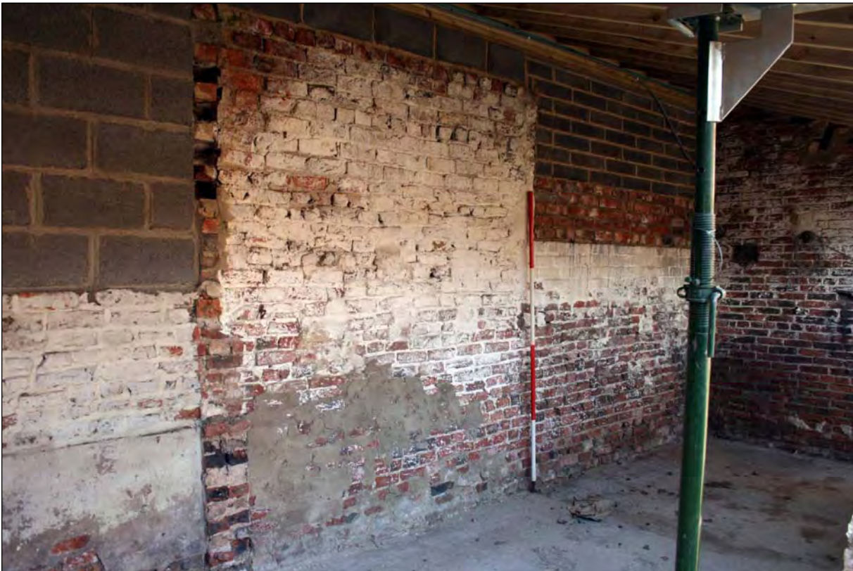
Plate 25. B2 interior NW looking west (image no. 253).
