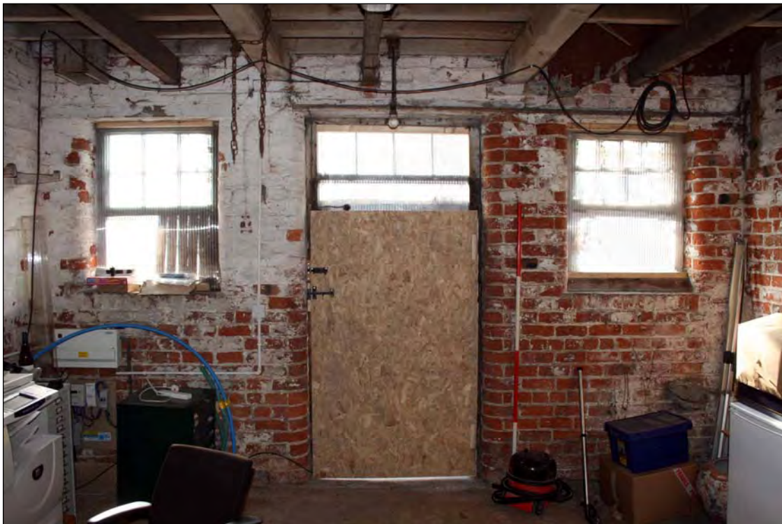
Plate 18. B1 interior ground floor looking NW (image no. 153).
