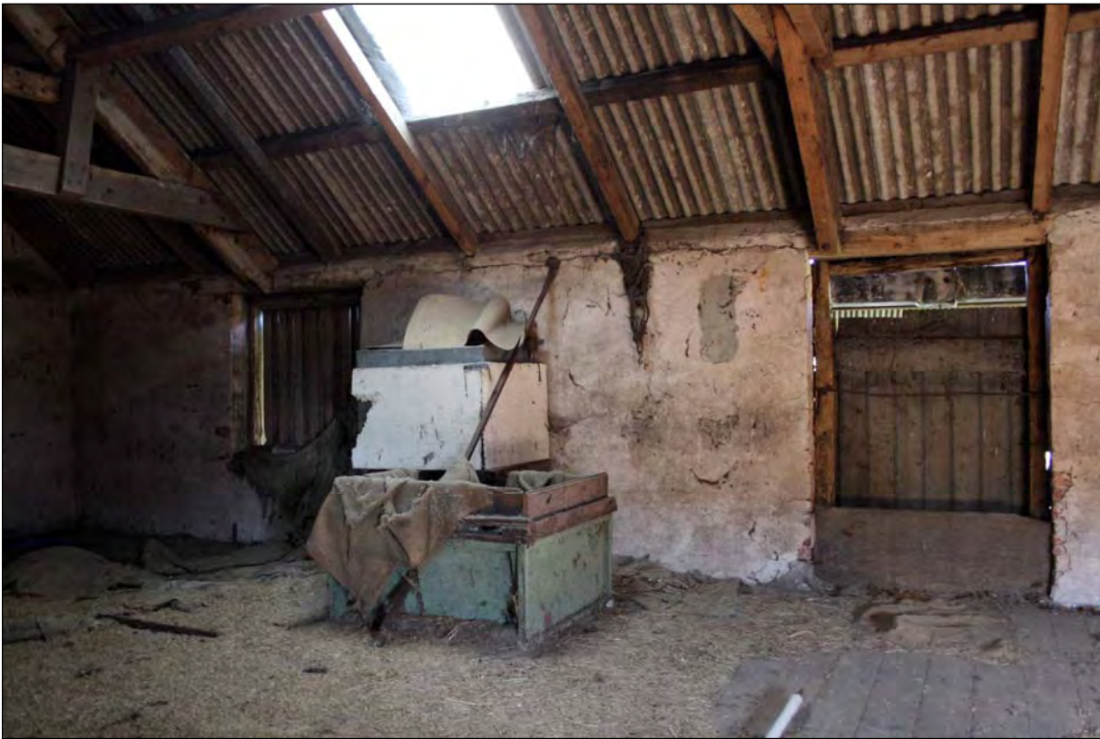
Plate 41. B3 interior first floor looking west (image no. 067).
