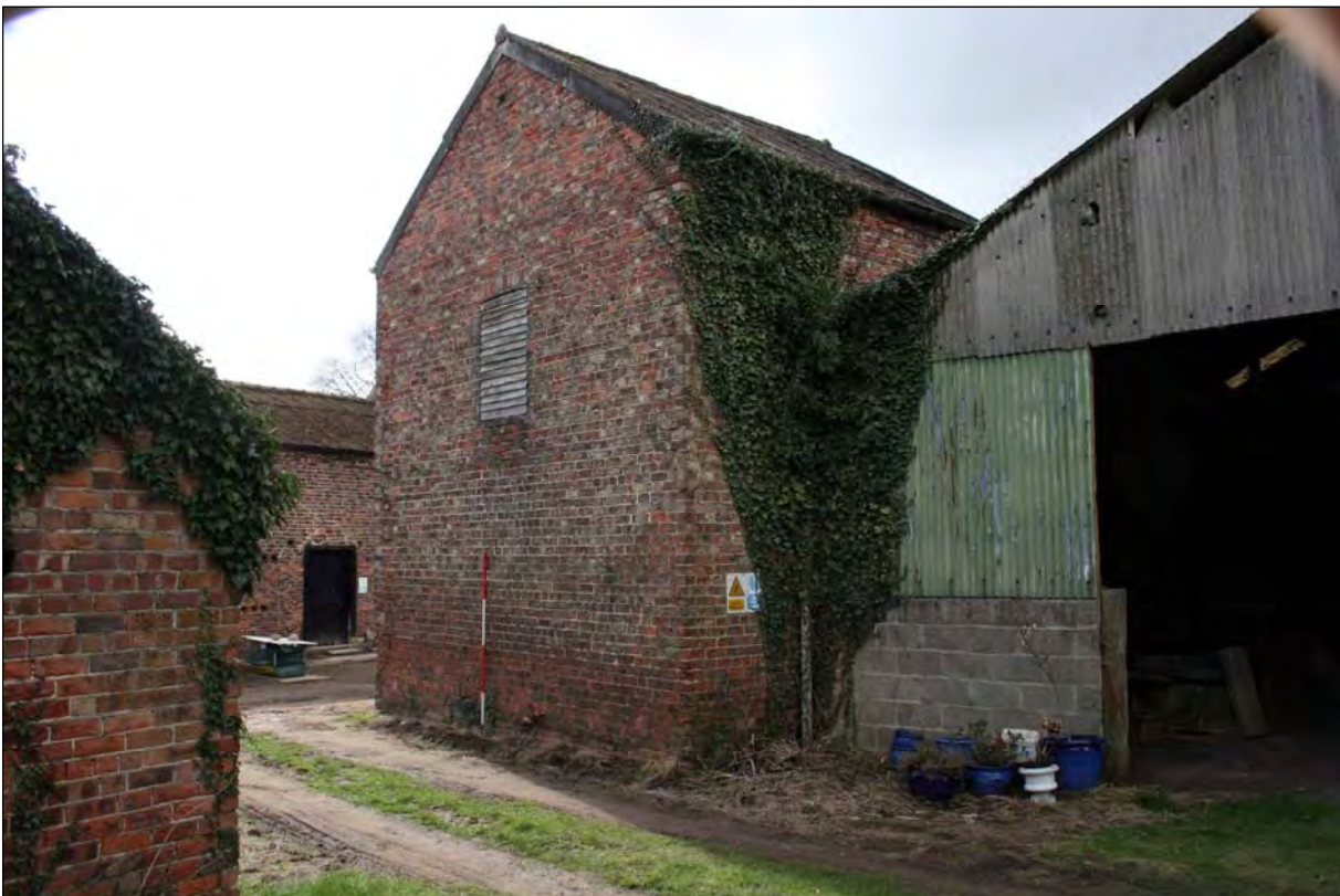
Plate 2. B1 exterior looking south (image no. 300).
