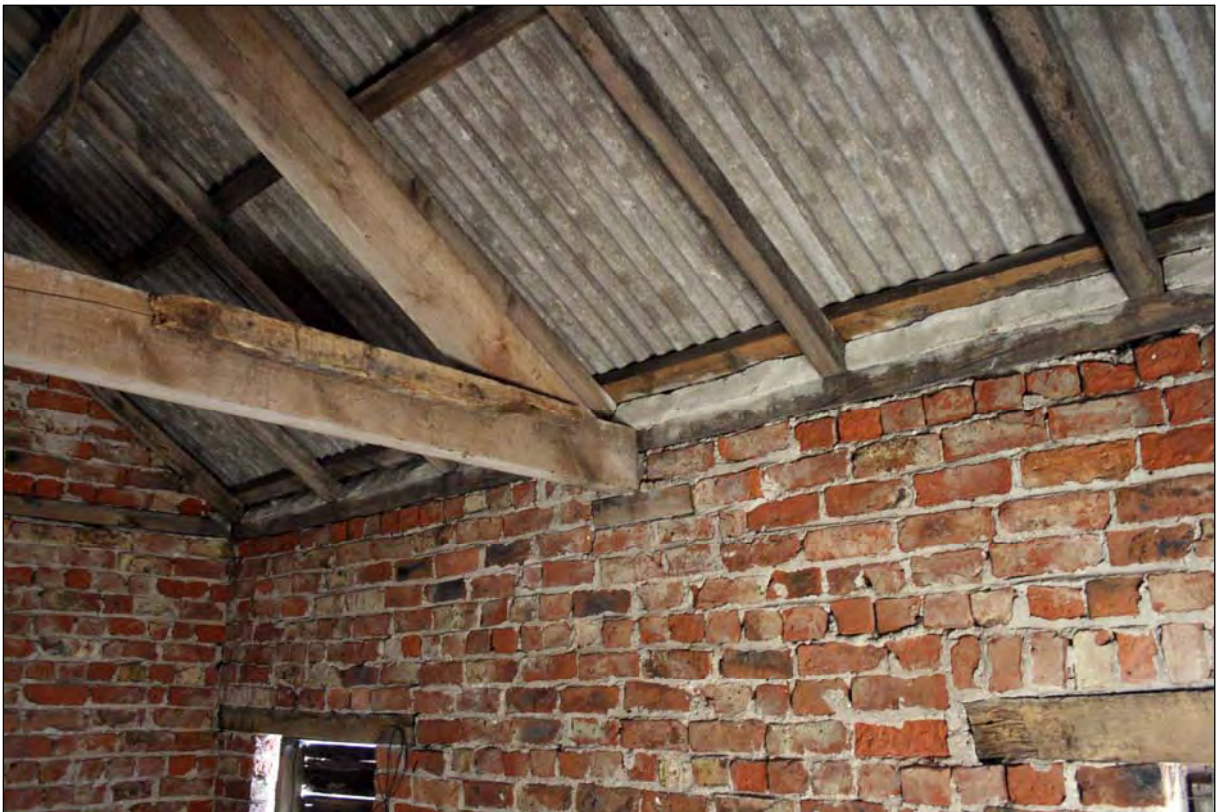
Plate 8. B1 interior looking east (image no. 023).
