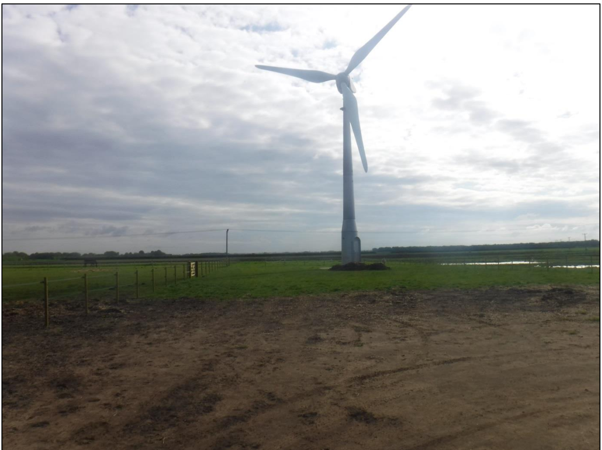
Plate 6. View of wind turbine located in the central-eastern part of the site, looking east.
