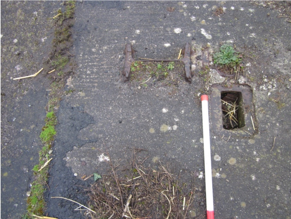
Fig 15 Girder sections that may have formed wall supports
