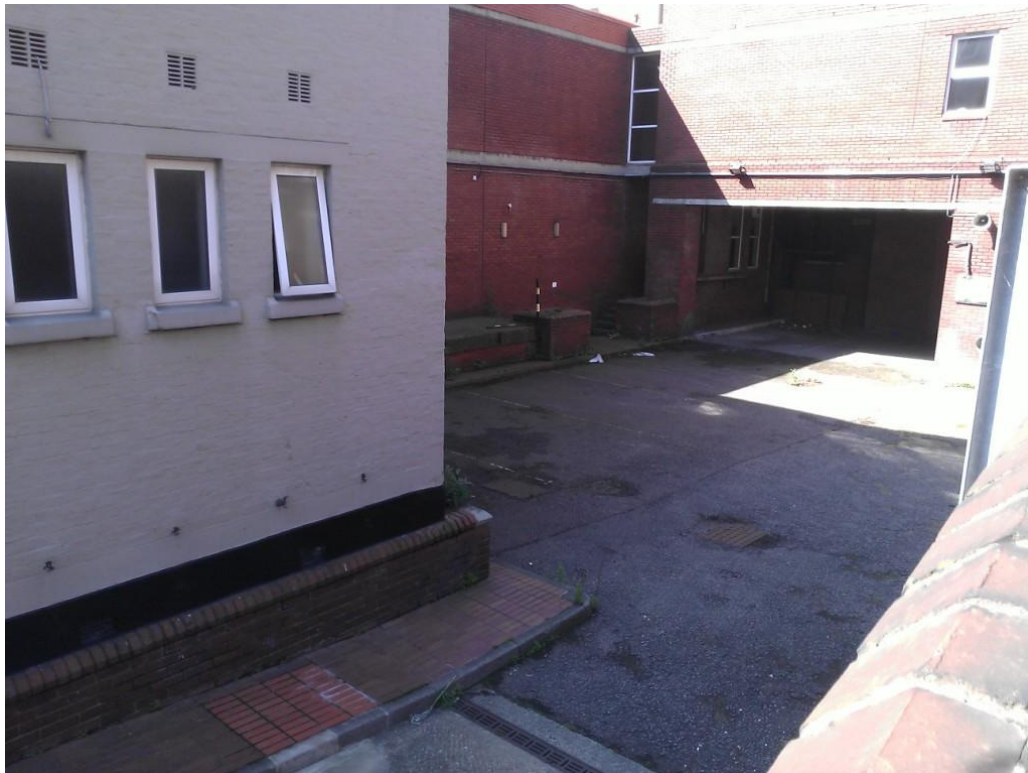
Figure 4 Courtyard and car parking area
