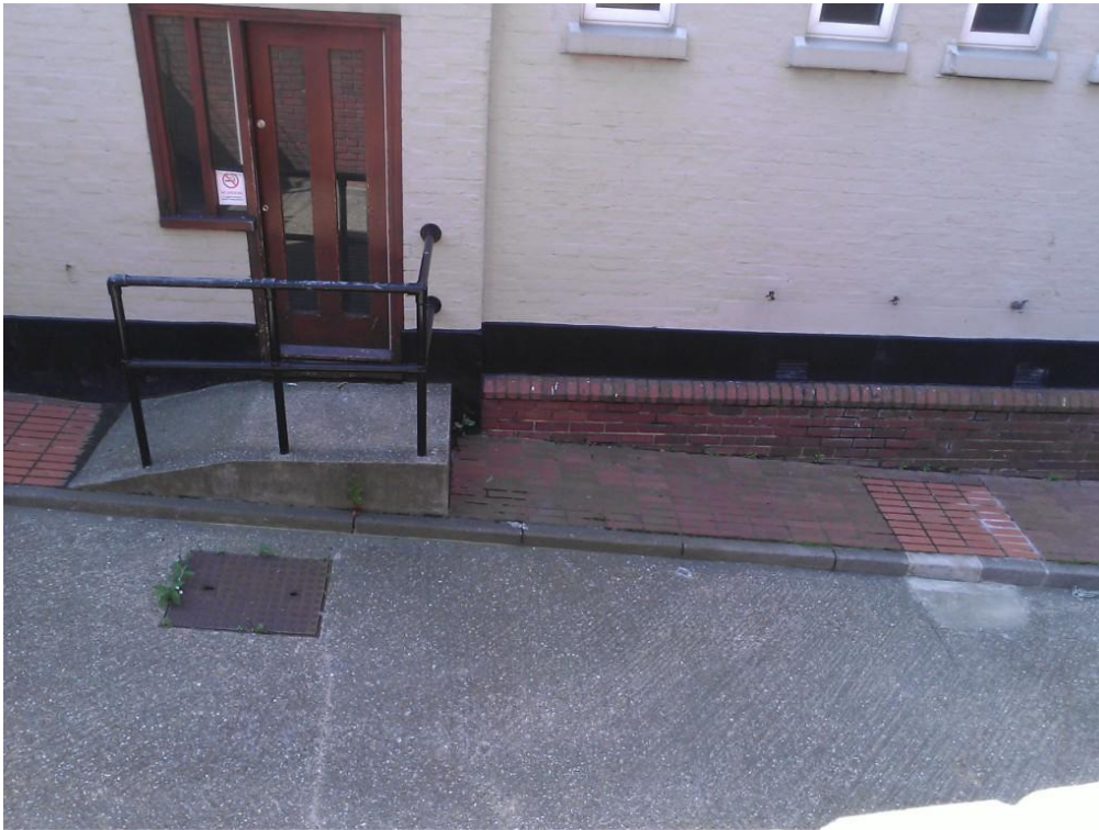
Figure 3 Concrete entrance roadway looking south
