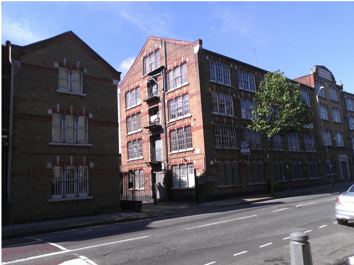
Figure 5 Neckinger Mills looking south from Abbey Street
