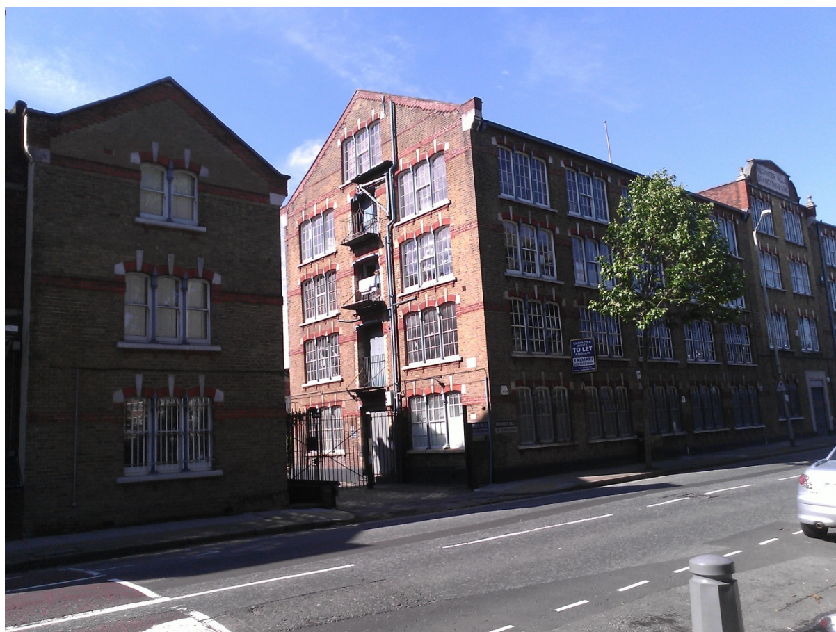
Figure 3 Neckinger Mills looking south from Abbey Street
