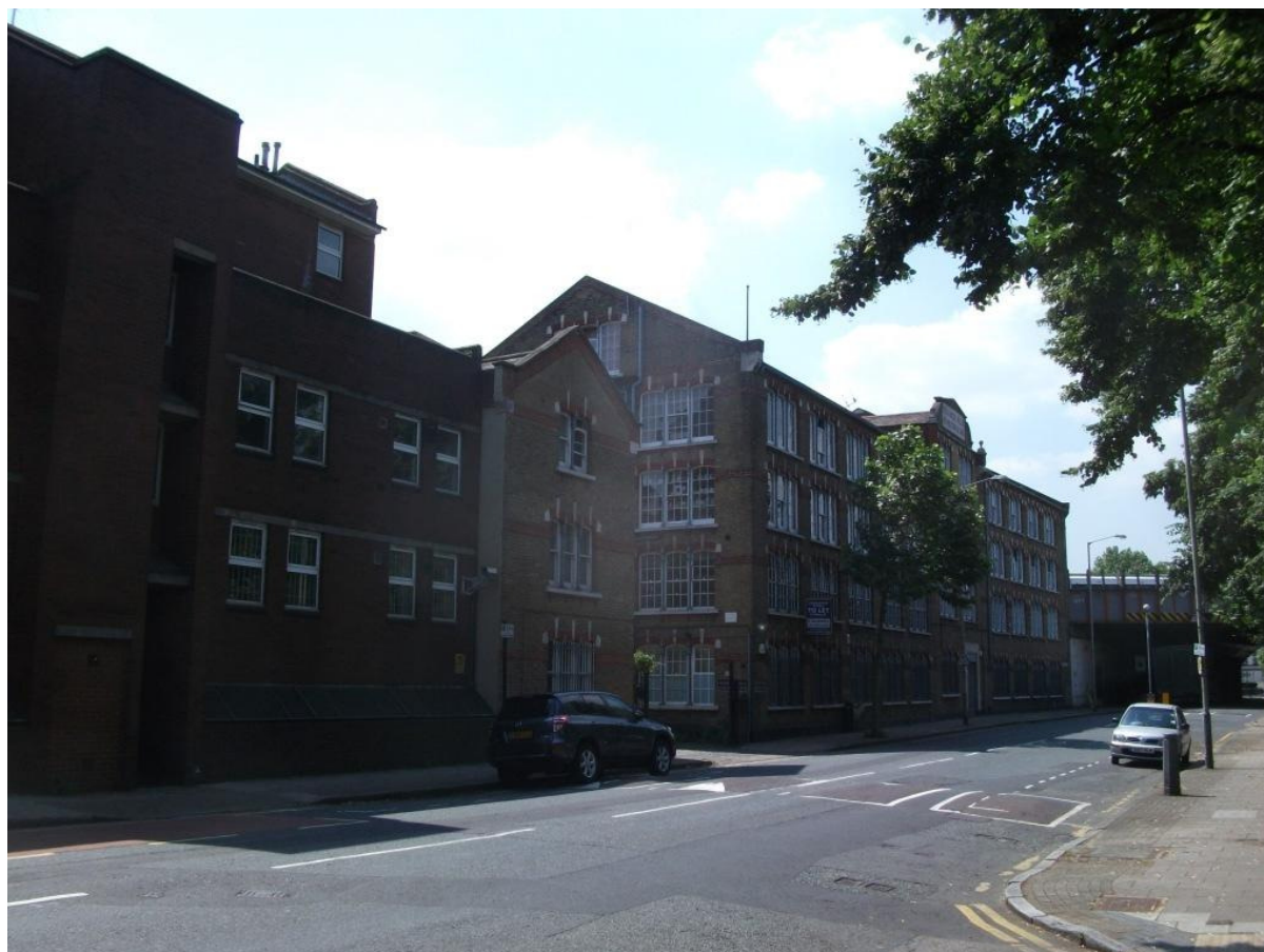
Figure 5 View of Neckinger Mills from Abbey Street with Old Drill Hall site adjoining
