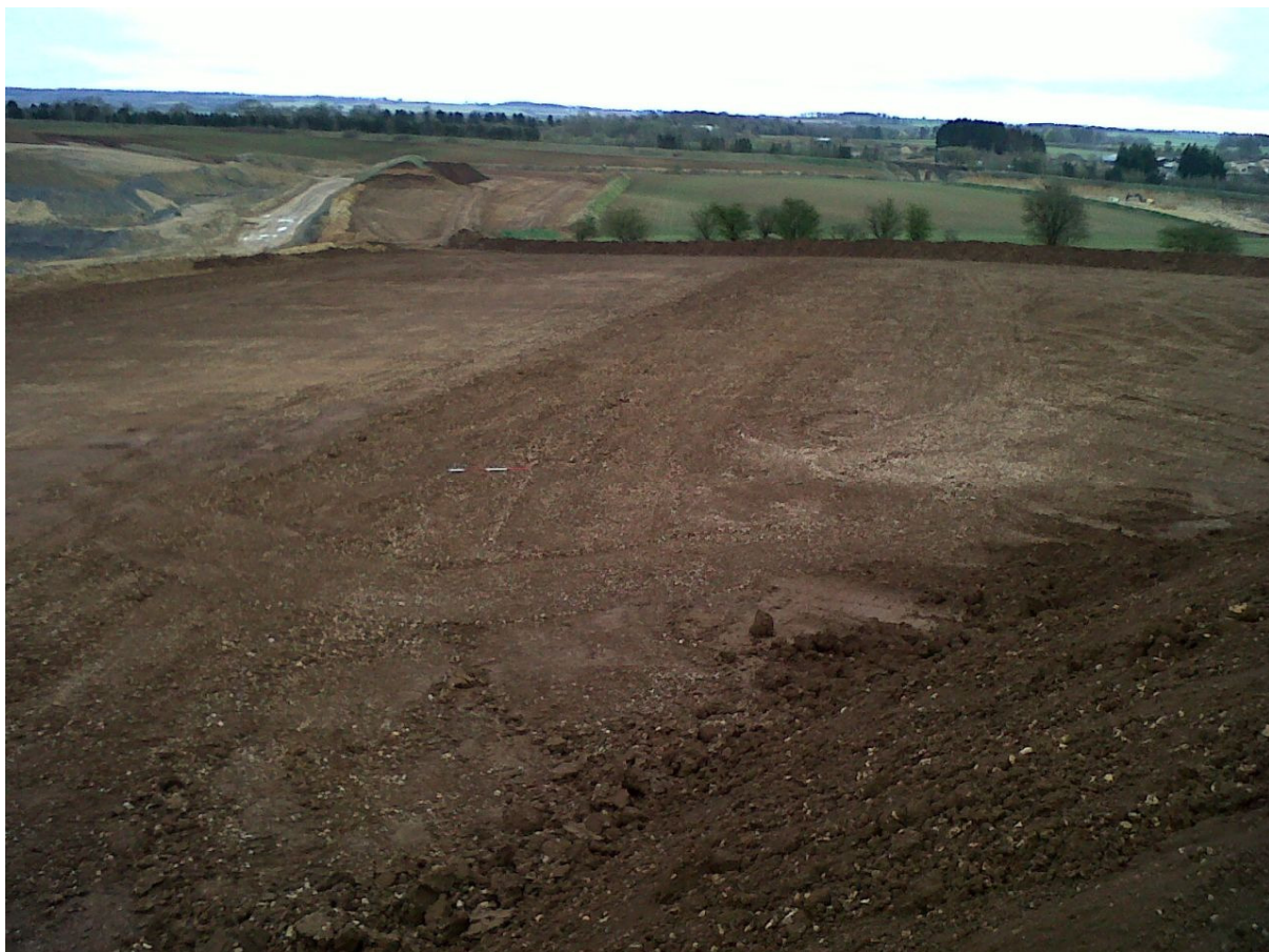
Figure 9 View of stripped area April 2012 looking northeast
