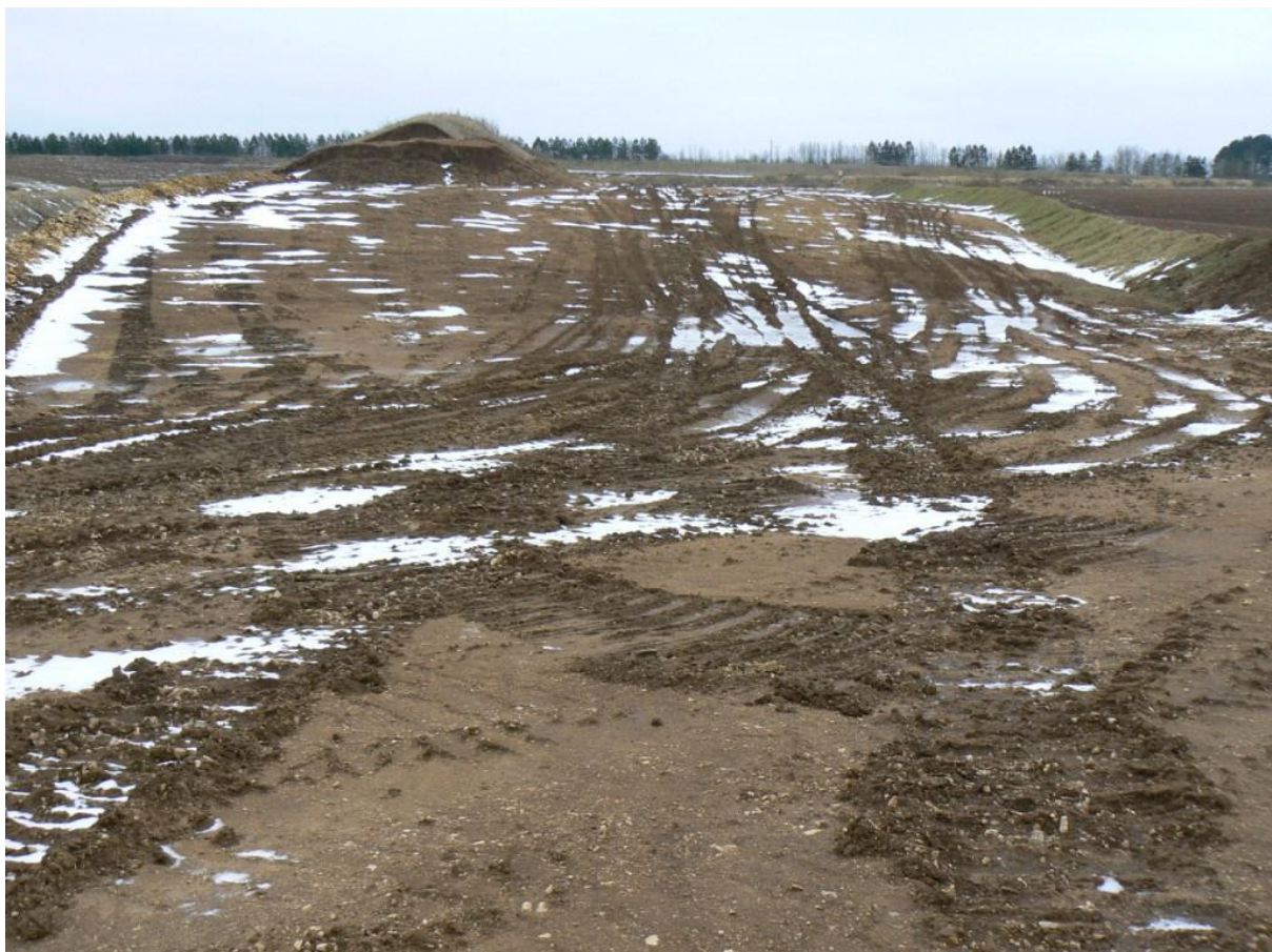
Figure 7 Photograph of February 2012 stripped area looking northeast
