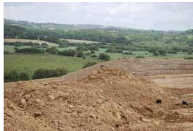
Figure 4: Views of site work in progress
