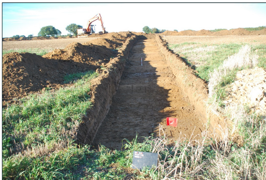
Figure 5-14 Trench 11 looking NNE
