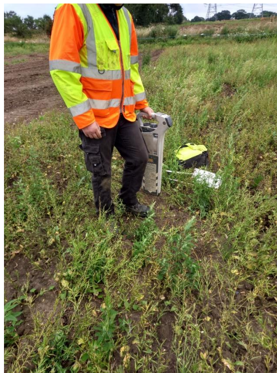
Plate 2. General Working Shot, SRS44
