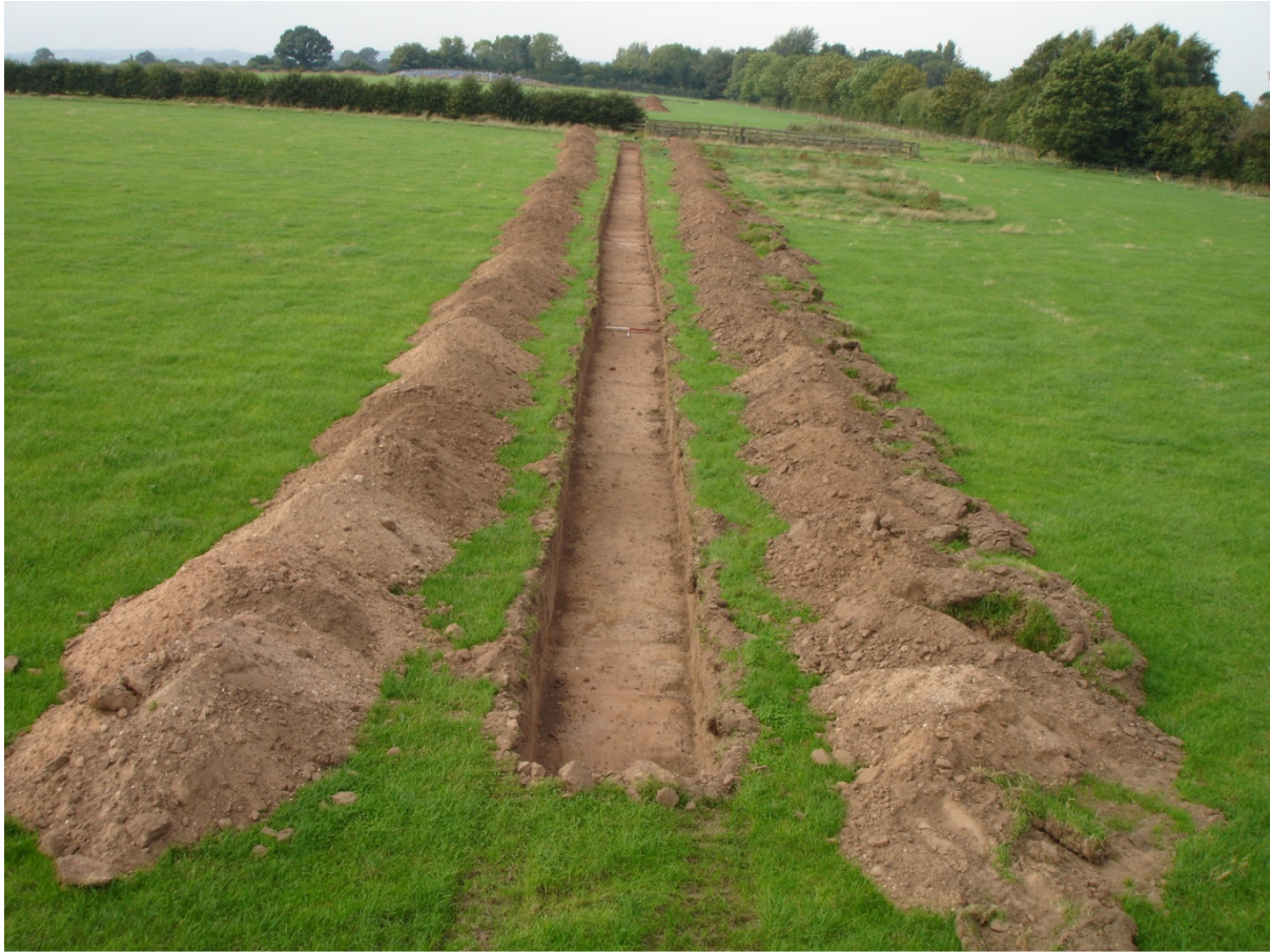
Plate 1. Trench 1 Overview. View: SE
