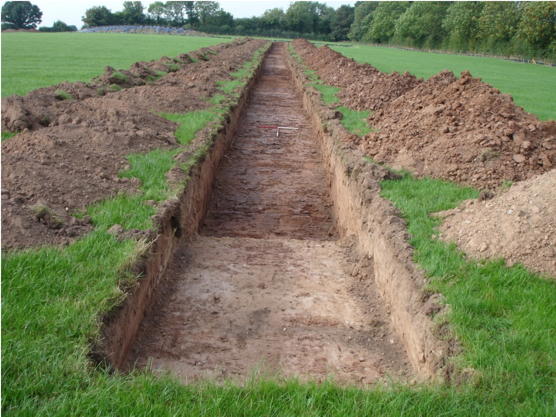
Plate 14. Trench 8 Overview. View: WSW
