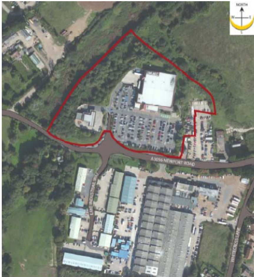
Figure 2 Aerial Photograph of the Site 4
