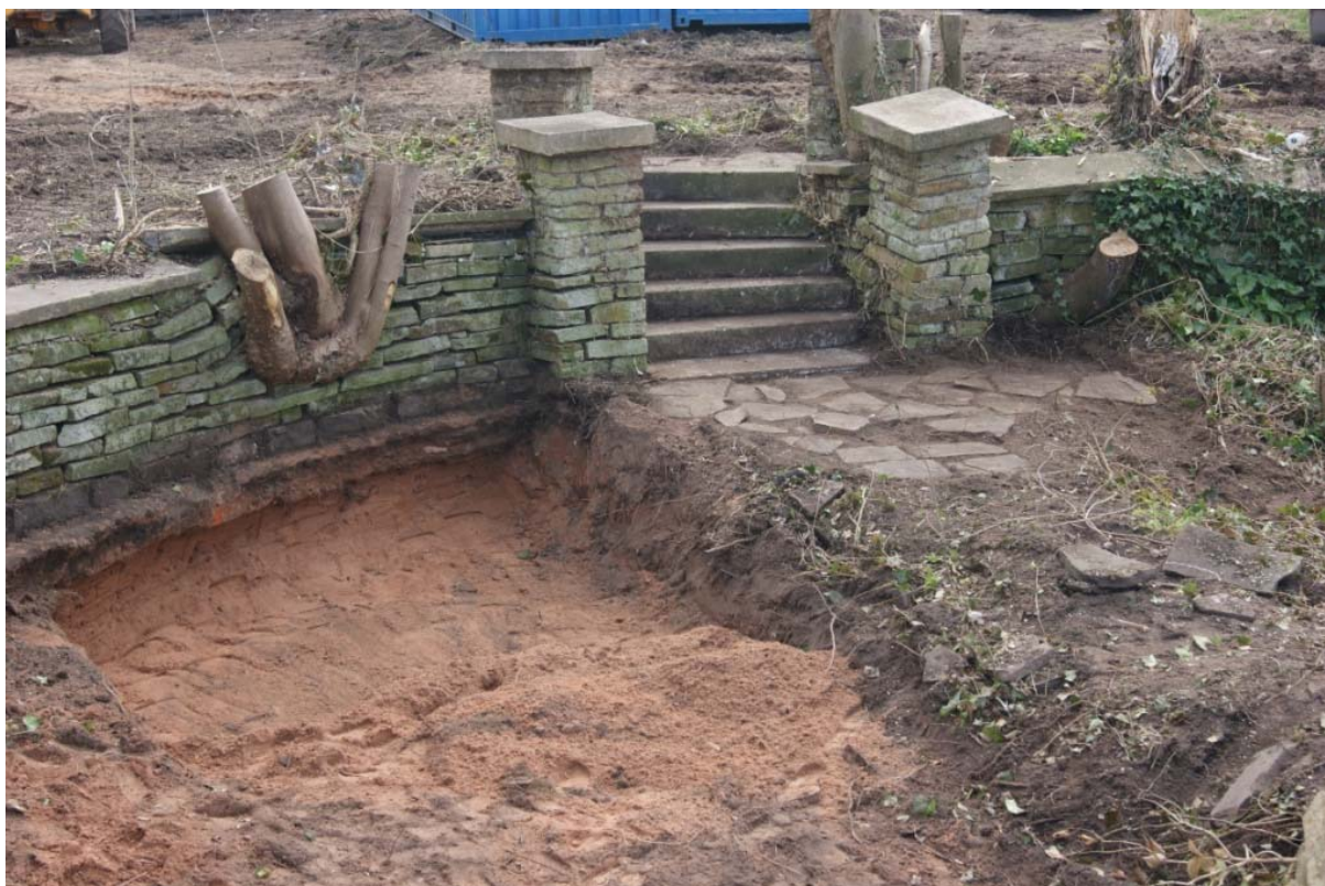
Plate 3: Sunken Garden wall, foundation, raised path and steps looking southwest
