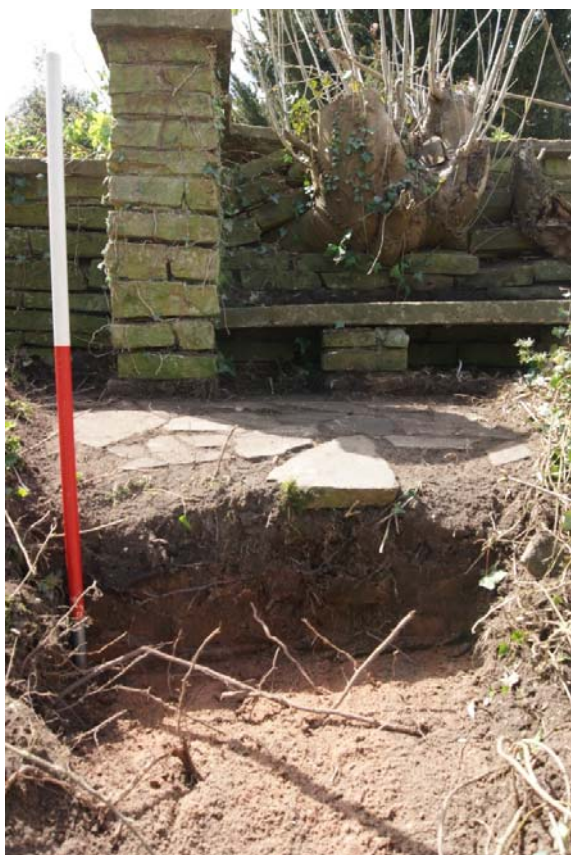
Plate 6: foundations for bench
