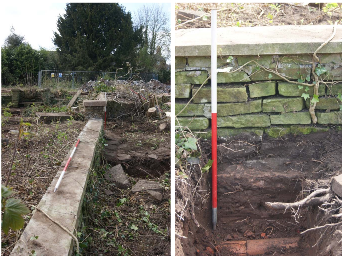
Plate 7: Retaining (dividing) wall looking southwest, and foundations looking east
