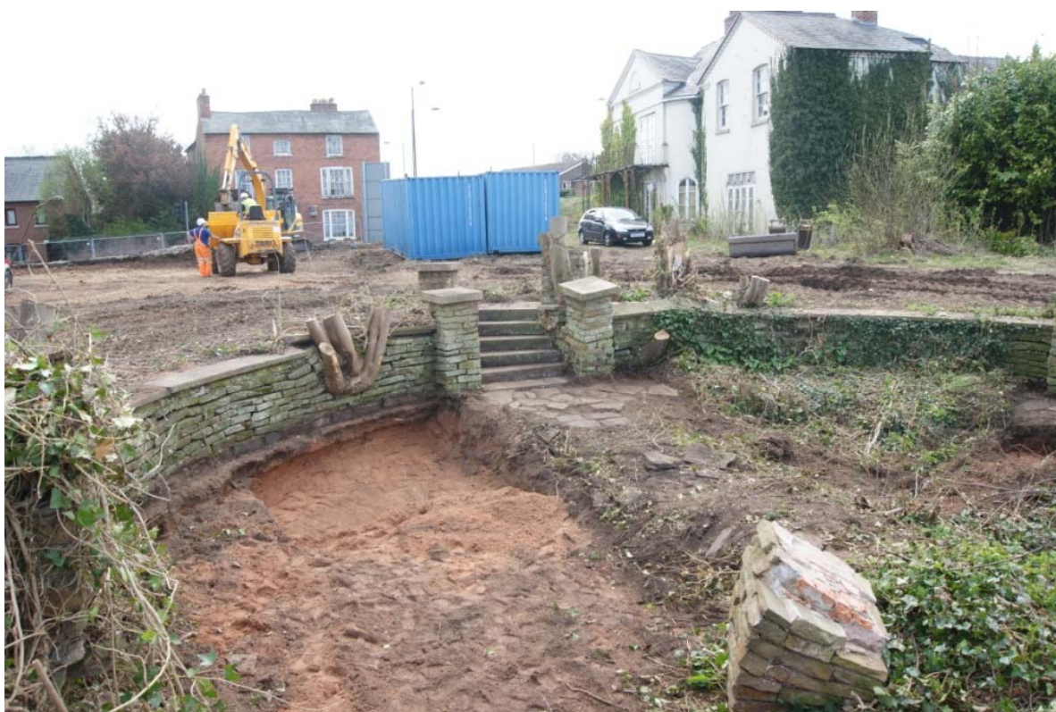
Plate 2: Sunken Garden after removal of vegetation and archaeological investigation
