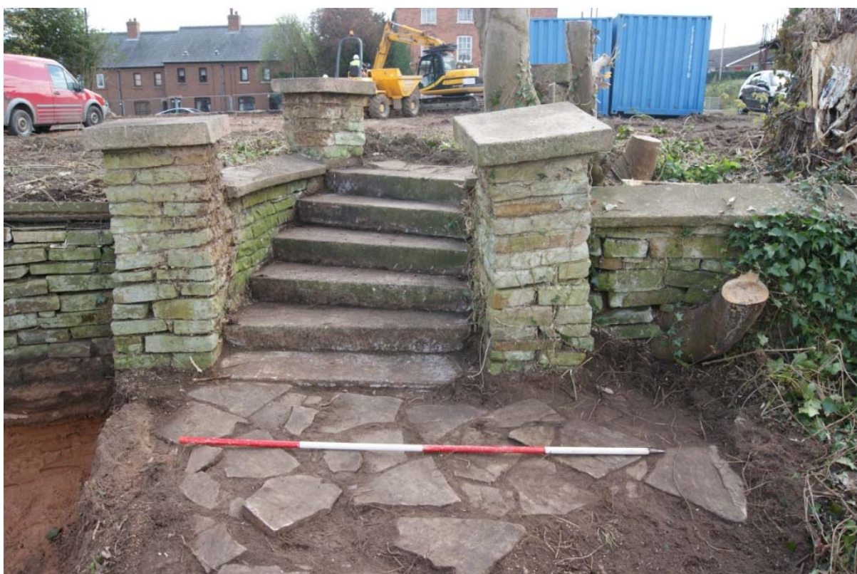
Plate 4: Detail of steps and path construction
