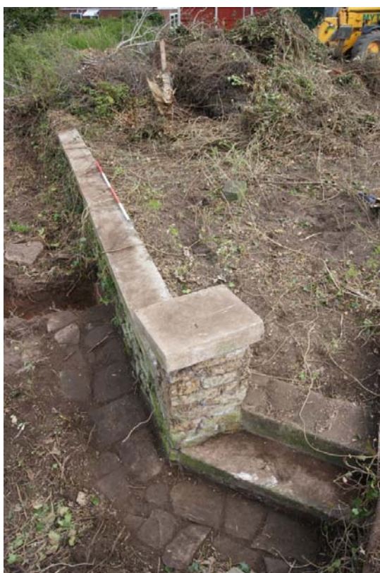
Plate 8: steps down from retaining wall on to path
