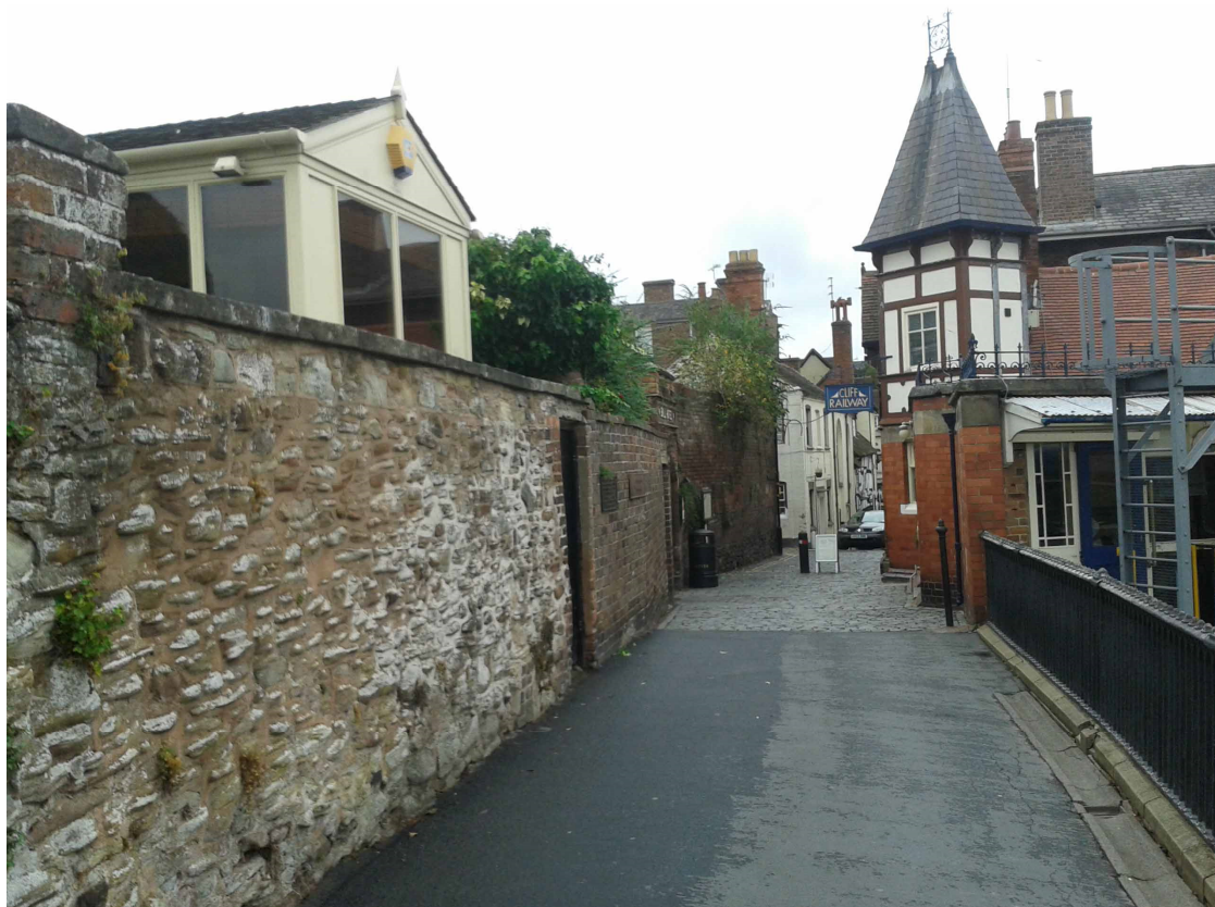
Figure 10 Looking north along Castle Terrace showing original stone coursed wall, with brick rebuilds at the northern end forming the boundary of the application site
