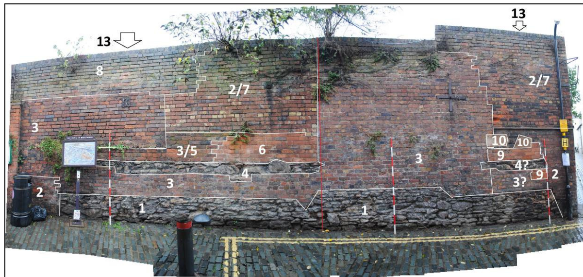
Figure 1 The Castle Terrace wall section, looking west
