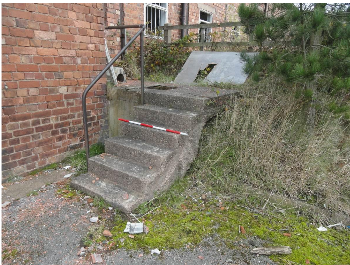
Plate 15. Concrete steps leading the southern elevation and rear of Building 9.6
