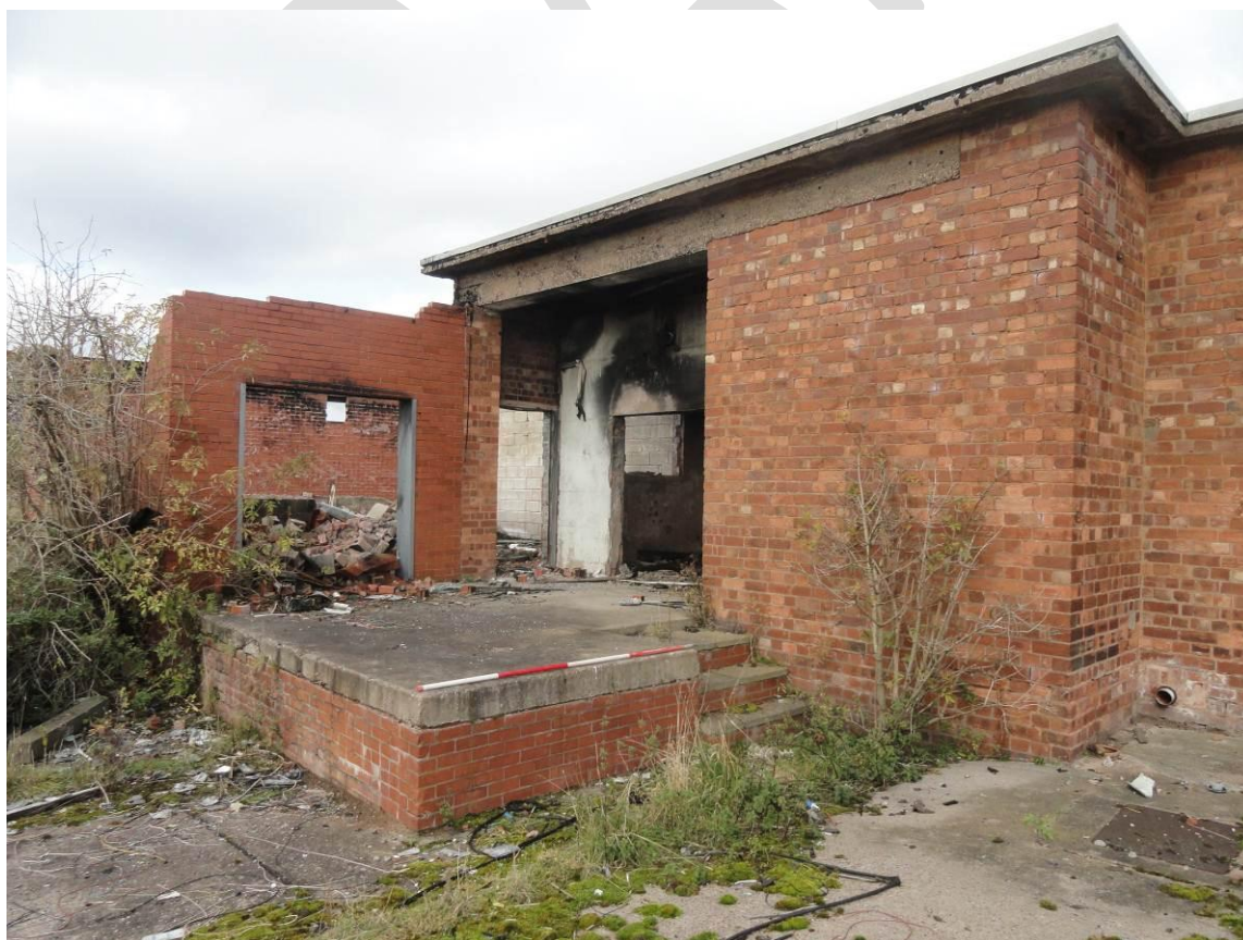
Plate 10. Loading platform and main entrance into Building 9.5, looking north-west
