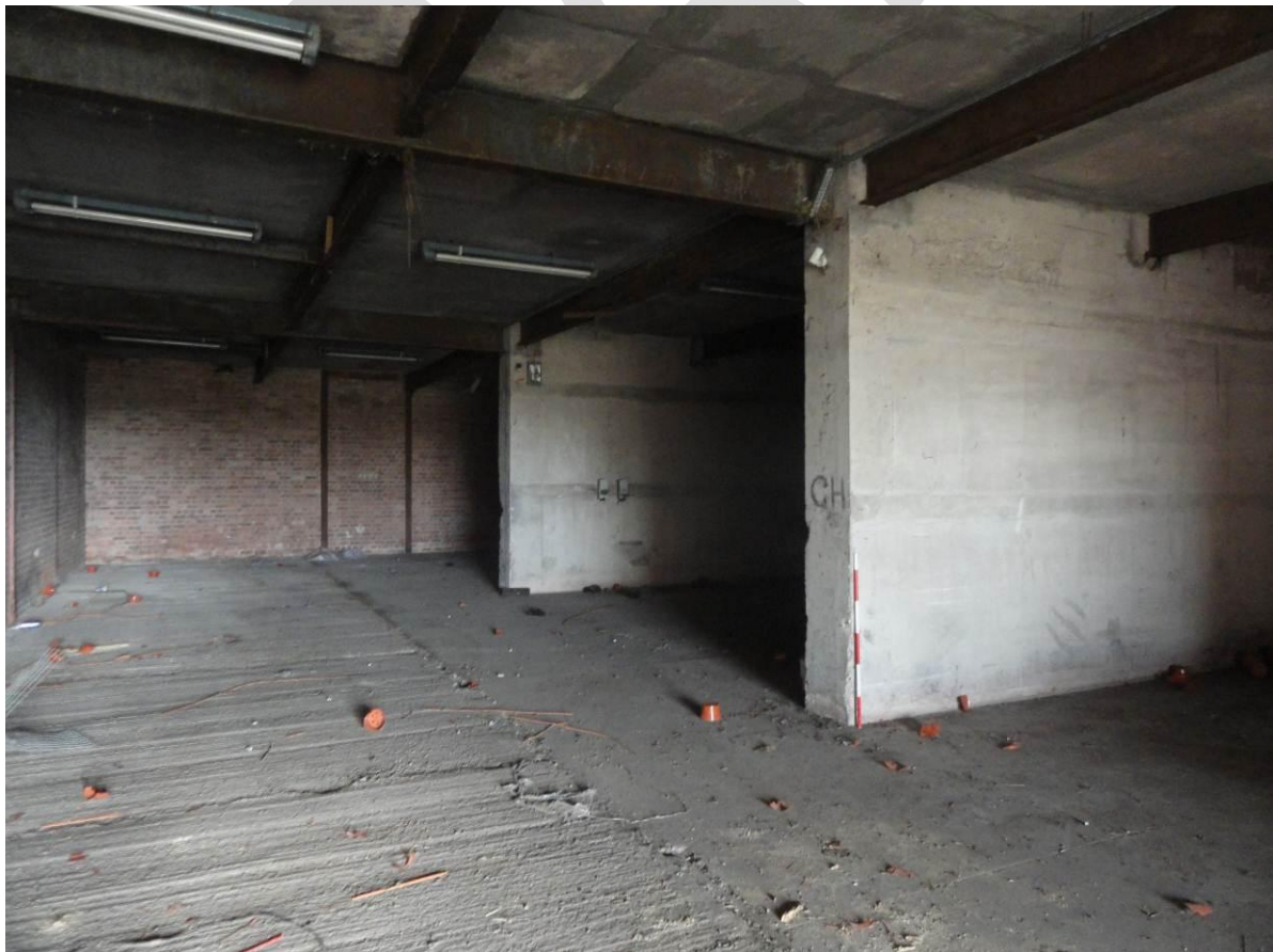
Plate 6. Internal partitions within Building 9.3, looking north
