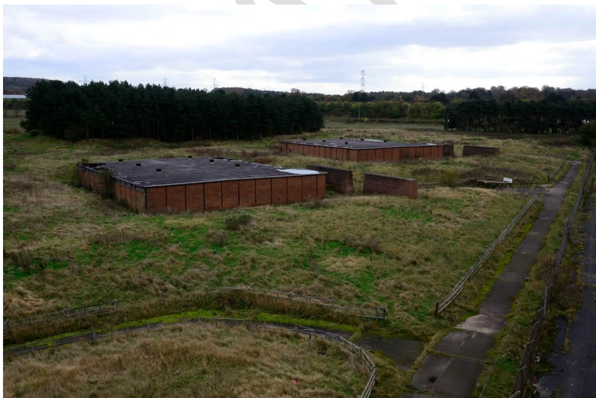
Plate 4. Building Nos. 9.8 and 9.9 with their respective blast walls, looking south
