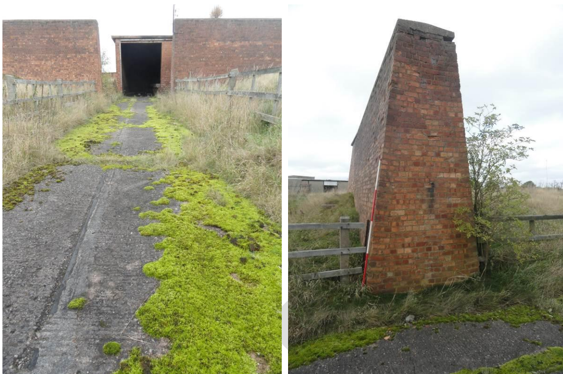
Plate 19. Railway line leading to Building 9.8, via a blast wall set
