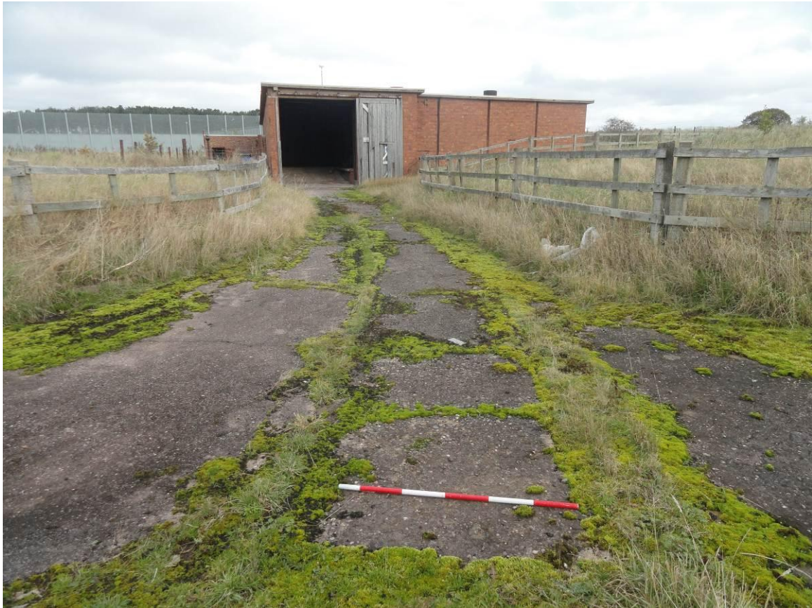
Plate 7. Standard gauge railway line leading to Building 9.3, looking north
