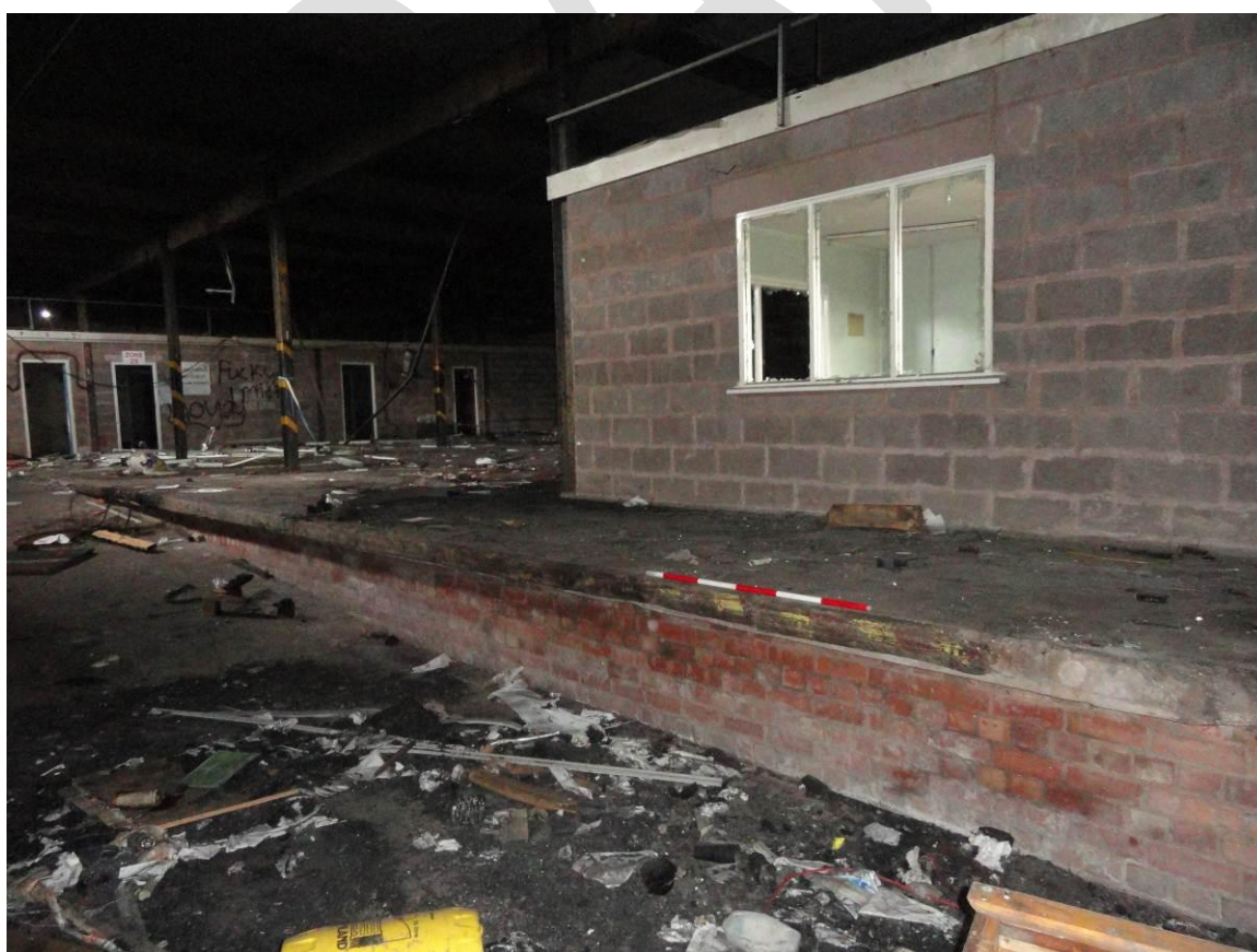
Plate 16. Internal view of loading platform of Building 9.6, looking north-east
