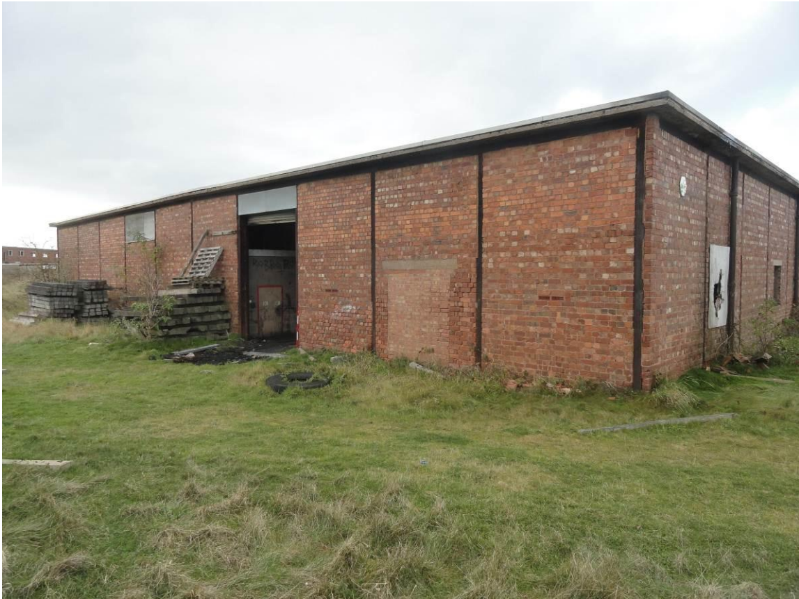
Plate 17. Rear elevation of Building 9.6, looking south-west
