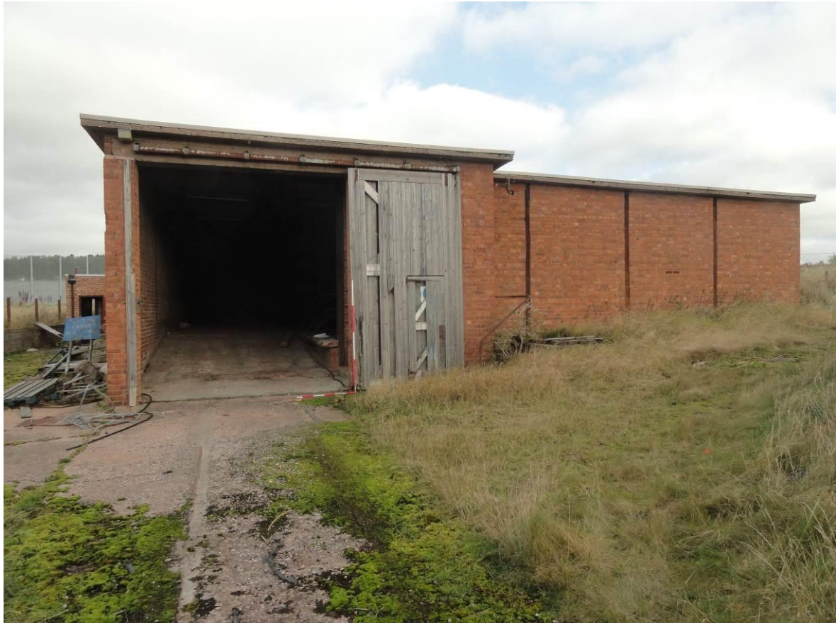
Plate 5. Building 9.3 showing sliding door entrance leading to loading platform, looking north
