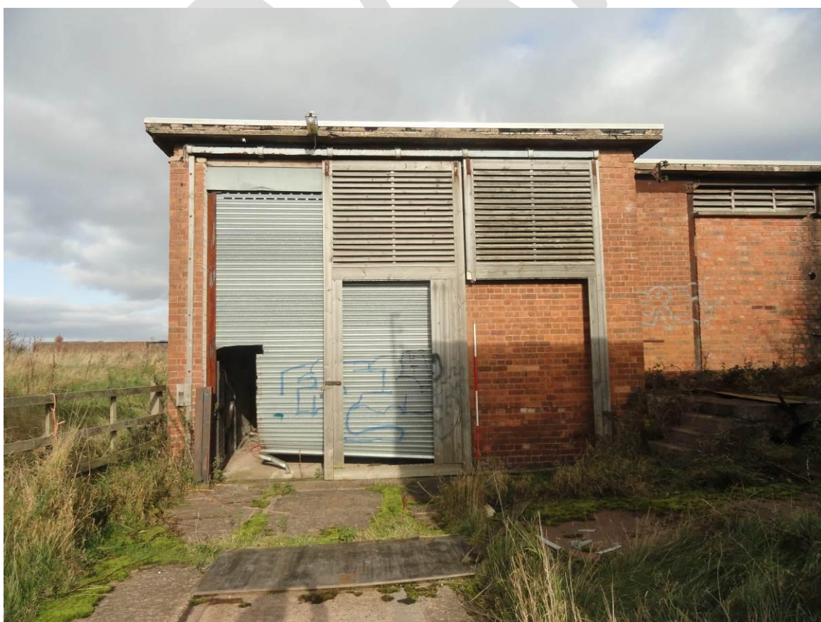
Plate 28. Southern entrance to Building 9.9 with original door sections, looking north
