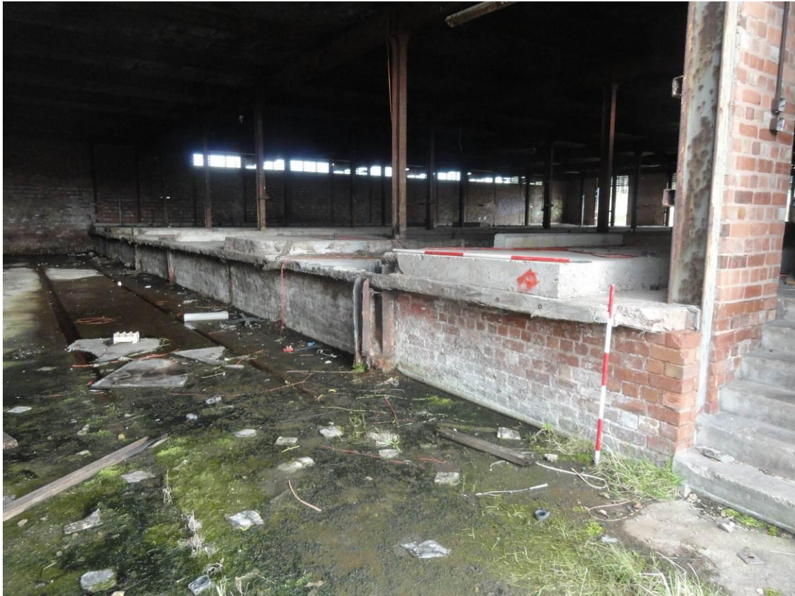
Plate 24. Loading railway platform within Building 9.8, looking north-east
