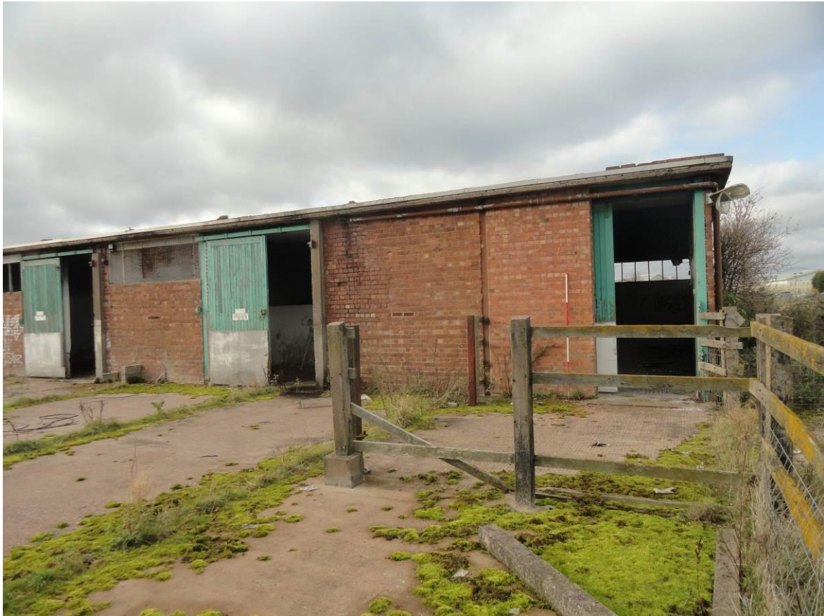
Plate 11. Rear elevation of Building 9.5, looking west
