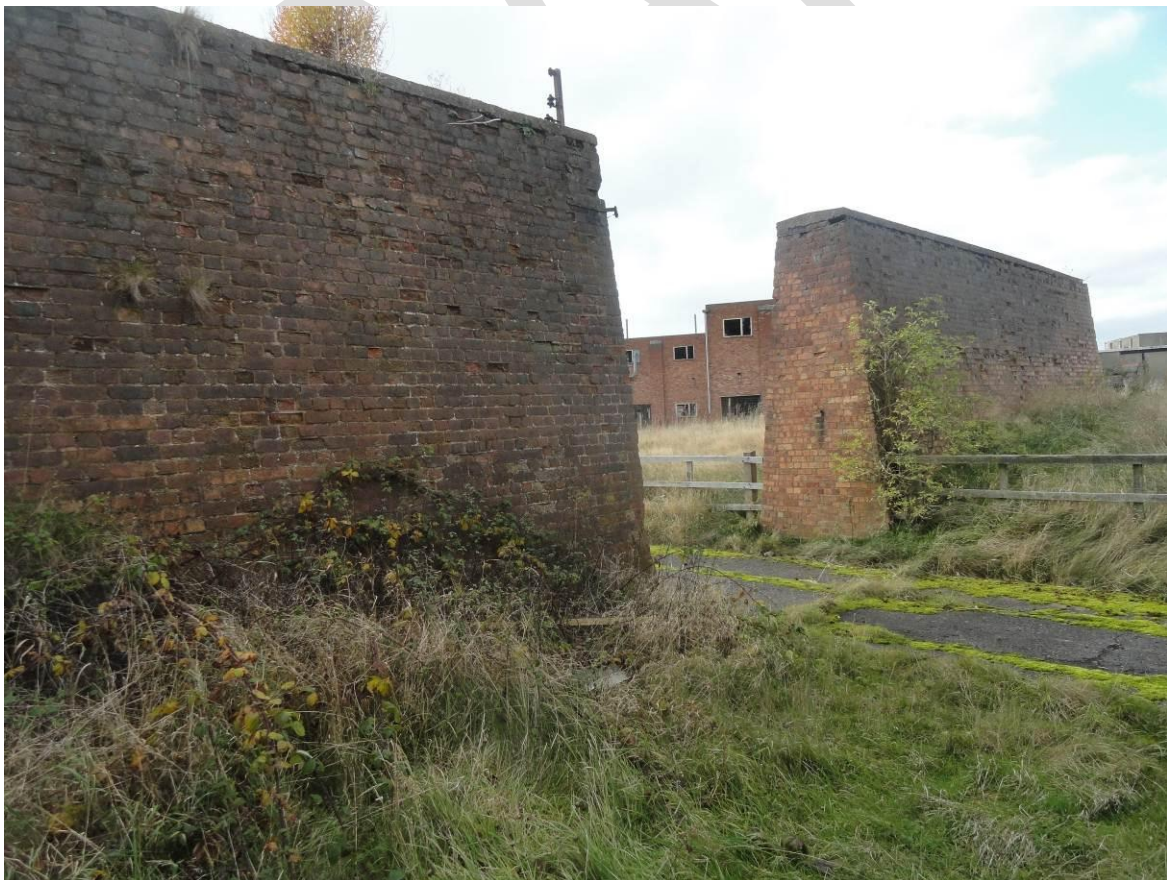
Plate 25. Blast wall set belong to Building 9.8; internal view, looking south-west
