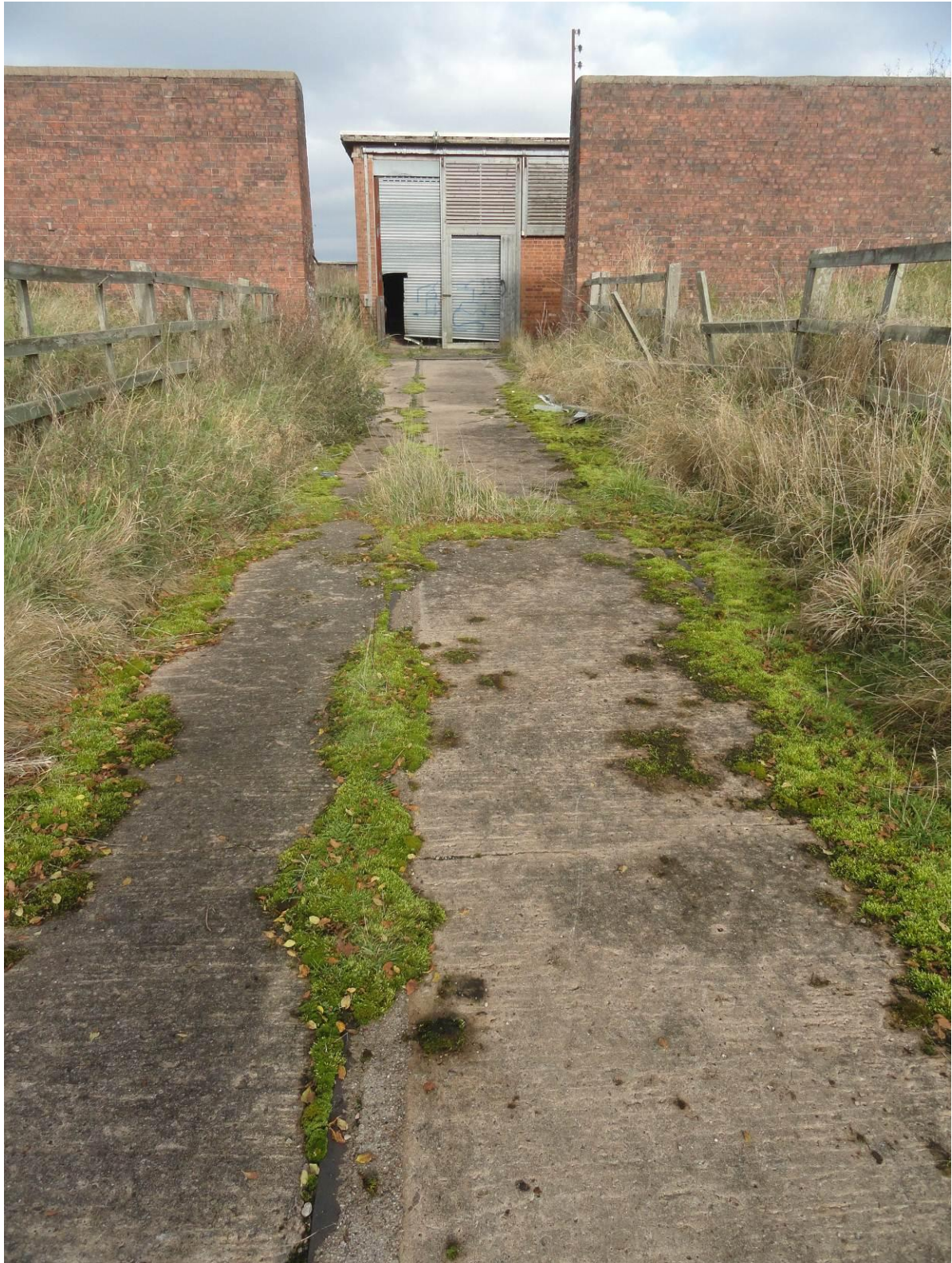
Plate 26. Southern approach to Building 9.9, looking north
