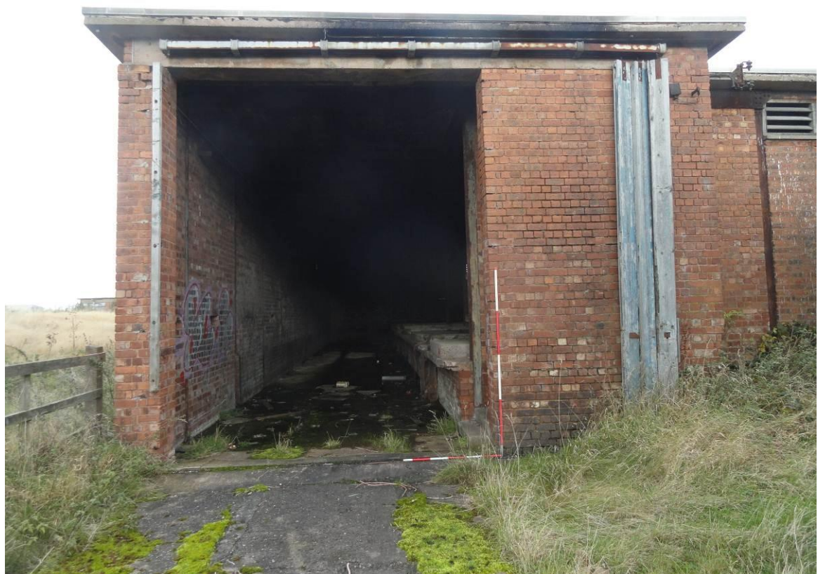
Plate 23. The southern entrance of Building 9.8, leading to loading bay
