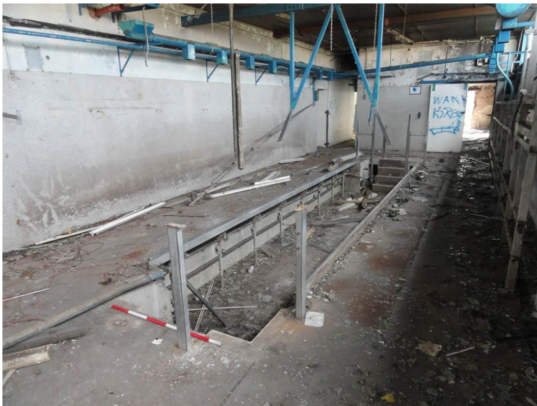
Plate 13. Western room within a subterranean chamber within Building 9.5, looking south
