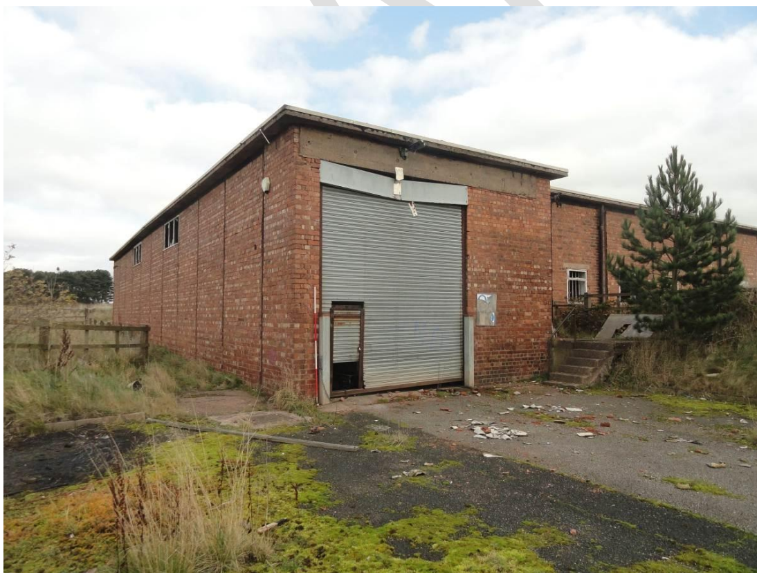
Plate 14. Roller-shutter entrance leading into loading platform area of Building 9.6, looking NE
