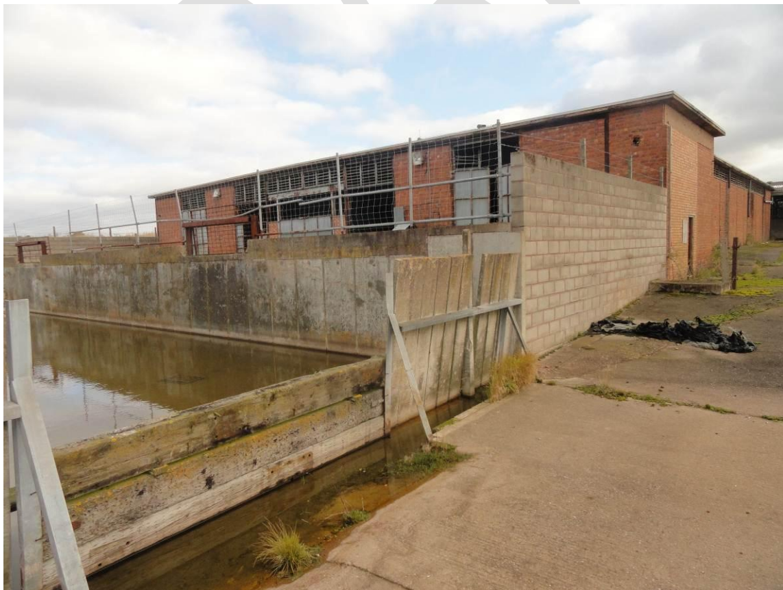
Plate 8. Building 9.4, modified and recently utilised as a cattle shed, looking NE
