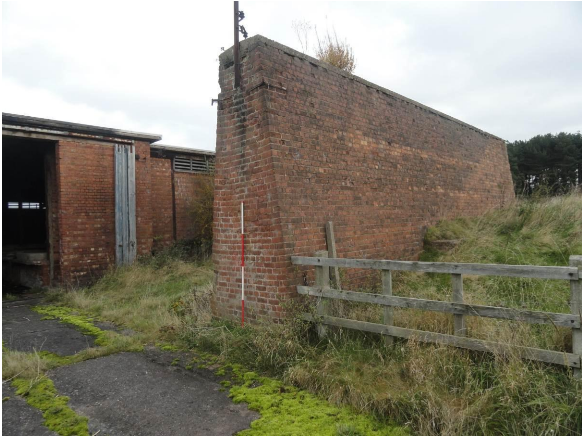
Plate 22. The eastern blast wall associated with Building 9.8, looking north-east
