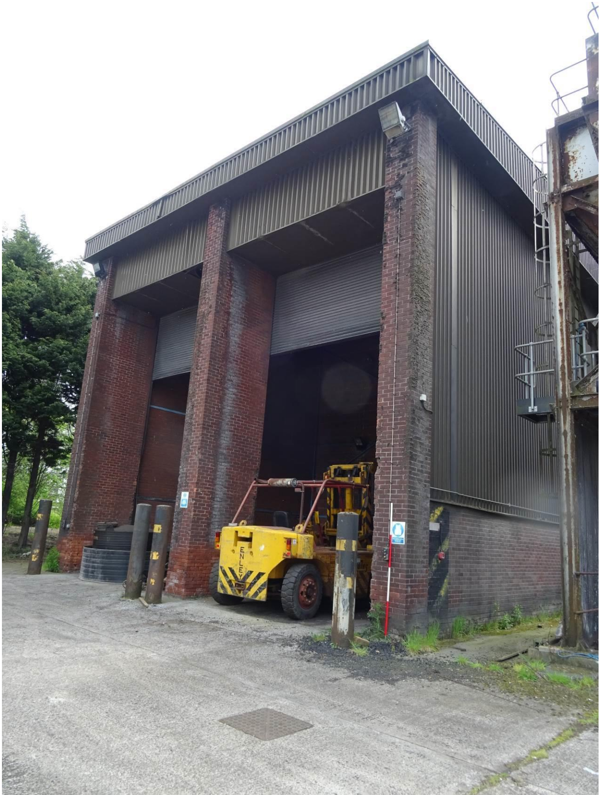
Plate 59. Fossil fuel grading unit, located at the NE end of the building
