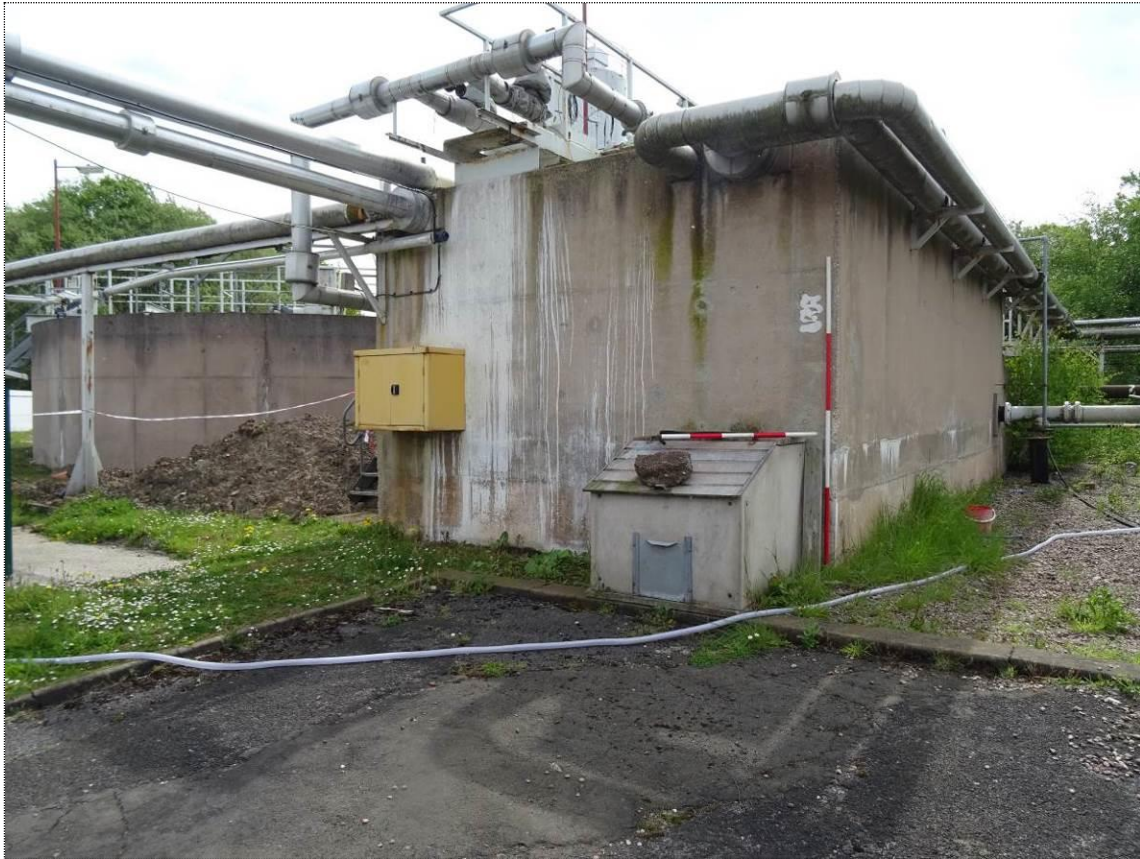
Plate 20. Northern section of the Final Neutralisation Tank (Building 4), looking south
