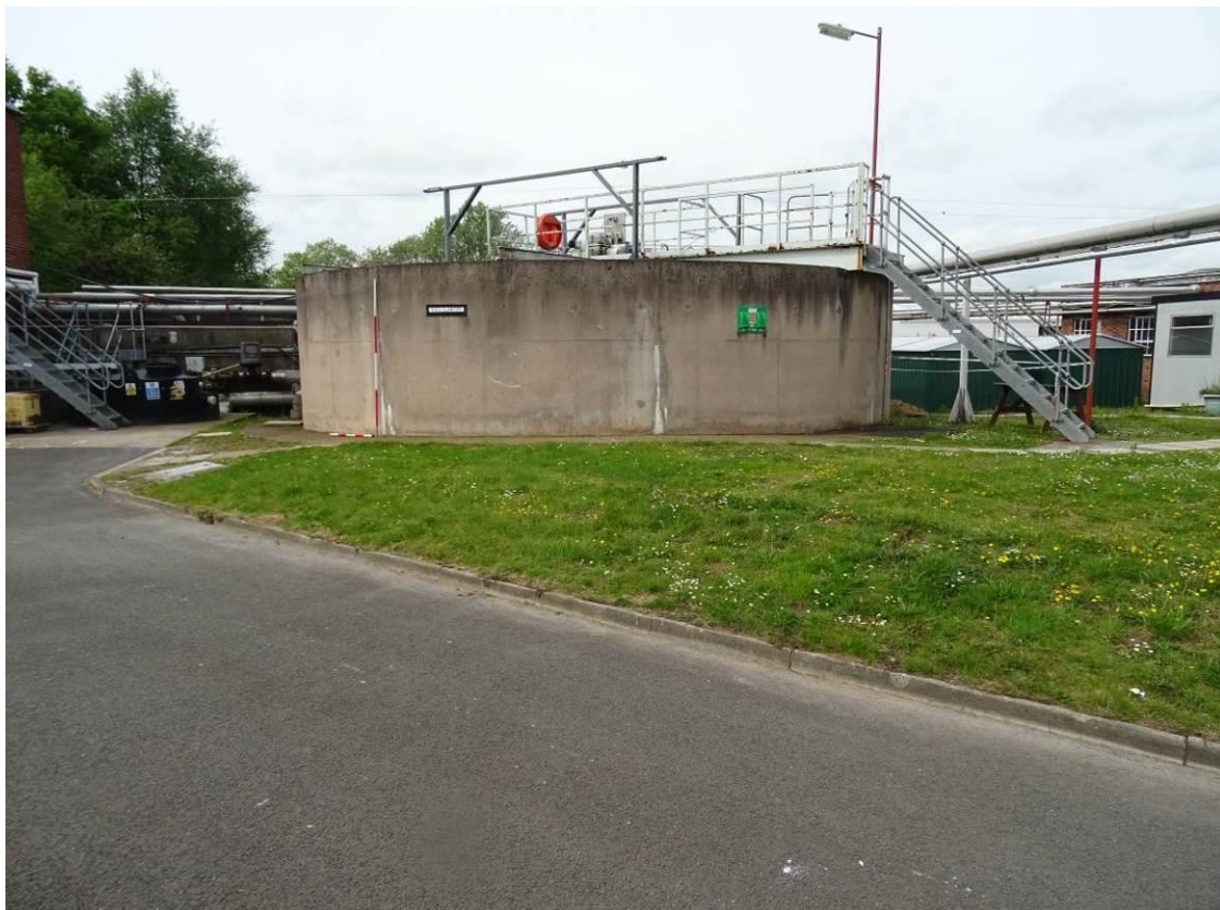
Plate 15. View of the effluent treatment tank (Building 2), looking SE
