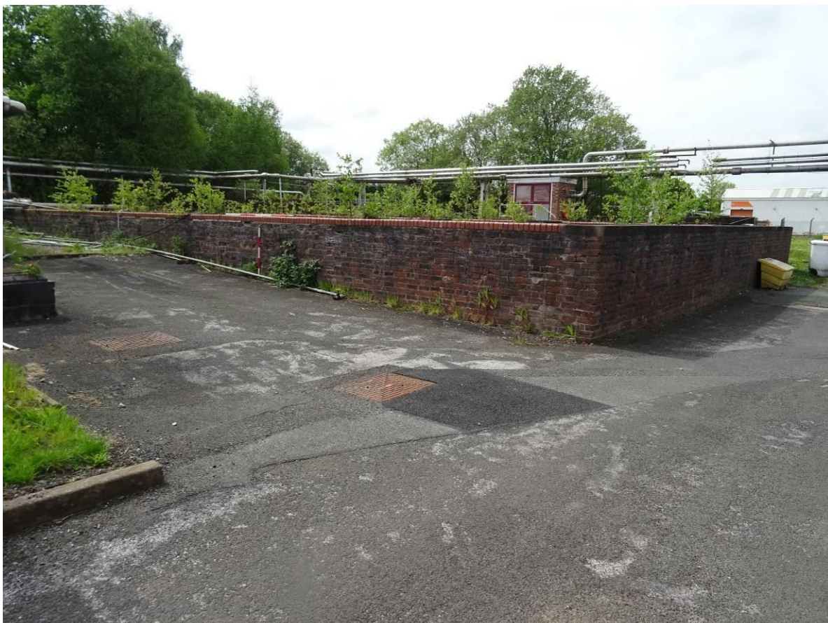
Plate 23. NE section of the second set of filtration tanks, looking SW
