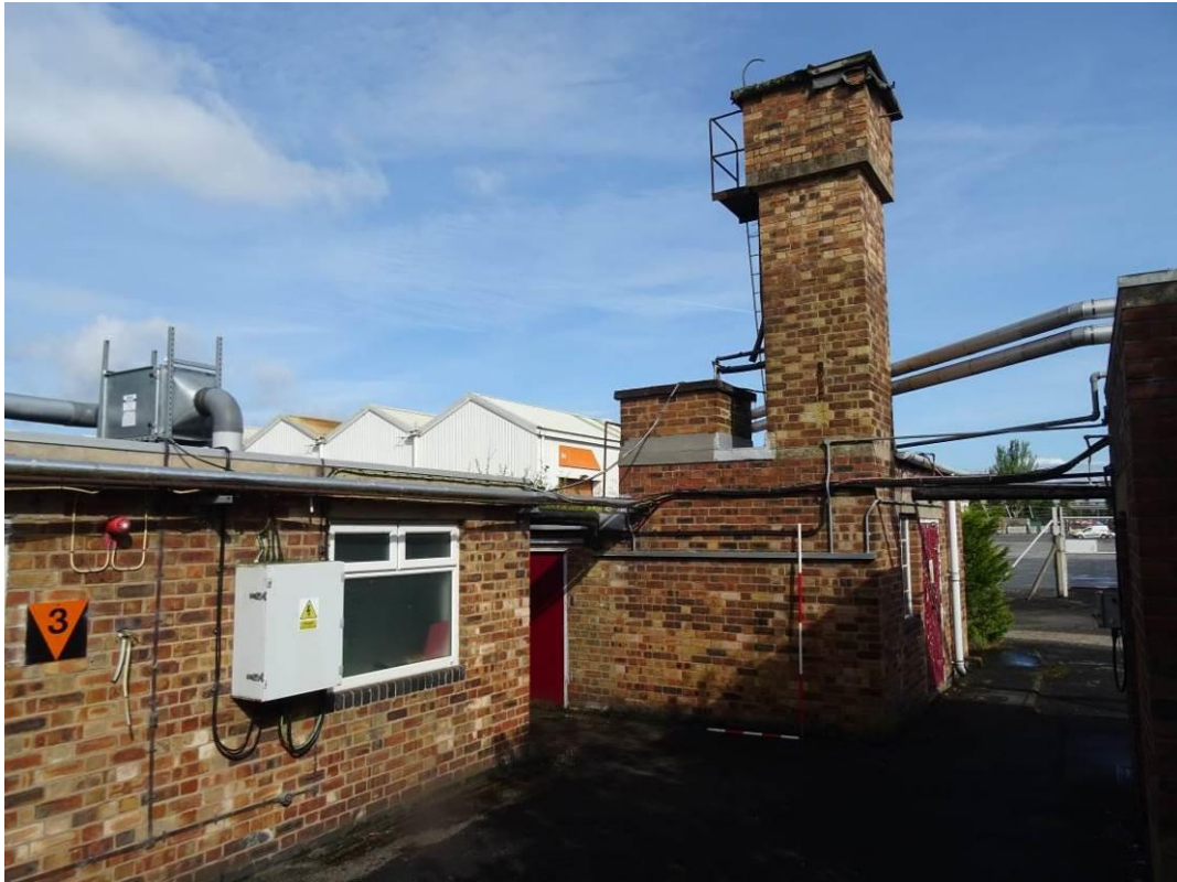
Plate 5. Ancillary buildings A (foreground) and B (with water tower), located west of the main Firing Range Complex, looking north
