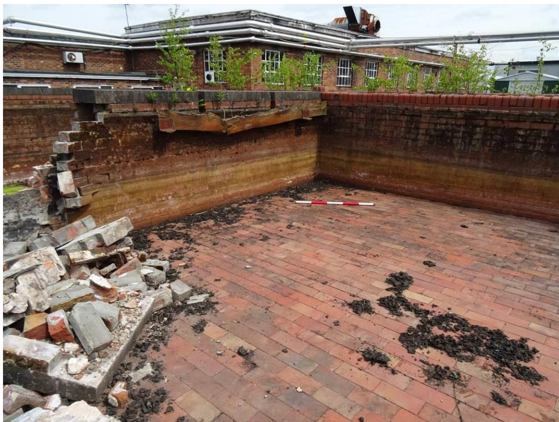
Plate 26. One of ten individual tanks with a brick-lined floor, looking north
