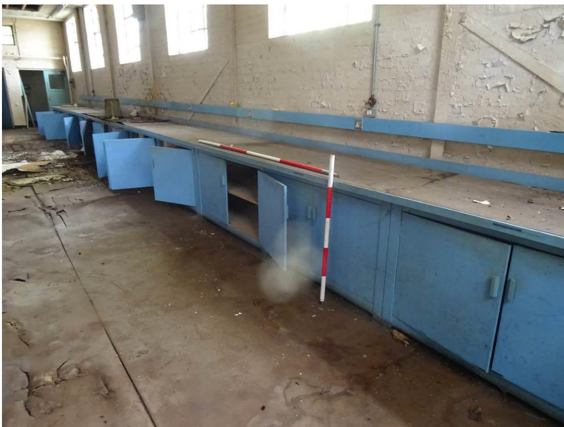
Plate 48. A row of laboratory benches built up against the northern [gable] wall, looking west
