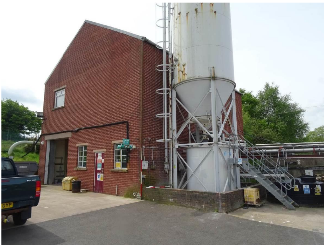
Plate 16. A recently-constructed effluent treatment building (Building 3) with adjoining silo, looking SW
