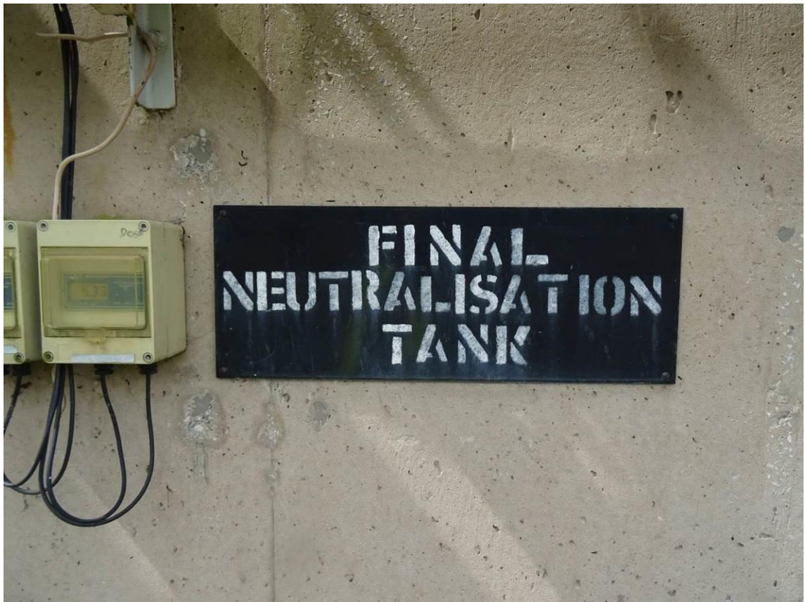
Plate 19. Make-shift signage located on the 'Final Neutralisation Tank' (see Plate 20)
