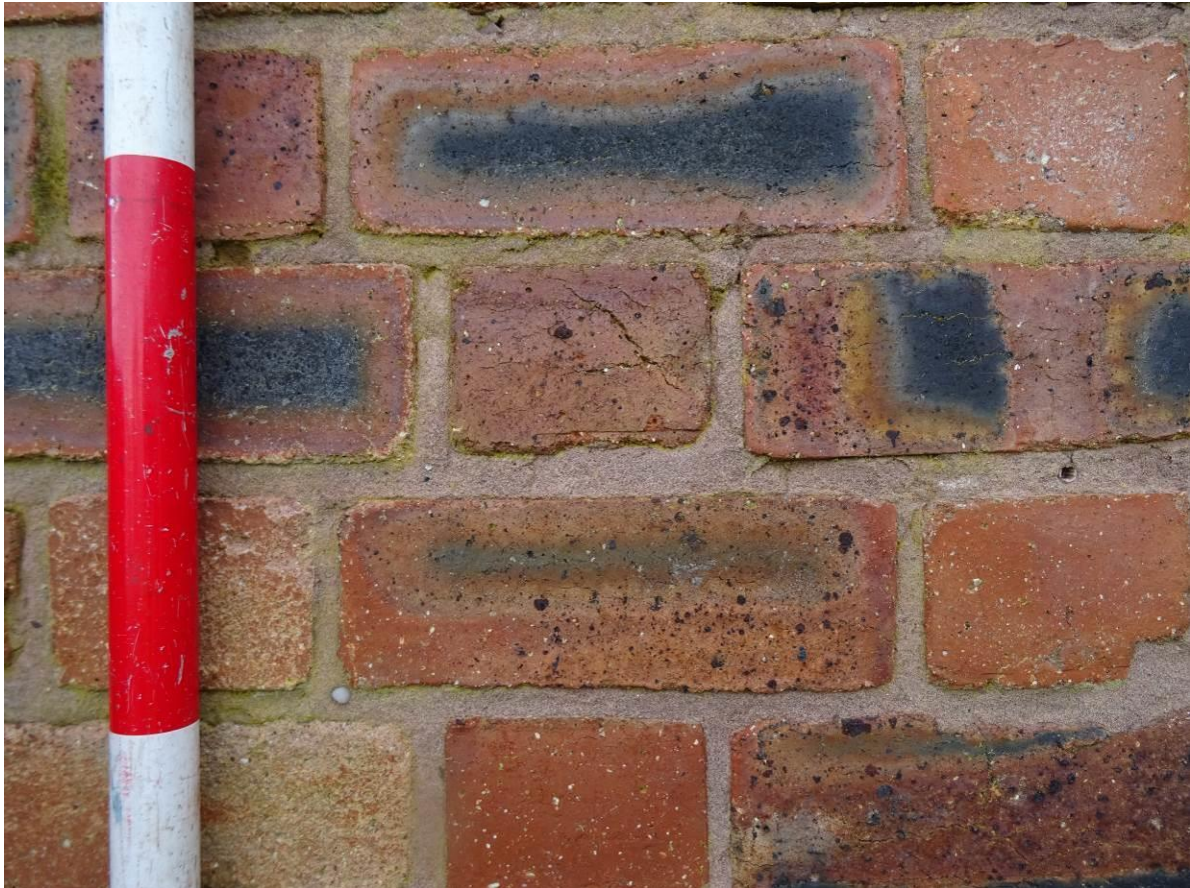
Plate 13. Sample of the brickwork from the northern elevation of Building E
