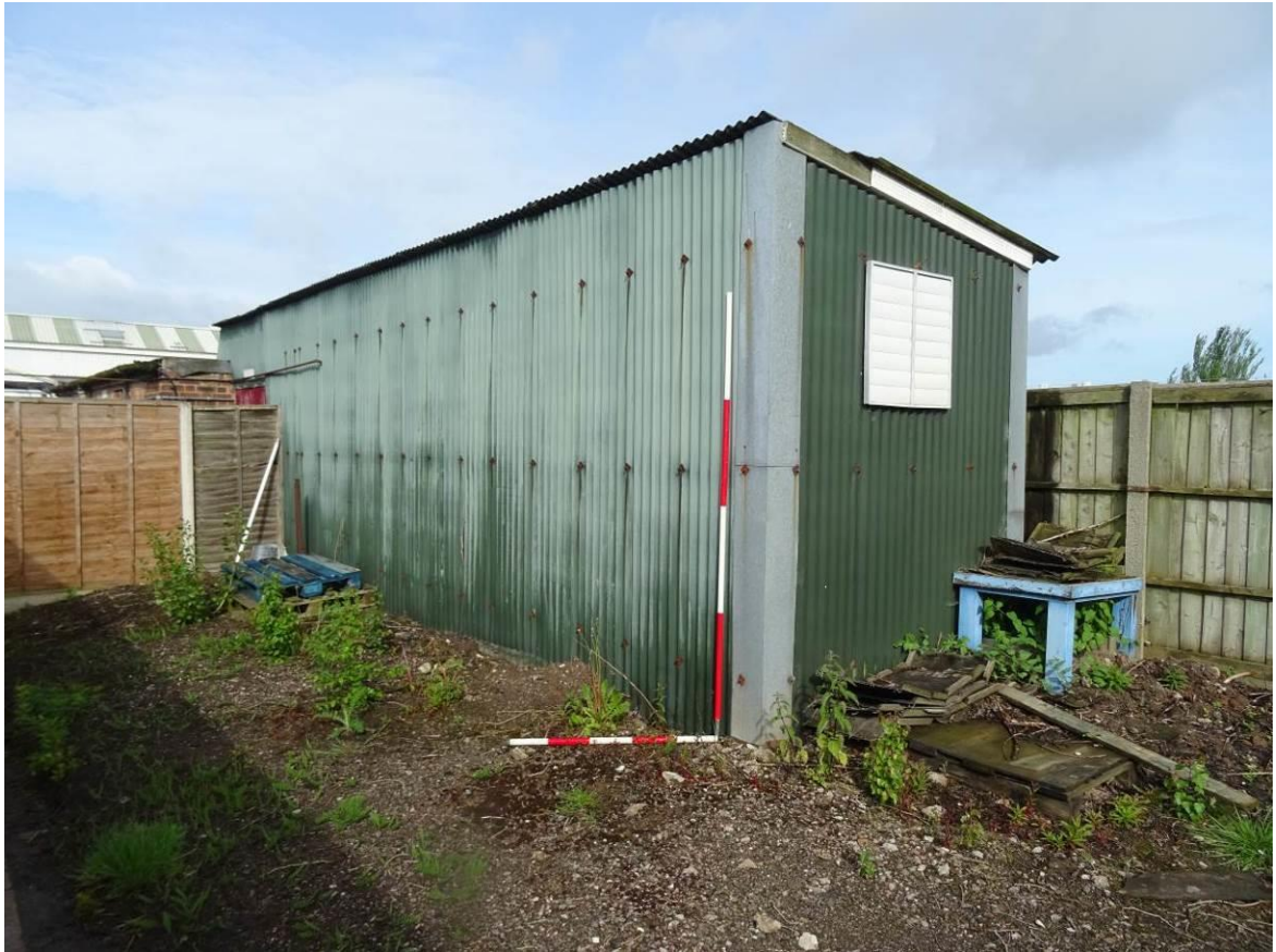
Plate 11. Corrugated lean-to shed, located along the north boundary of the Firing Range, looking N
