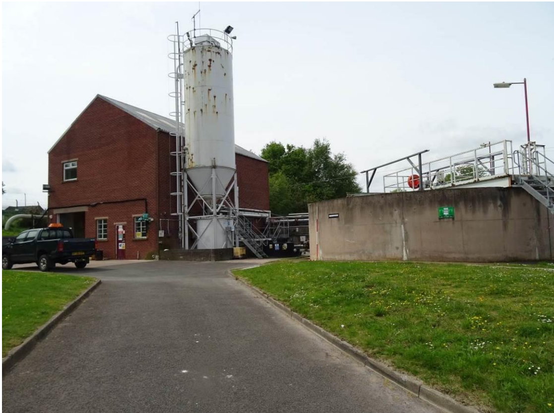
Plate 14. General view of the effluent treatment plant (Buildings 2 and 3), looking SE
