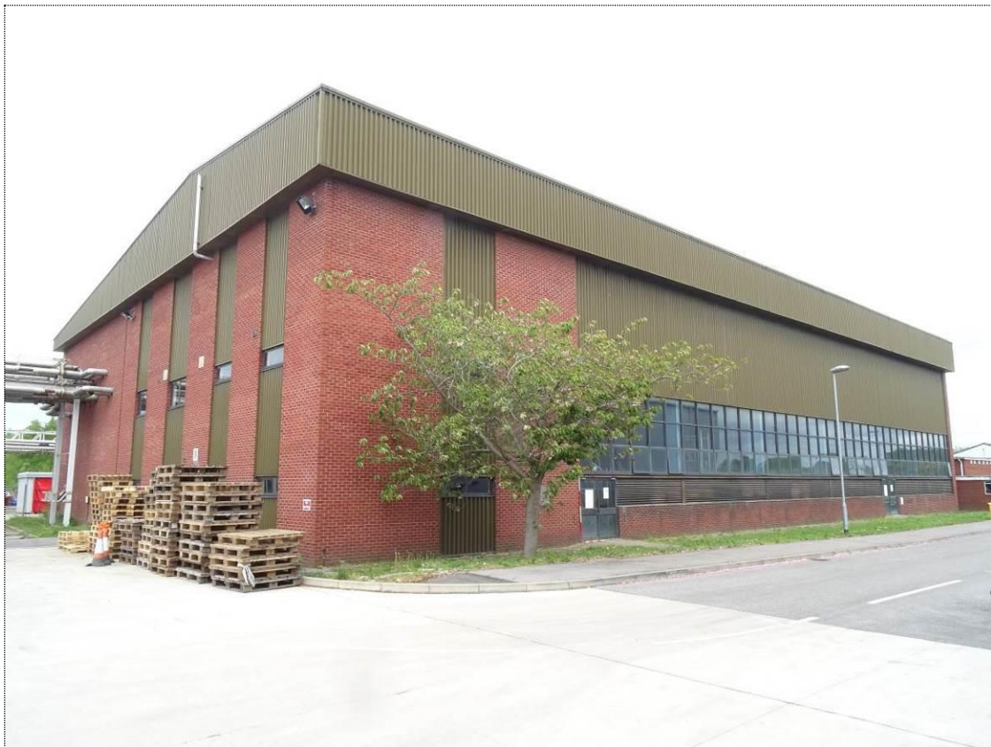
Plate 54. View of the northern section of the building, looking north
