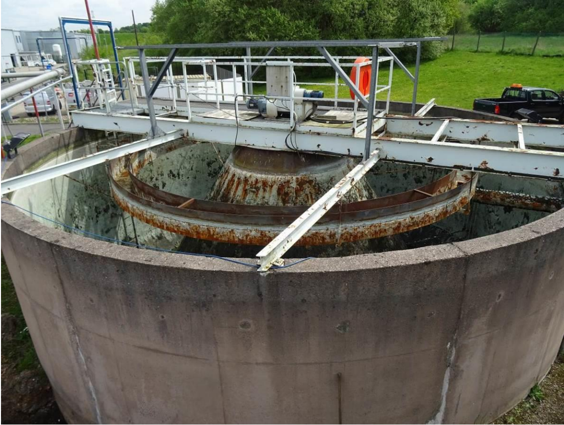
Plate 18. Above view of the effluent treatment tank (Building 2), looking NE
