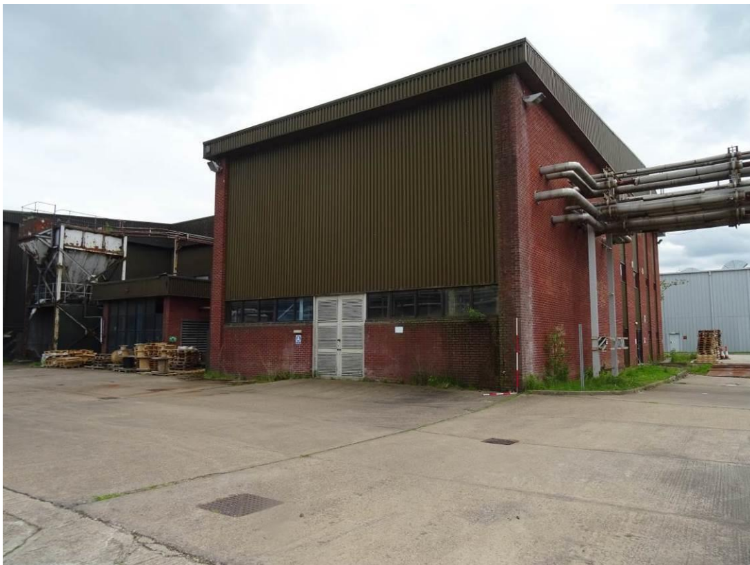
Plate 52. Rear section of the Boiler House and the courtyard, looking SE
