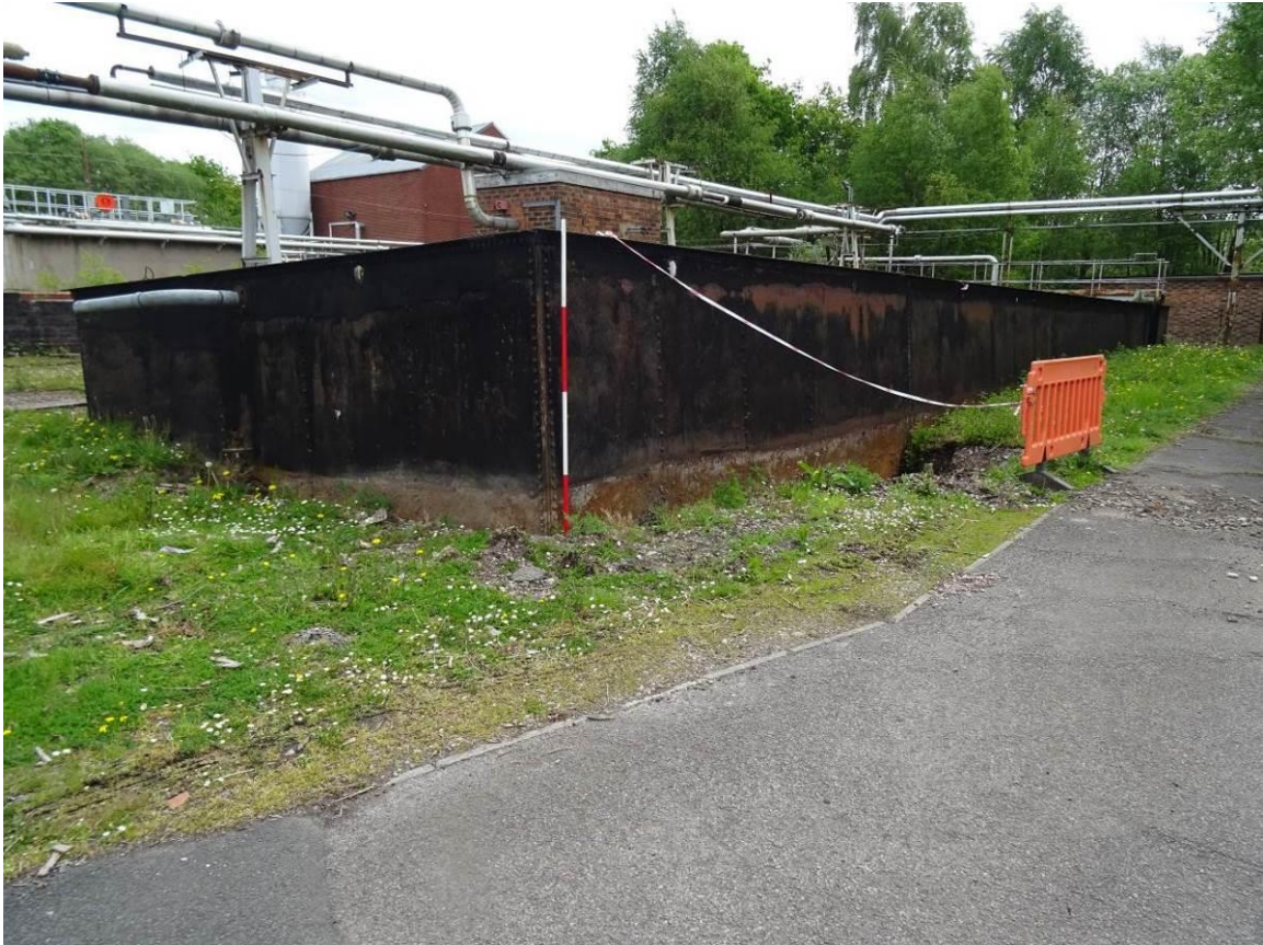
Plate 28. The earliest filtration tank (Building 6), constructed of riveted iron plates and located SW of the later tank system (Building 5), looking SE
