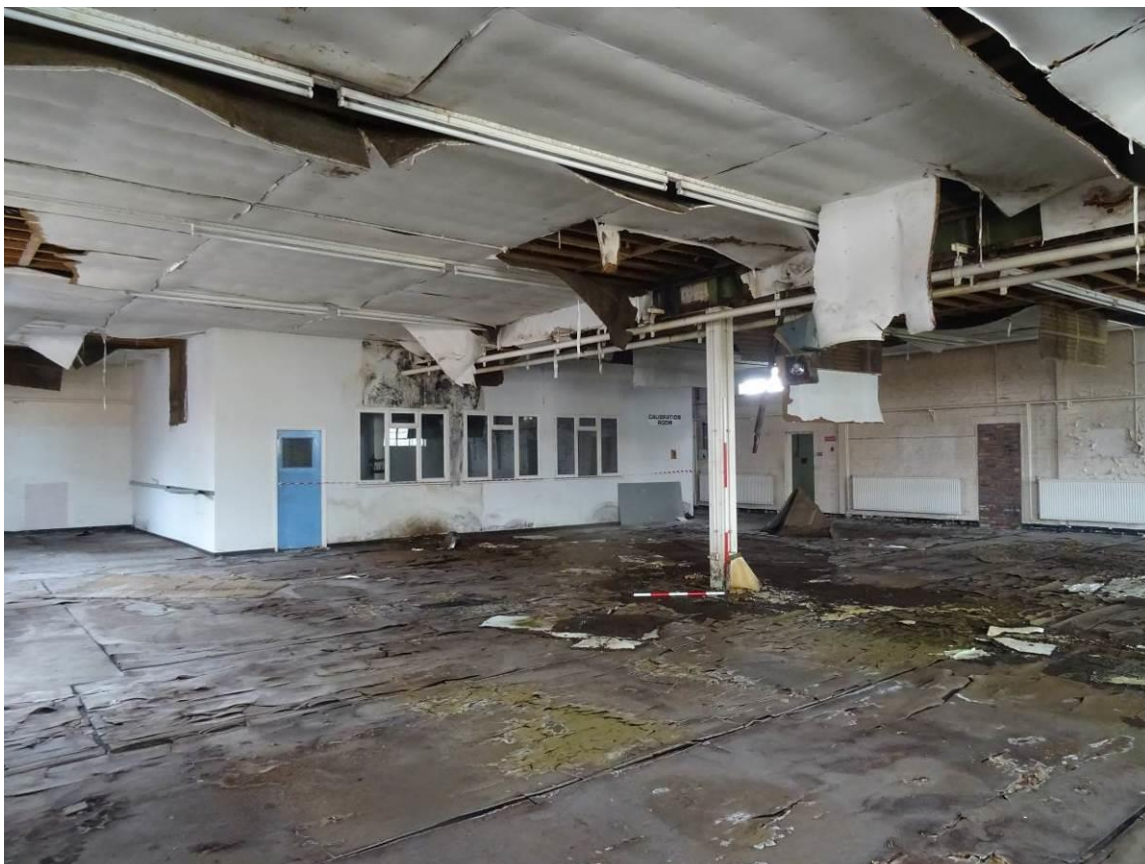
Plate 47. The principle [northern] laboratory room and shop-floor offices, looking SE
