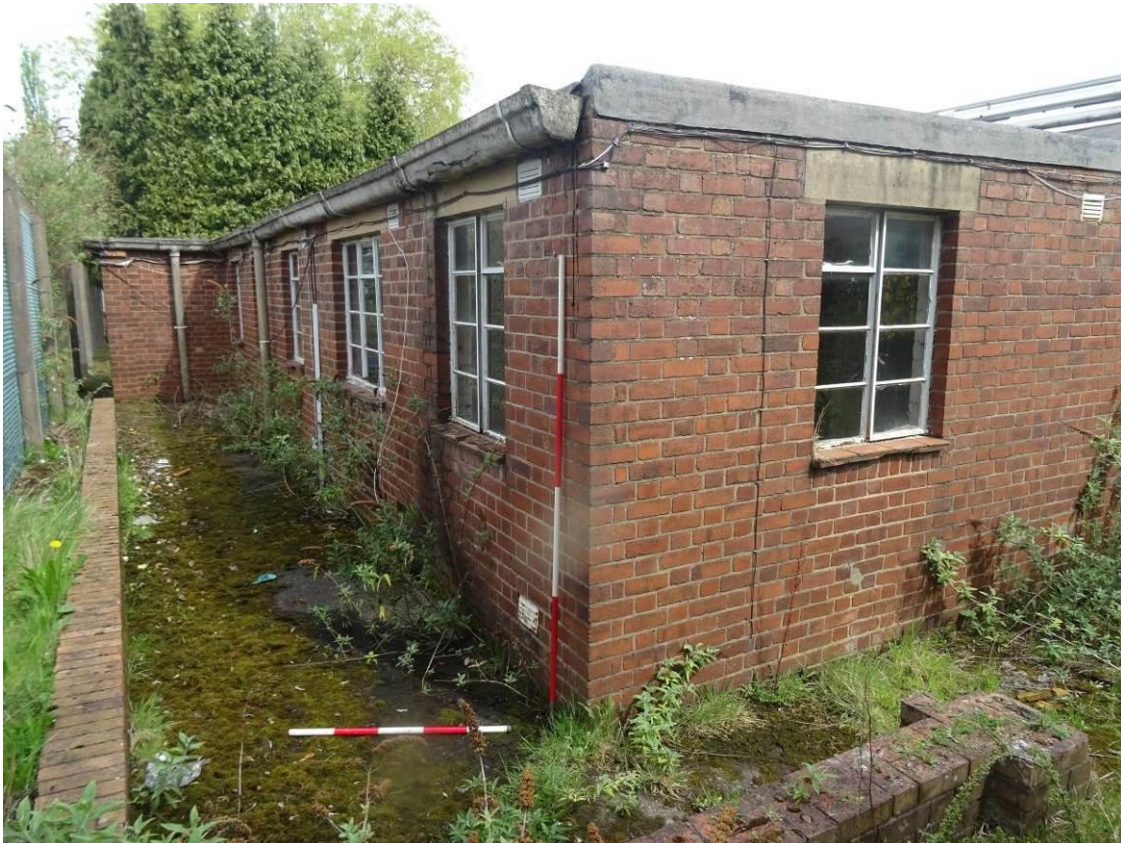
Plate 37. Rear [western] section of the building (offices), looking north
