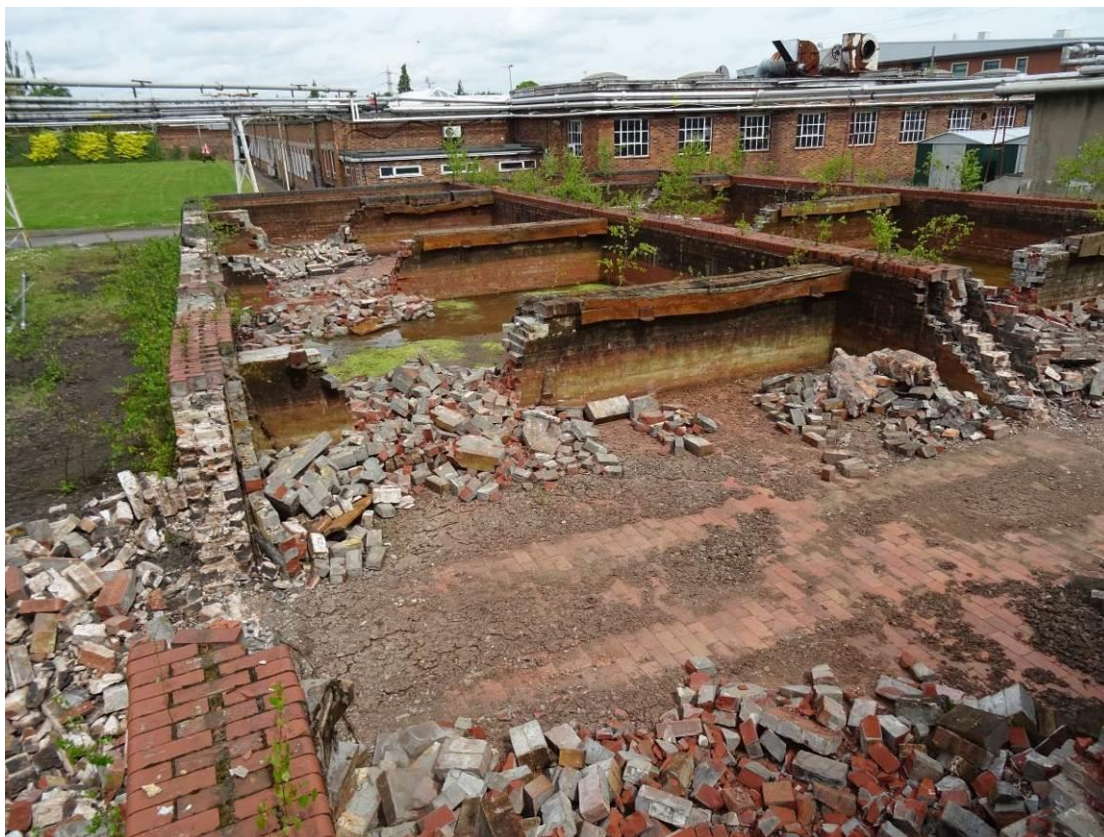
Plate 25. Overhead view of the second set of filtration tanks showing individual brick sections, looking north
