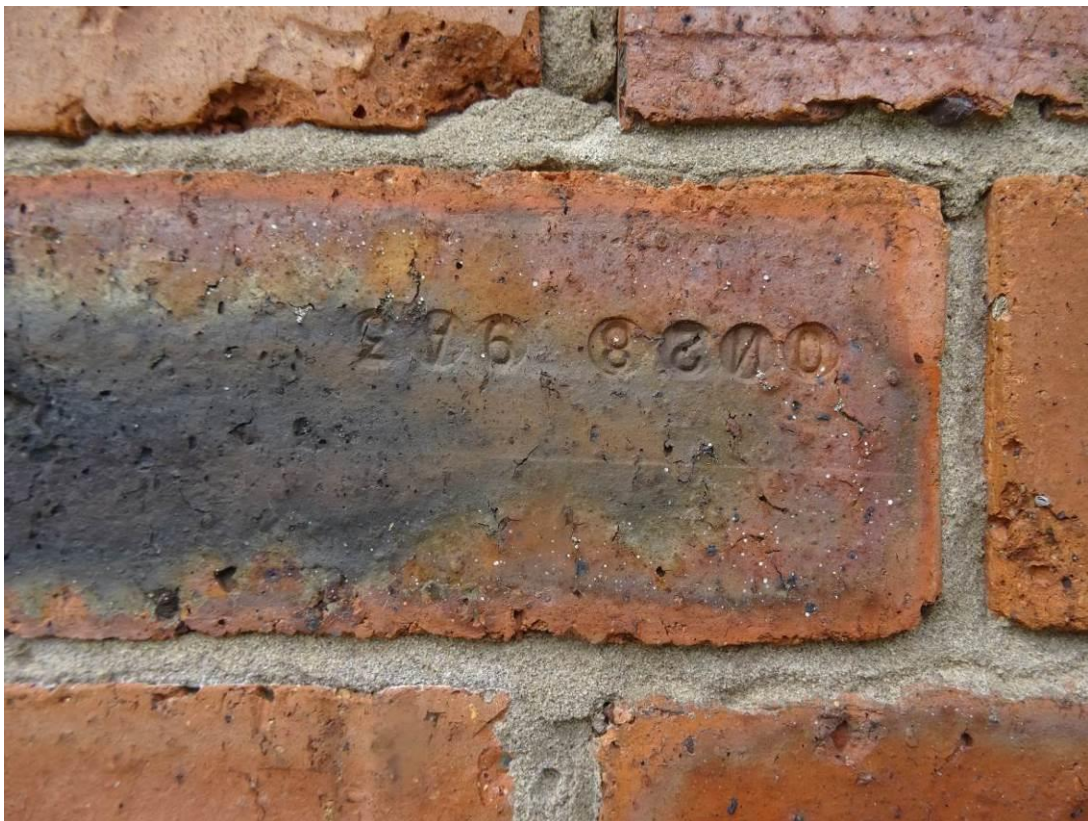
Plate 33. Brick sample from the NE elevation showing batch manufacture code
