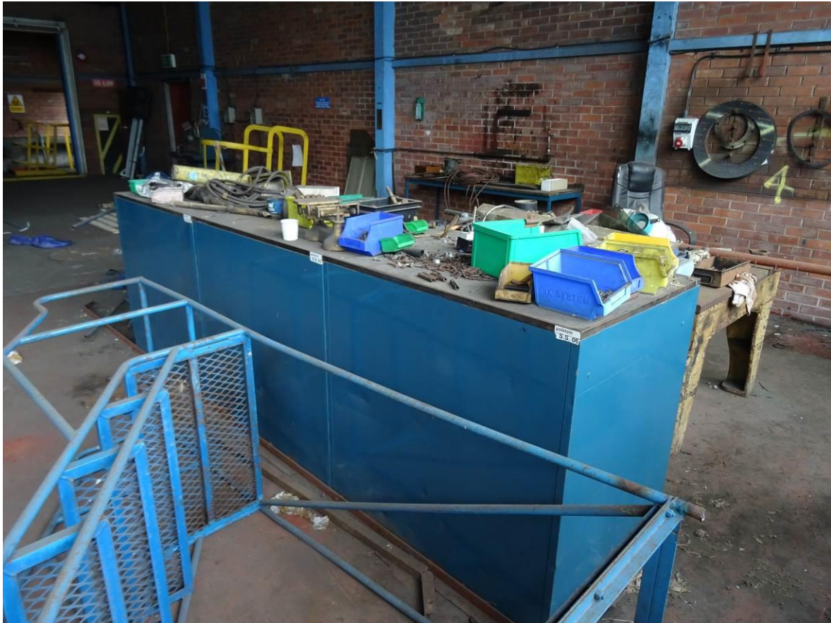
Plate 66. Maintenance area within the principle room of the boiler house
