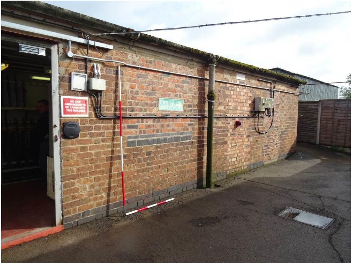
Plate 12. The southern elevation of the Gunnery Room (Building F), looking nor
