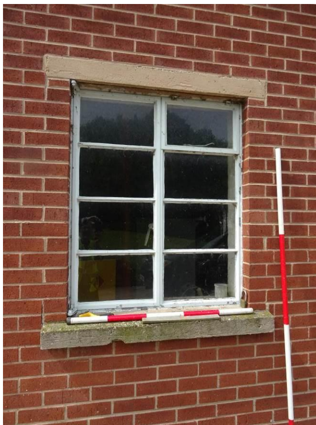
Plate 17. Detail of the window casement, located on the NE elevation
