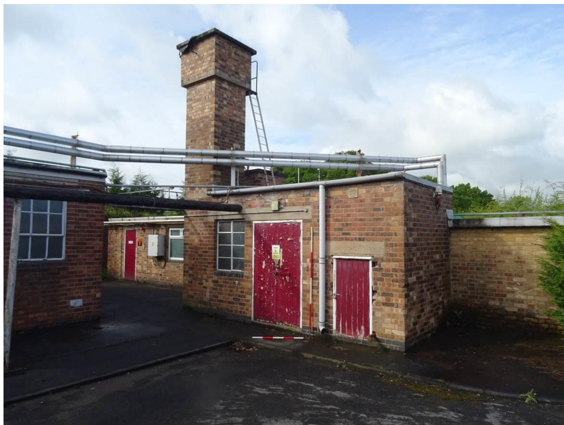
Plate 4. Eastern ancillary building (B), located west of the Firing Range Complex, looking
