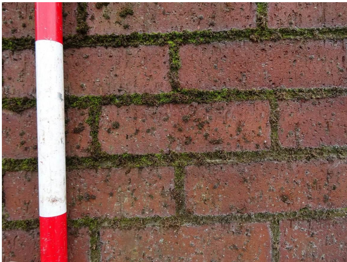
Plate 55. Sample section showing the brickwork
