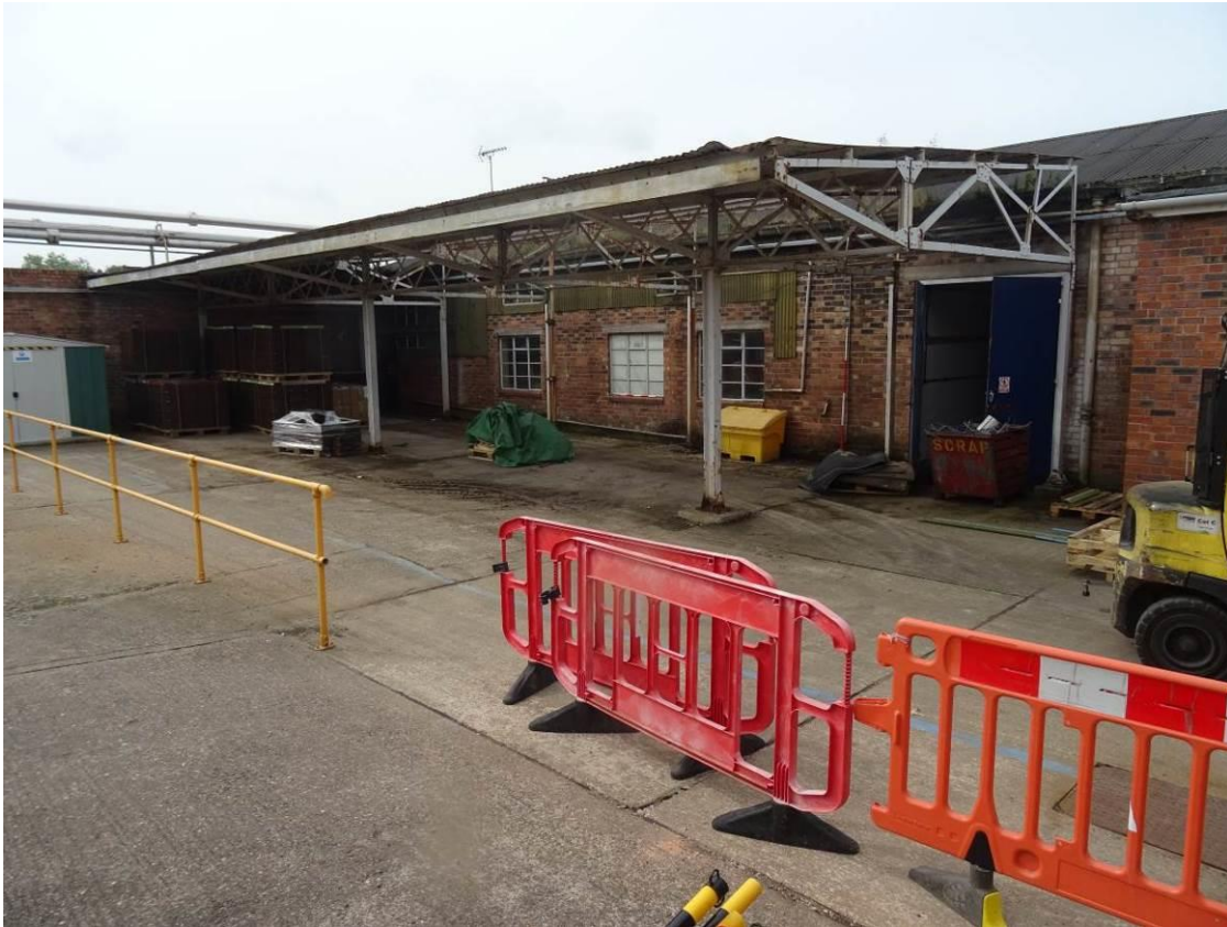
Plate 30. General view of the NE elevation, looking south
