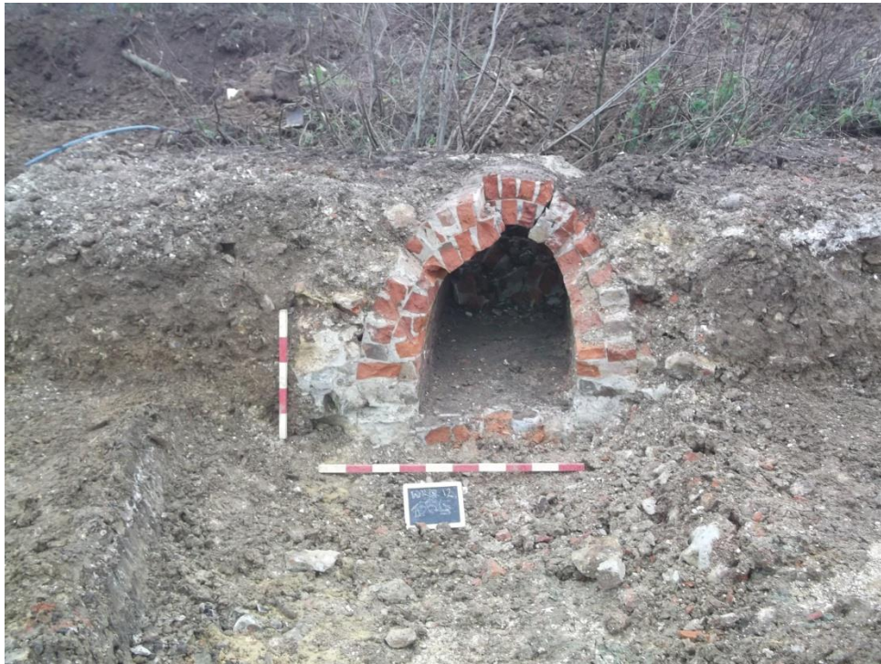
Figure 34: Culvert (501) facing west
