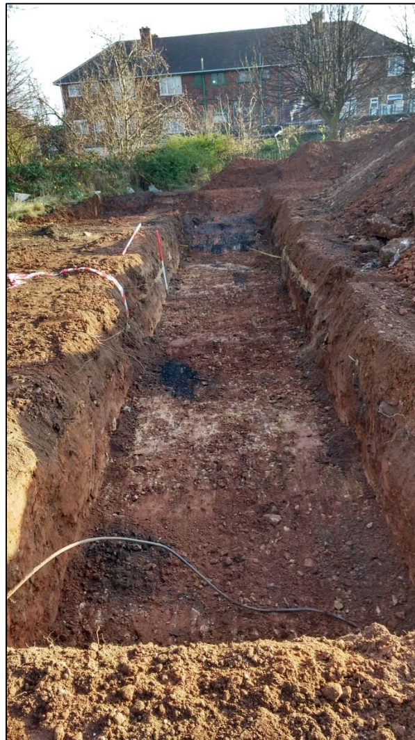
Figure 13 Trench 6 looking south east
