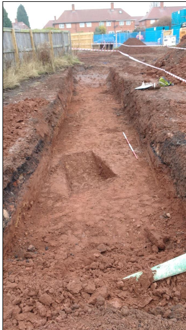
Figure 4 Trench 2 looking north west
