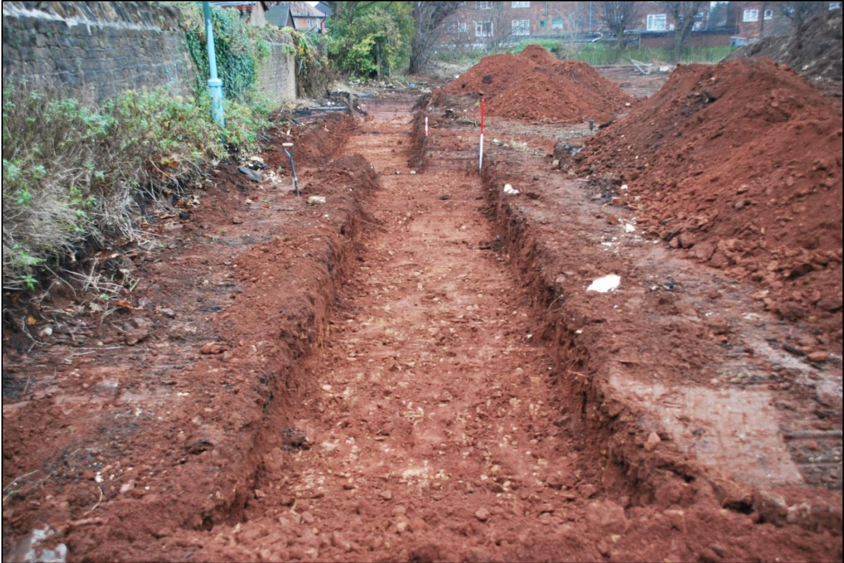
Figure 8 Trench 4 looking west-north-west
