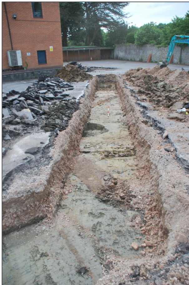
Figure 10 Trench 6 looking WSW
