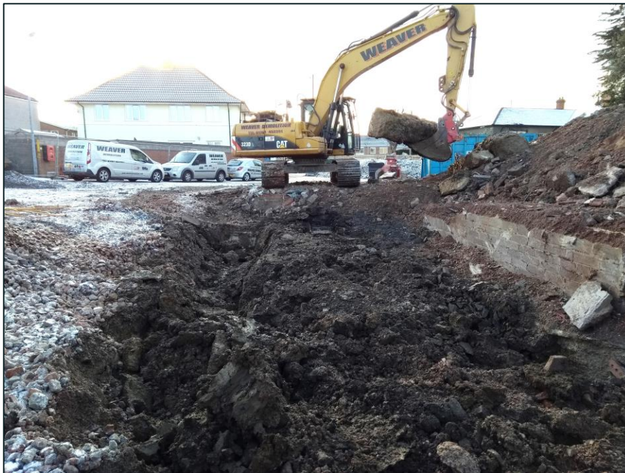
Figure 15 Removal of footings at north of former police station looking east
