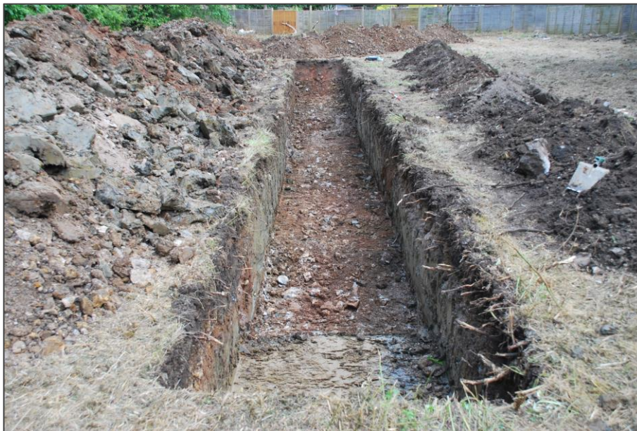
Figure 3 Trench 1 looking east
