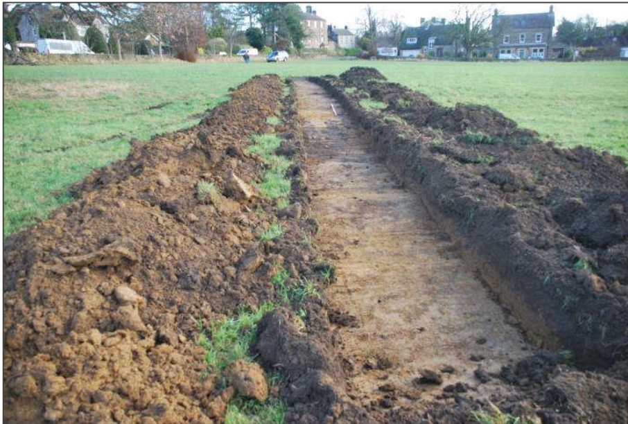
Figure 5-11 Trench 4 looking south east
