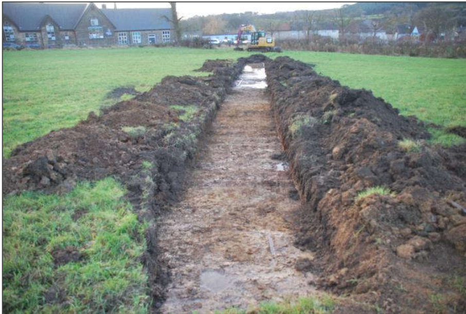
Figure 5-19 Trench 9 looking south
