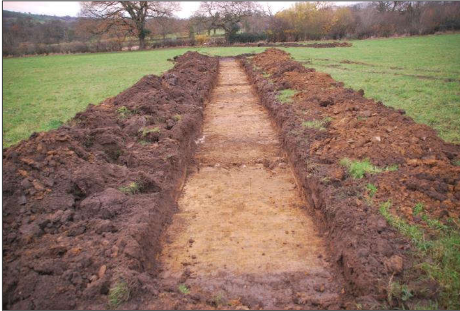
Figure 5-16 Trench 7 looking north west
