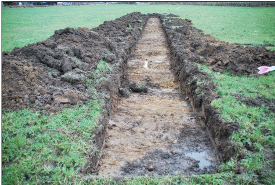
Figure 5-13 Trench 5 looking south
