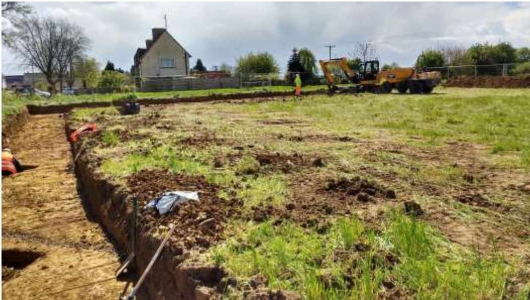
Plate 1: Stripping in progress, Greatworth village in view, facing south-southwest
