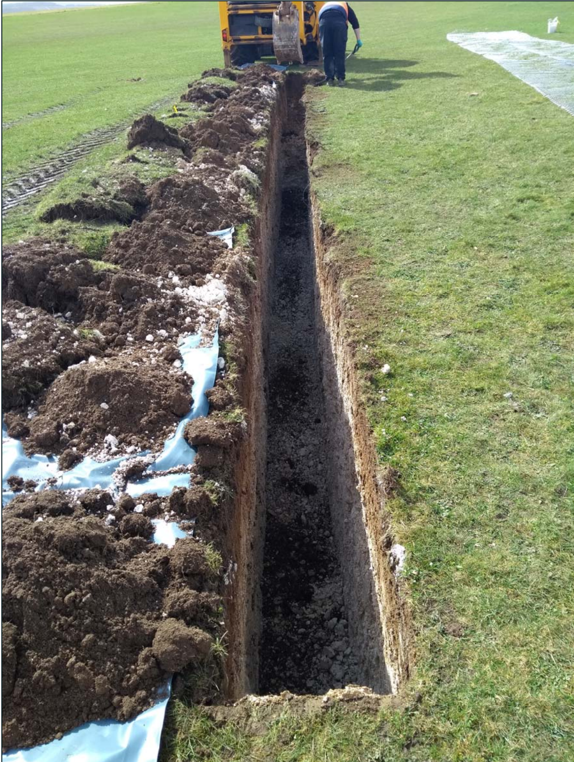
Figure 5 Northern end of trench looking SSW
