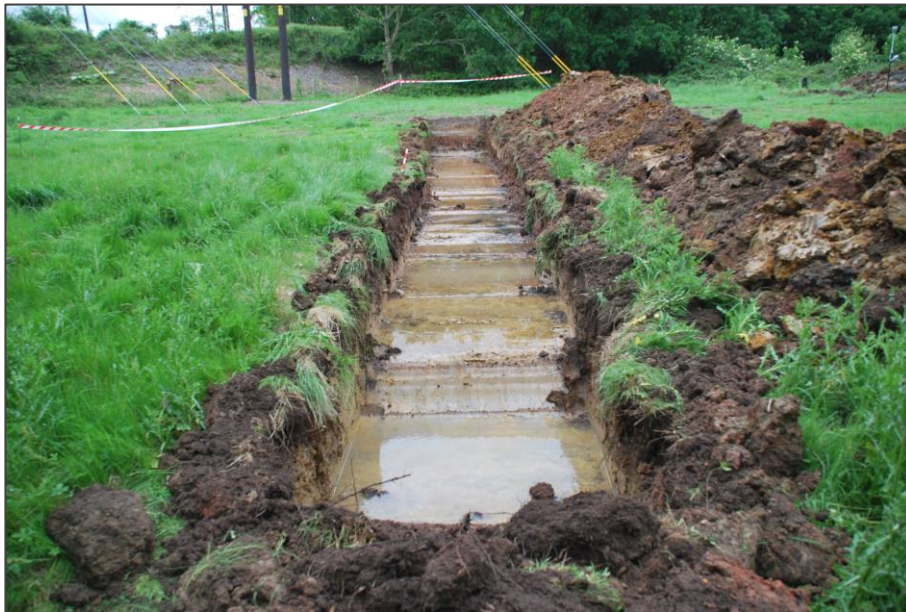
Figure 14 Trench 9 looking north west
