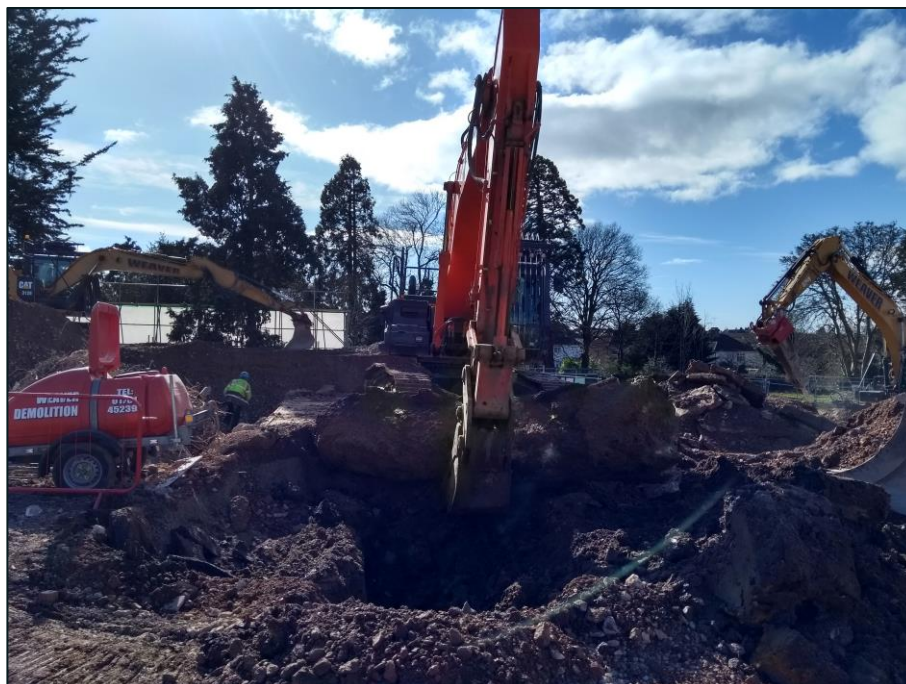
Figure 17 Removal of footings towards eastern end of former police station site looking south
