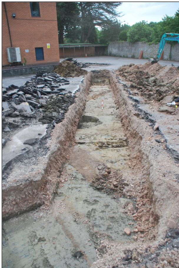
Figure 10 Trench 6 looking WSW
