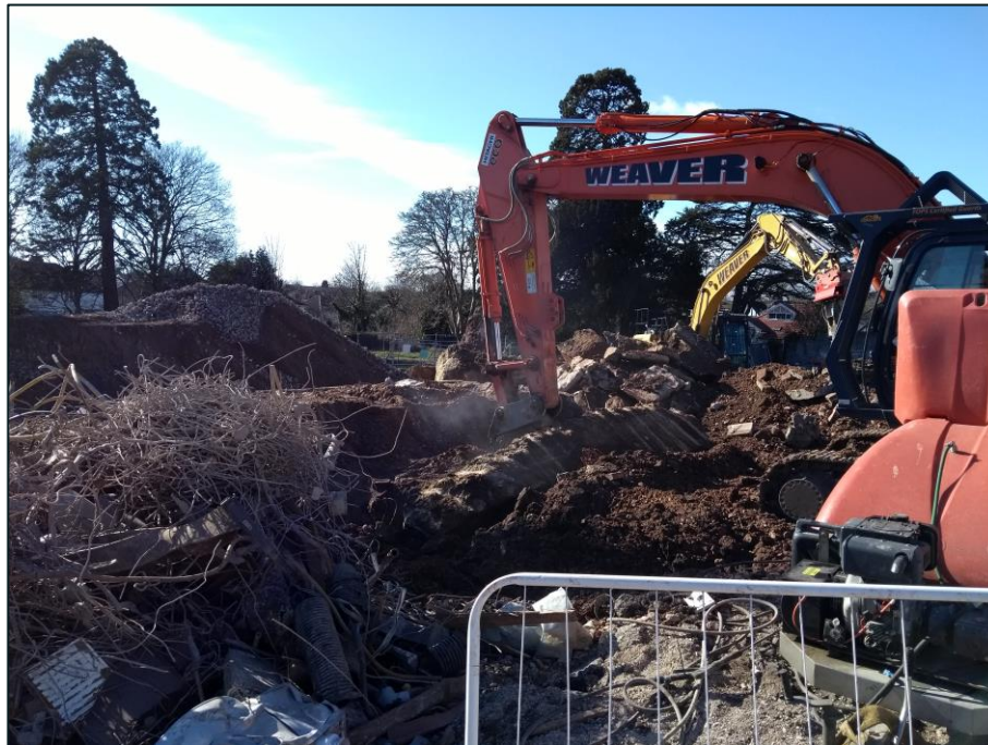
Figure 16 Removal of footings at south of former police station looking south west
