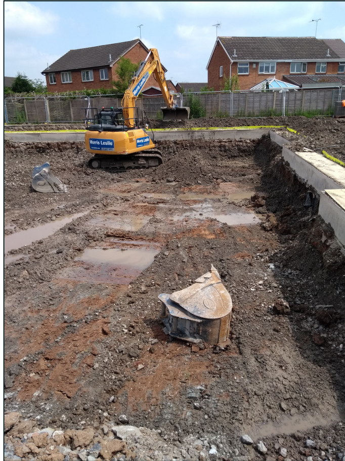
Figure 5-4 Phase 2 Basement area looking north east
