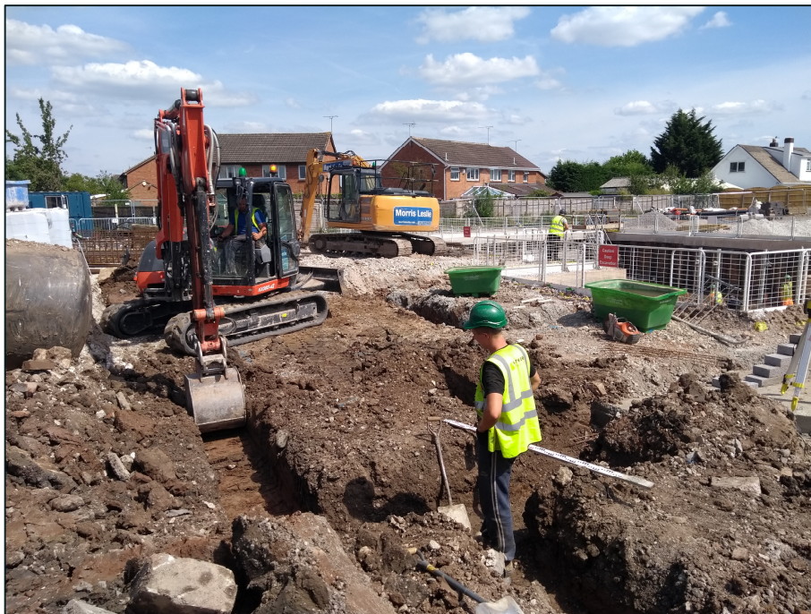
Figure 5-6 Excavation of Phase 3 foundations looking east
