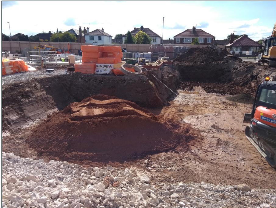
Figure 5-7 Phase 4 attenuation tanks area looking south west
