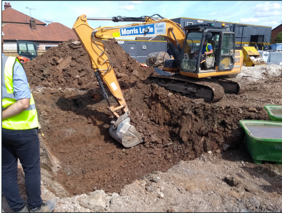
Figure 5-5 Removal of oil tank during Phase 3 looking north
