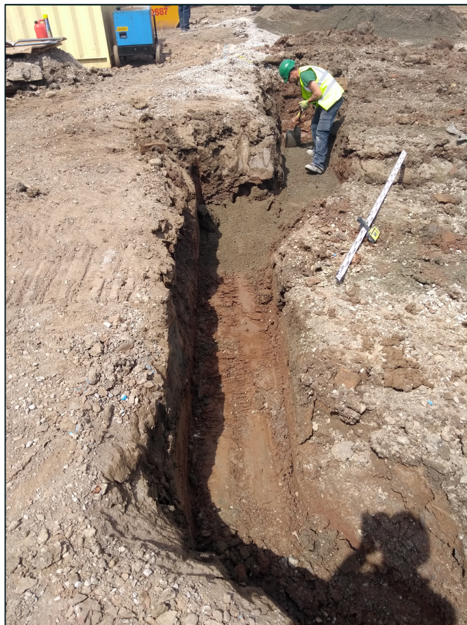
Figure 5-2 Foundation trench during Phase 1 of works looking north west
