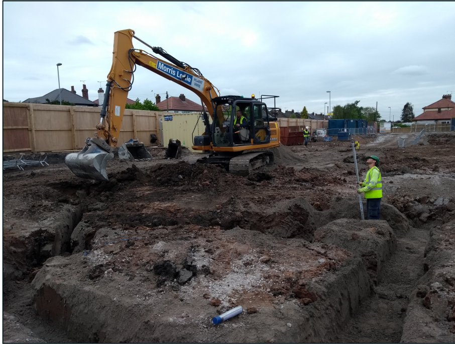
Figure 5-3 Excavation of foundation trenches during Phase 1 looking north west
