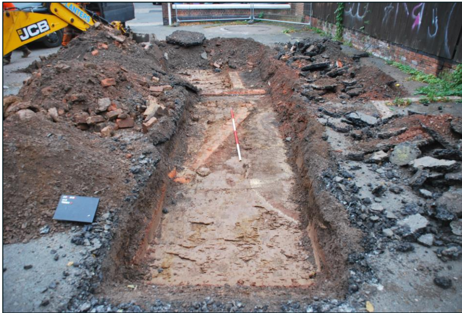
Figure 5-5 Trench 2 looking north west
