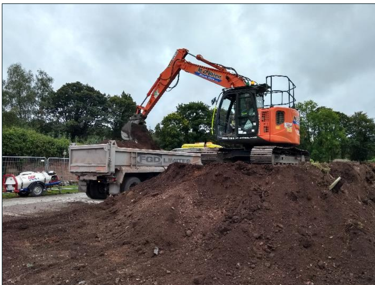
Figure 3-1 Central spoil heap being removed looking south west
