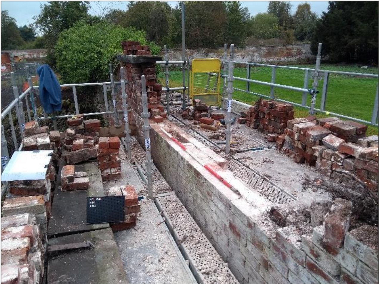
Figure 3-3 Area of garden wall after bricks taken down prior to rebuilding
