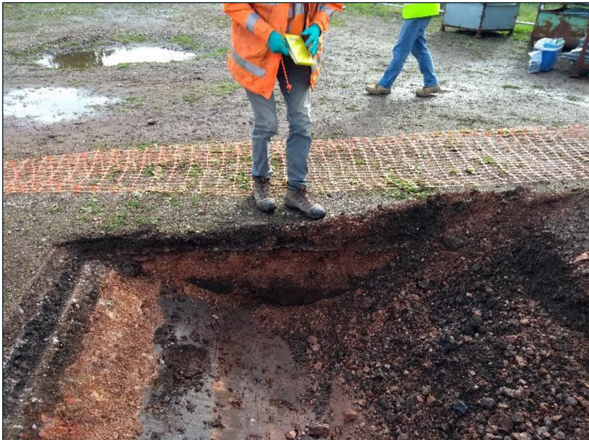
Figure 3-8 Test pit D1 looking south east
