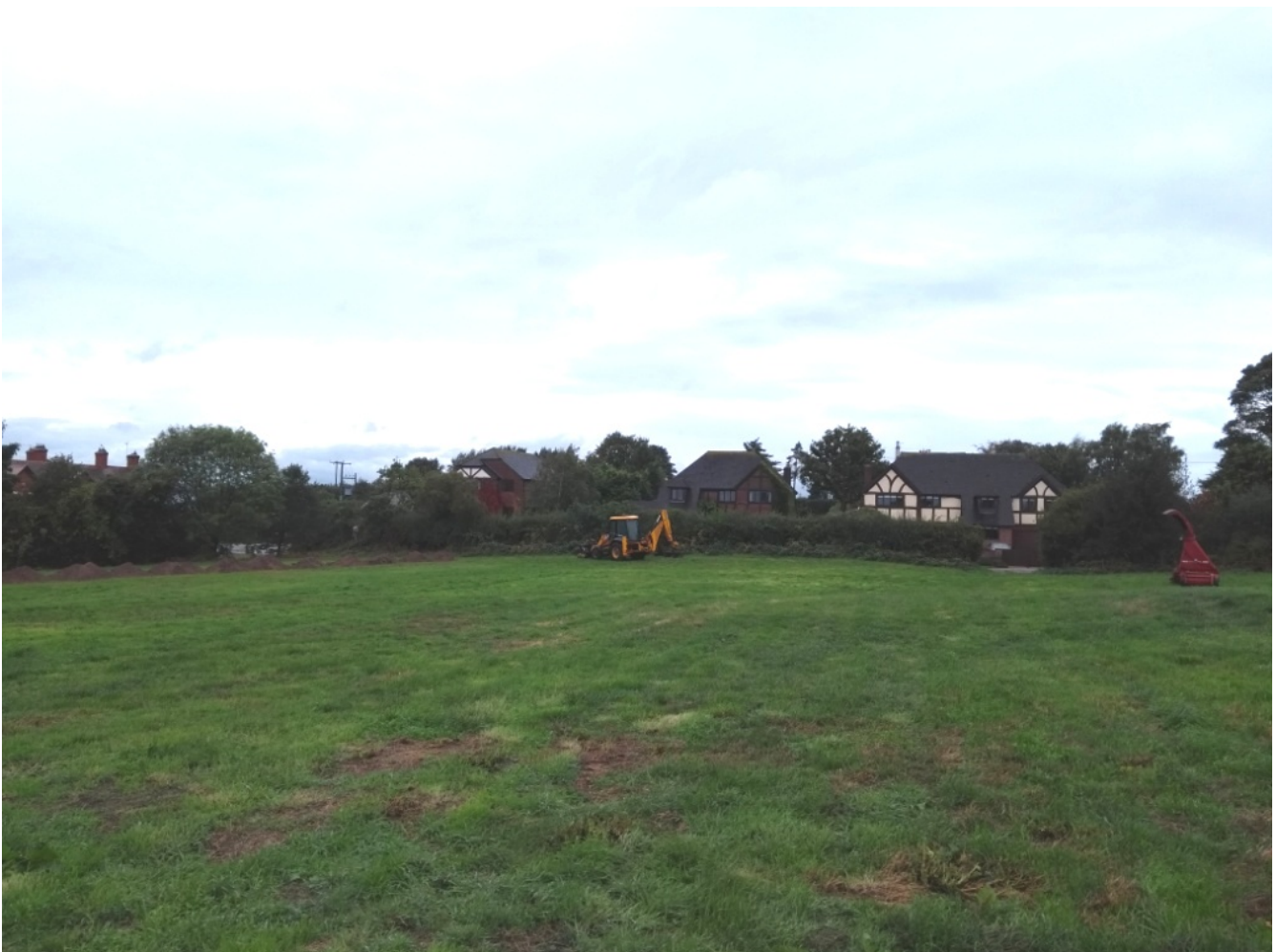
Figure 6 General view of West end of site and Trench 1
