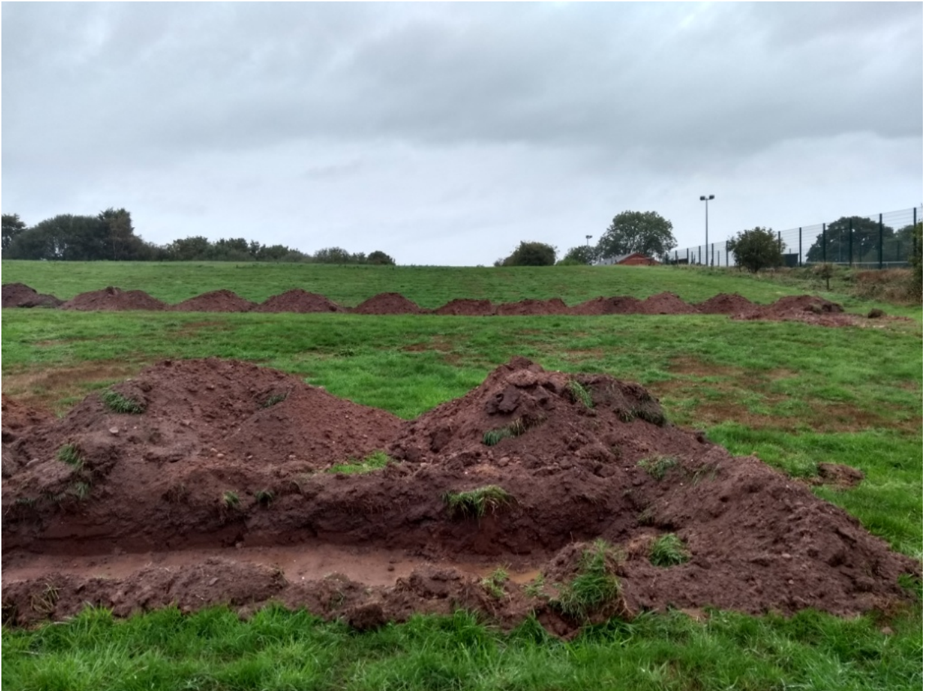
Figure 7 General view of East end of site
