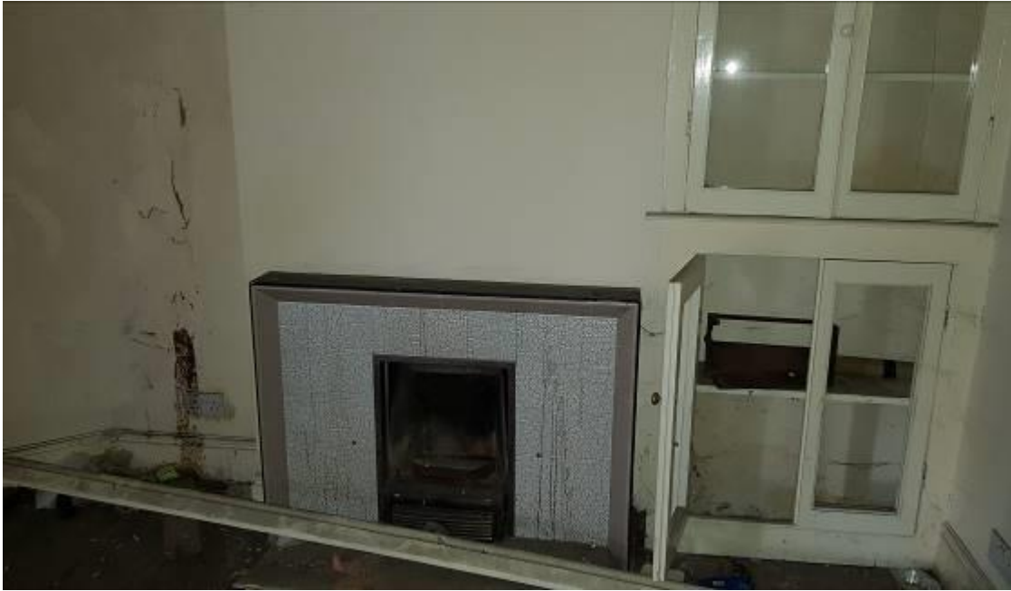
Plate 18: Bedroom 1 (north). Fireplace and surround. No scale.
