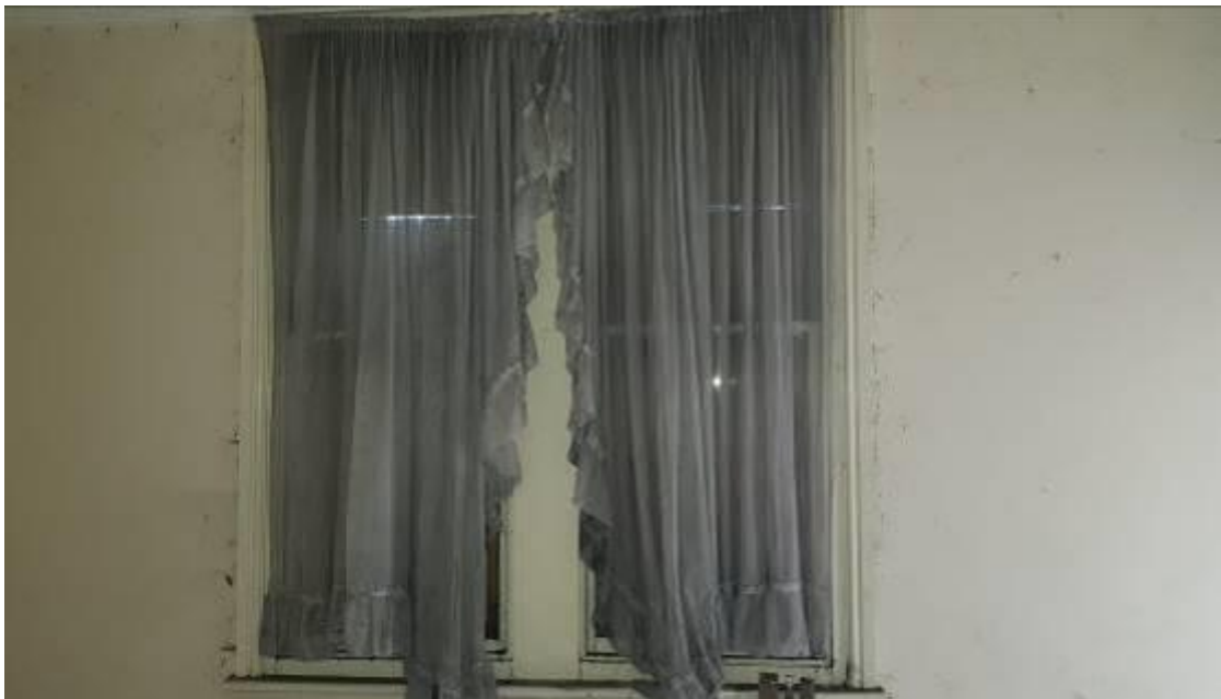
Plate 15: living room moulded window frame (lower floor). No scale.
