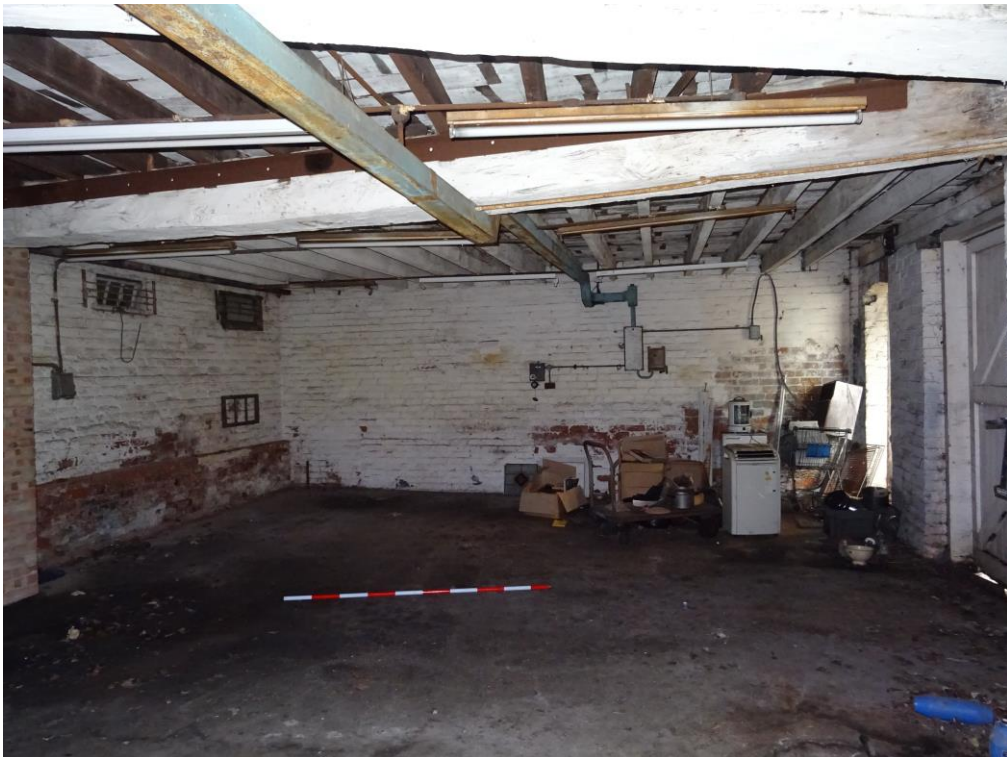
Plate 45: Section B western elevation. 2m scale.
