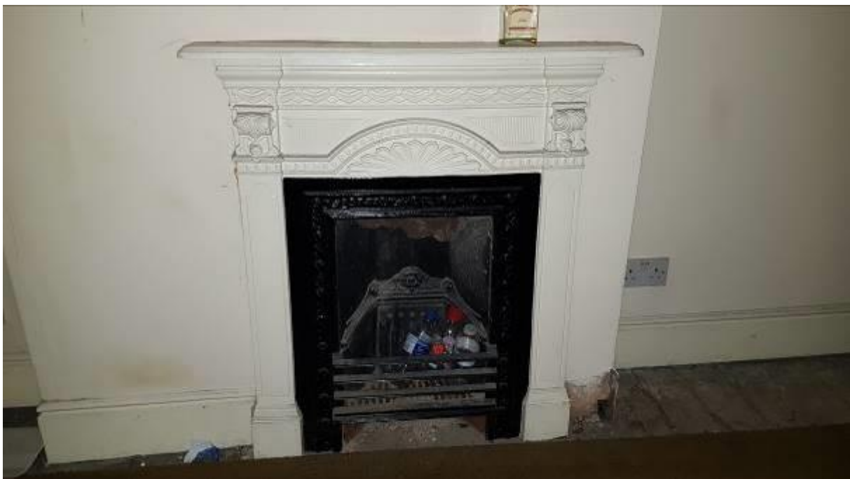
Plate 28: bedroom 3. Fireplace, grate and surround. No scale.
