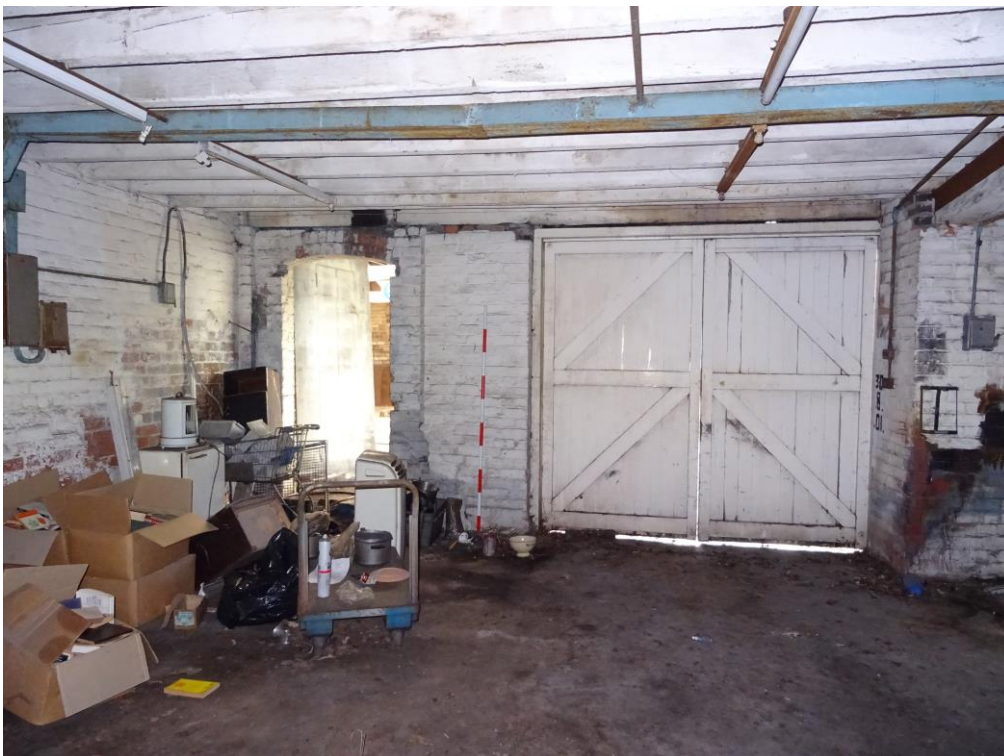
Plate 35. Exit to courtyard from section A. 2m scale.
