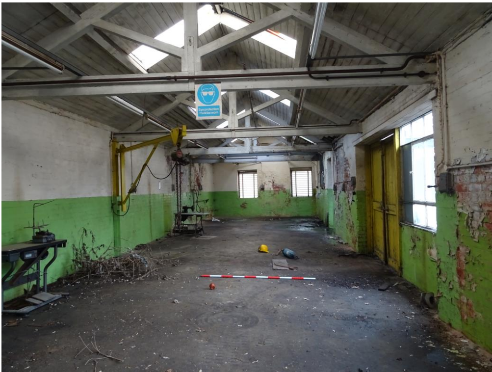
Plate 31: view west along section A. 2m scale.
