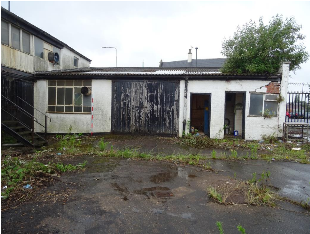
Plate 11: front of north and west facing workshop. 2m scale.
