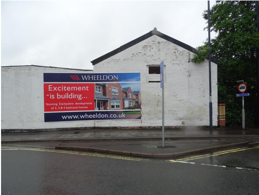
Plate 28: exterior brickwork of western elevation. 2m scale.
