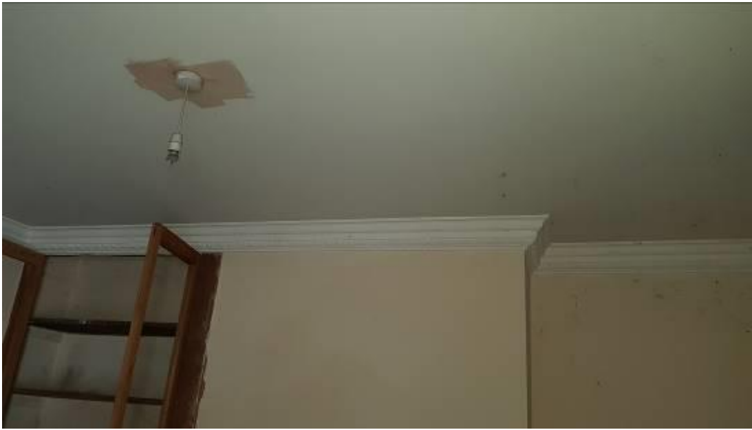
Plate 14: living room cupboard and cornice (lower floor). No scale.
