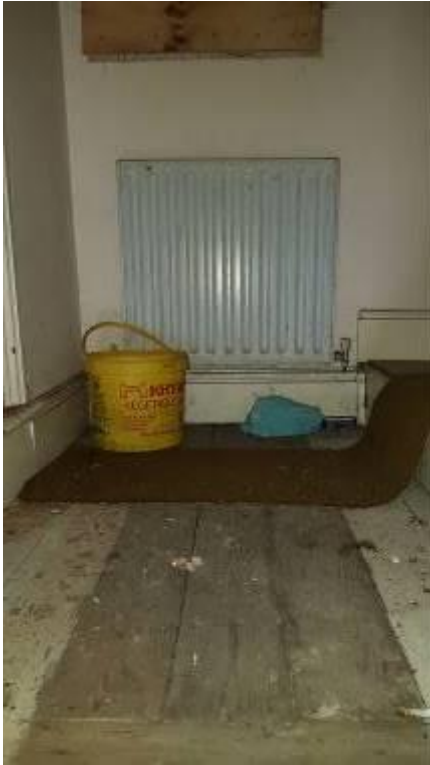
Plate 20: landing between bedroom 1 and 2*
