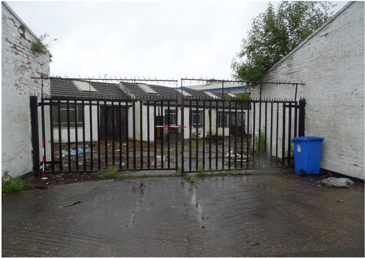
Plate 8: front entrance off Mansfield Road. 1m scale.
