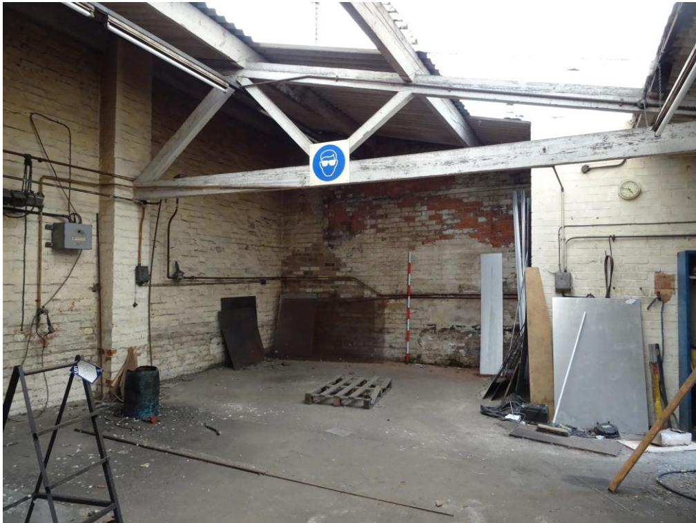
Plate 46: Section D looking toward northern gable end. 2m scale.
