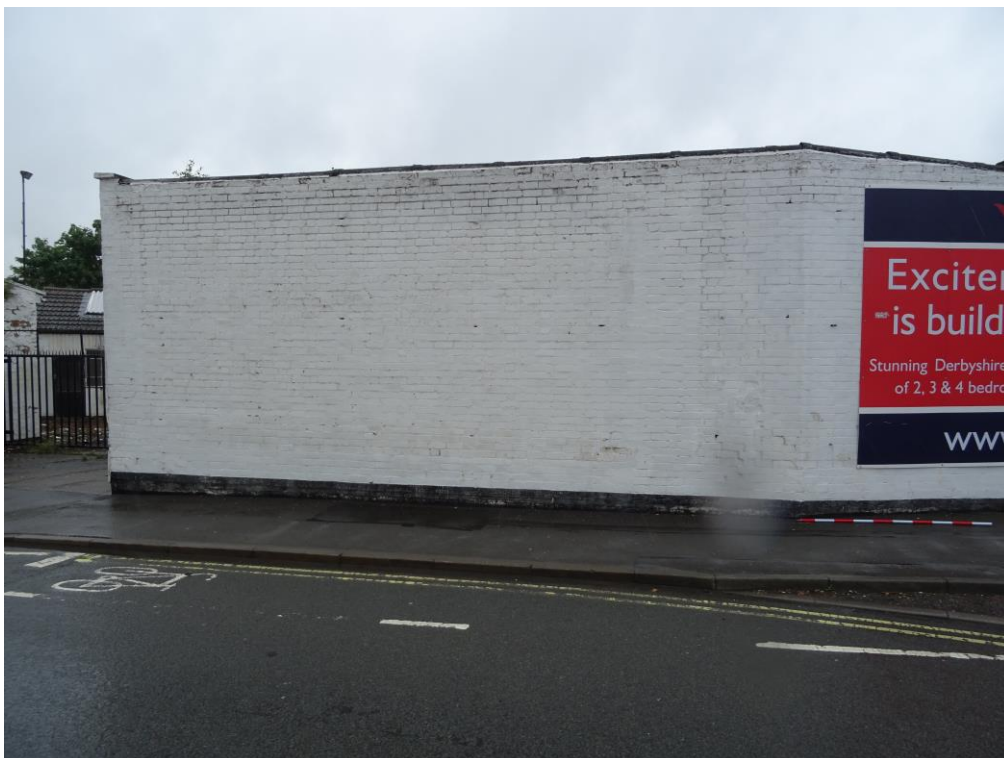
Plate 29: exterior brickwork of western elevation. 2m scale.
