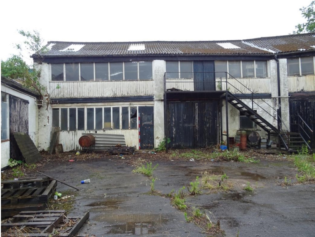
Plate 10: main workshop building: 2m scale
