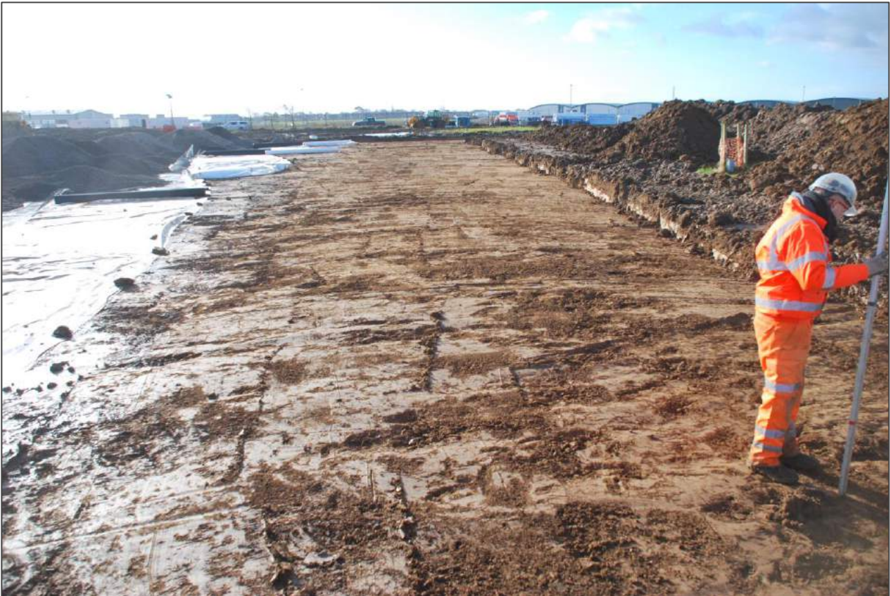
Figure 5 West of site during topsoil strip looking south
