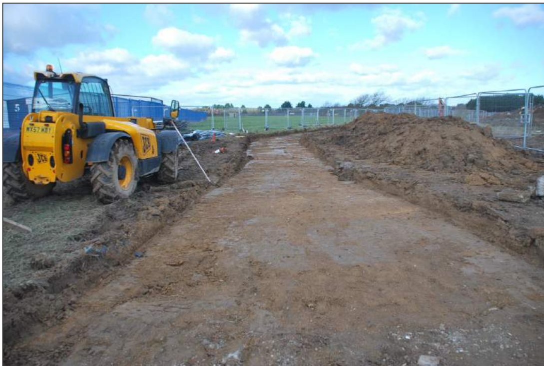
Figure 11 South of haul road looking north east
