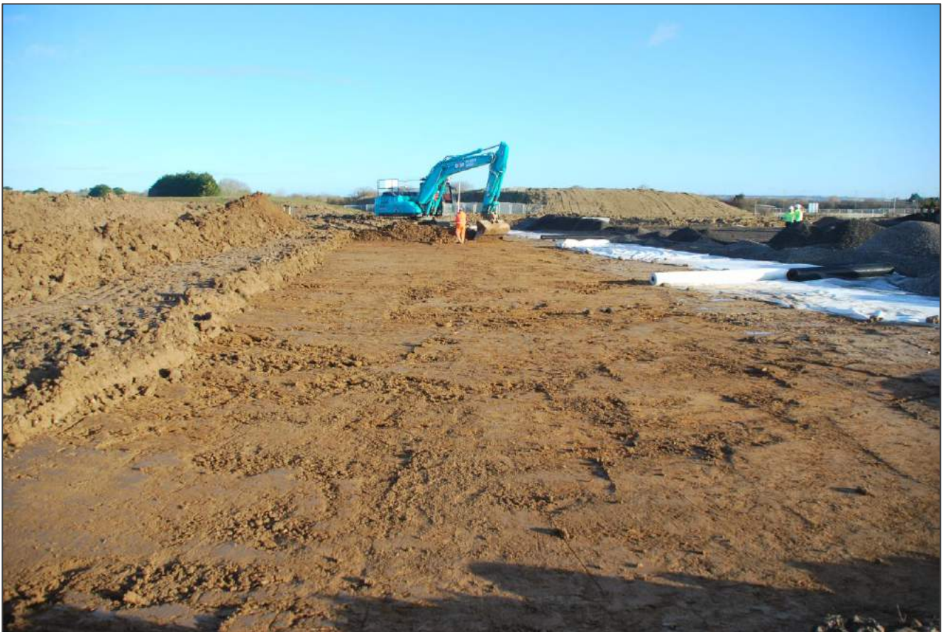
Figure 4 Centre of site during topsoil strip looking north east
