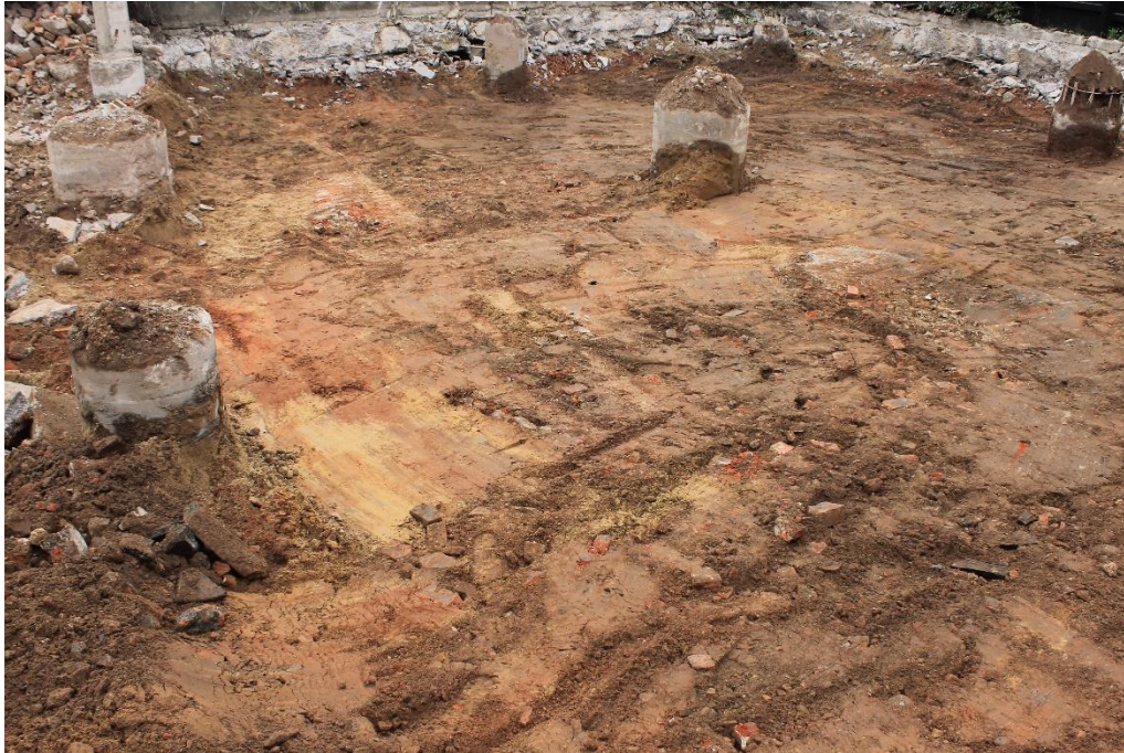
Figure 4-15 Area Around ATP7-ATP12 Stripped to Formation Level
