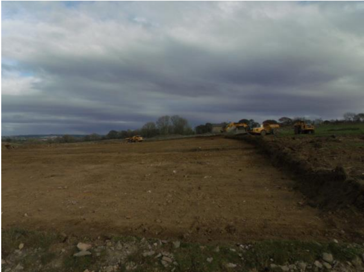
Figure 4 Completion of 4 th strip 24/10/15 looking east toward North Side West farm
