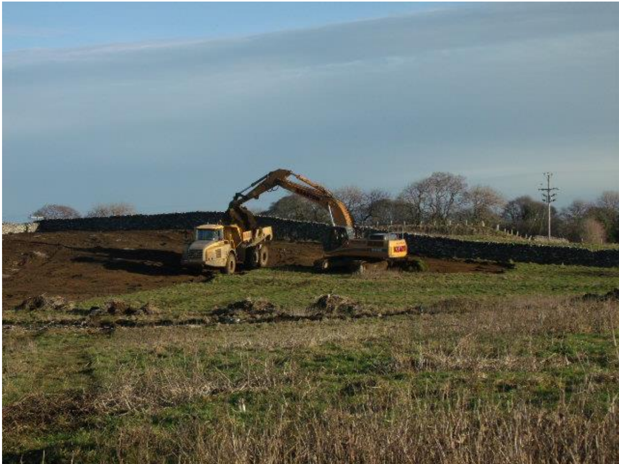
Figure 8 Completion of 8 th strip 5/12/14 looking north-east showing power lines
