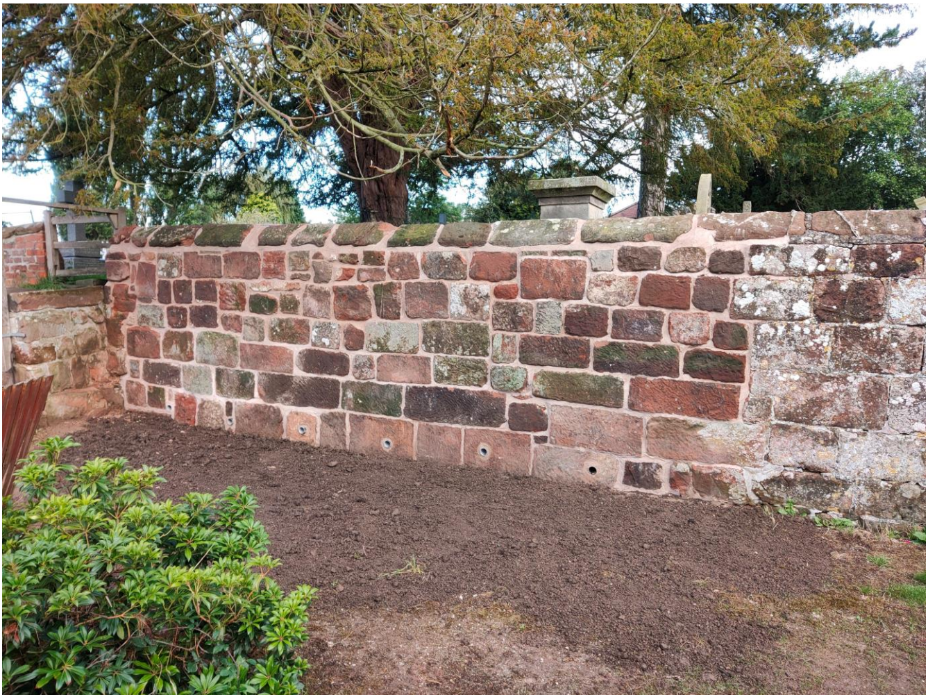
Figure 12 Rebuilt graveyard wall
