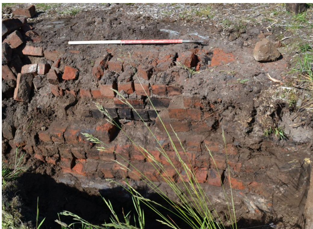
Plate 1: Foundation wall [021] in test pit 1.5
