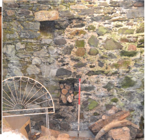
Plate 9: Blocked hole & raised flue on internal face of northern gable
