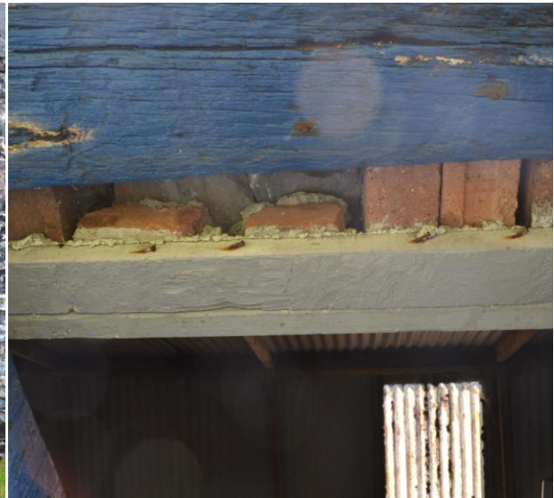
Plate 7: Brick repairs to wooden door lintel
