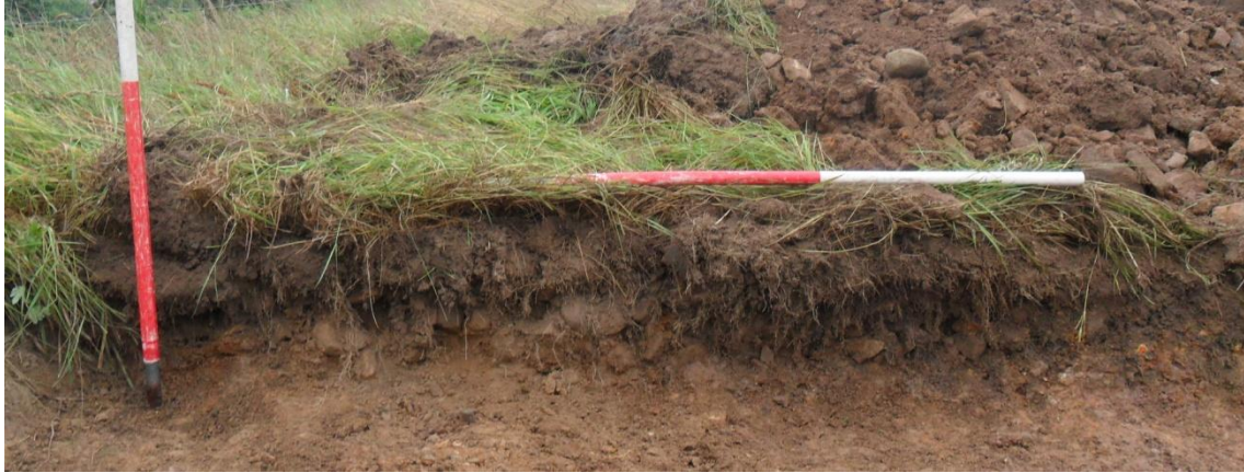
Plate 1: North-west facing section through possible rough track surface (016)
