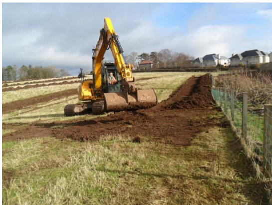
Image 74 - Working shot - backfilling
