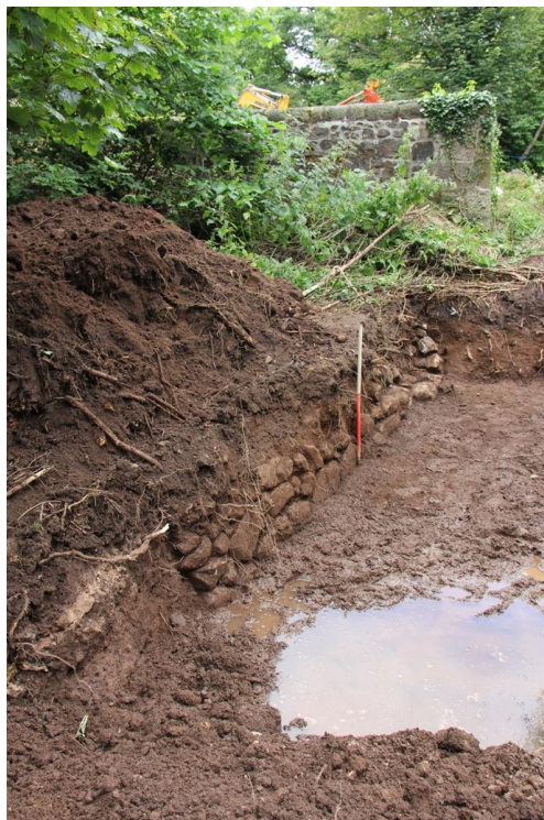
Plate 15 Test Trench C, from the south-east
