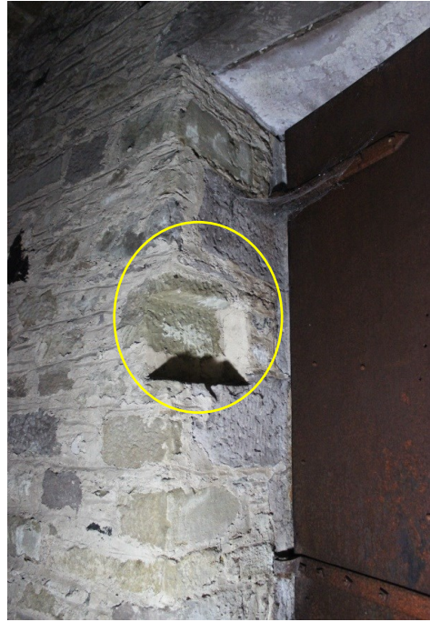
Illus. 55: Stone pocket in 006 (south)—remnant of early door/gate fitting.
