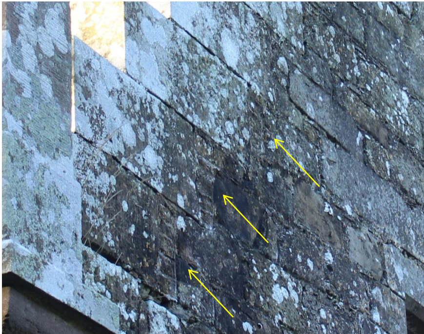
Illus. 24: Detail of stonework pinning on east gable.
