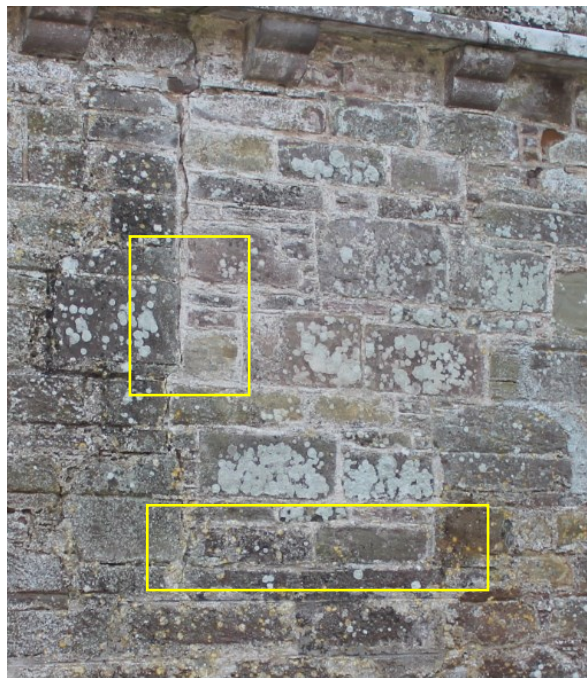
Illus. 39: Detail showing possible sill and jamb 040 .
