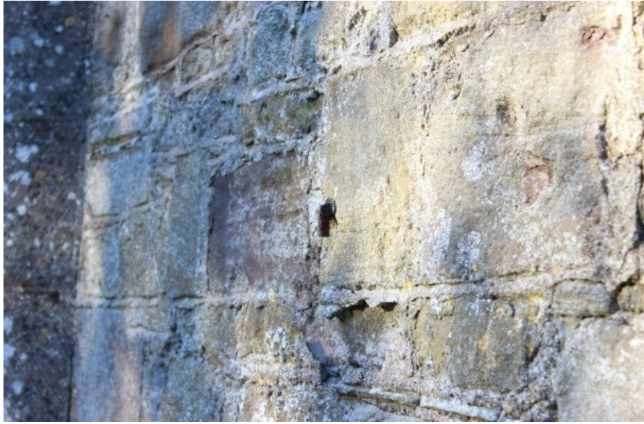
Illus. 21: Metal fittings near Window 012.
