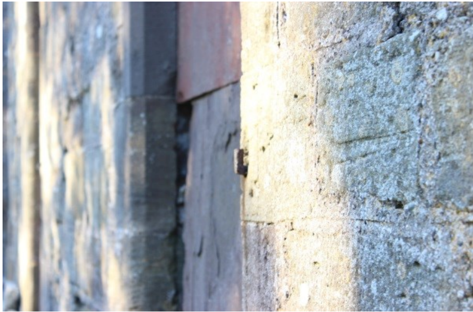
Illus. 22: Metal fittings near Window 012.
