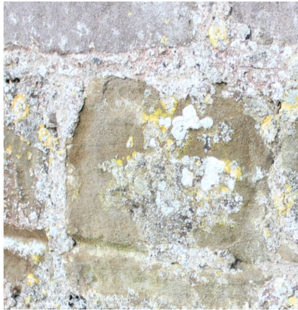
Illus. 38: Detail of the pronounced pointing on stonework rebuilt 032 and 037 .
