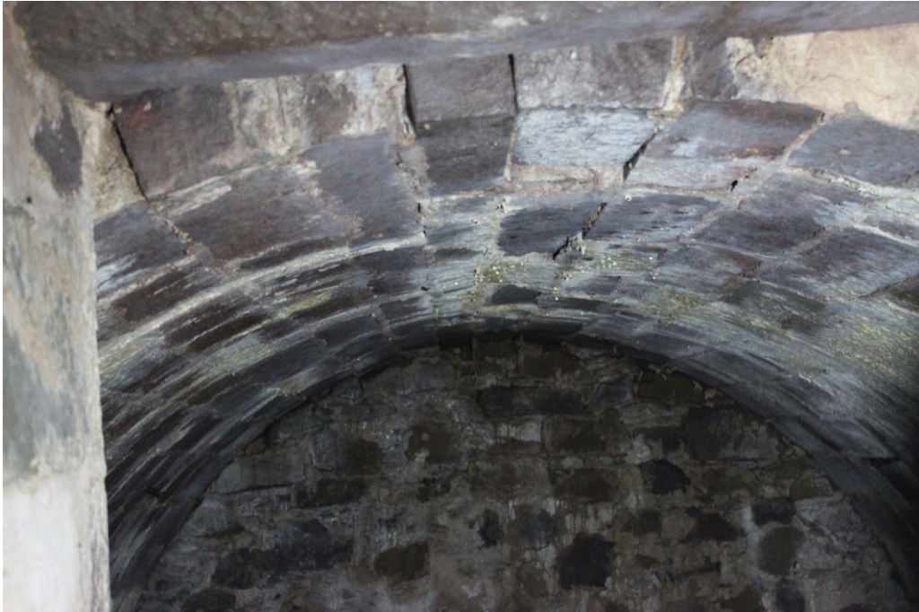
Illus. 59: View of barrel vault 060 , showing clearly that it is an inserted feature.
