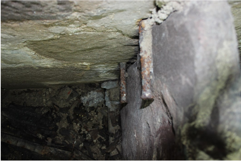
Illus. 57: Heavy iron pins holding slabs 062.
