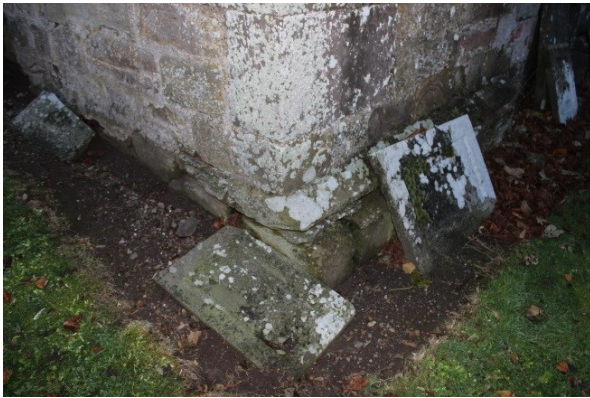
Illus. 26: Hammered foundation, south end of E gable.
