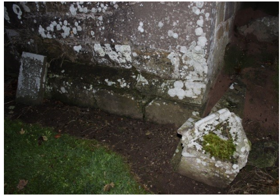
Illus. 27: Hammered foundation, north end of E gable.
