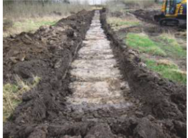
017 - Post excavation shot of trench 7 from N
