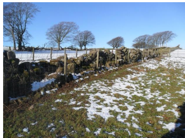
Figure 4: Dry-stone field boundary in NW corner of the development area, viewed from the SE
