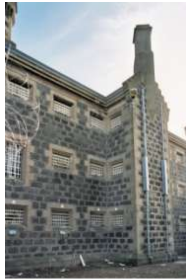
Figure 18: Salient on 'A' Hall west elevation, viewed from north (abd049p – SPS)
