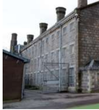
Figure 16: West elevation of 'A' Hall (from south) (Craiginches_129 - AAGM)
