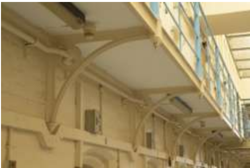
Figure 24: Gallery support brackets and balustrades in 'A' Hall (DP_172982 – RCAHMS)
