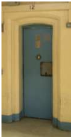
Figure 30: A typical cell door in 'A' Hall (172972 - RCAHMS)
