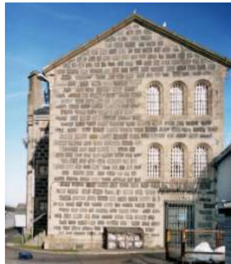
Figure 34: 'B' Hall southern elevation (abd060p - SPS)
