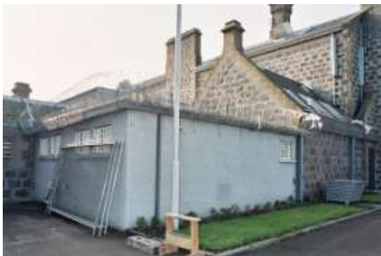
Figure 35: North elevation, recent photograph (abd066p - SPS)
