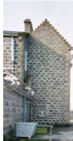
Figure 38: Details of 'B' Hall north elevation and east gable (abd064p - SPS)
