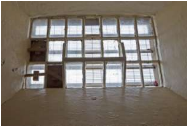
Figure 17: A typical window with locked hopper in a cell in 'A' Hall (Craiginches_012 - AAGM)
