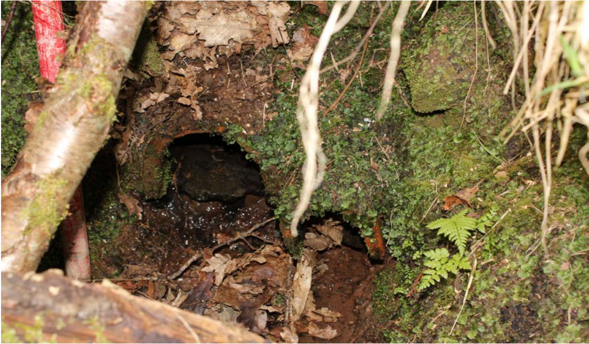
Plate 8: A close up detail of the horse shoe shaped, ceramic drains (Site 12).
