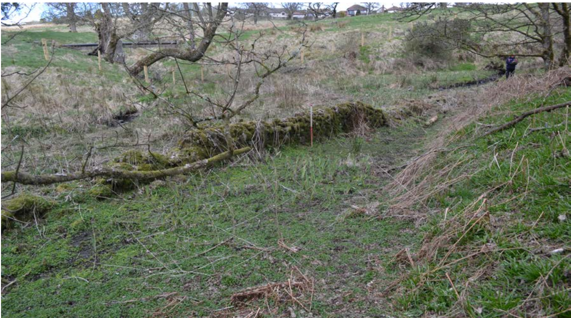
Plate 7: The drystone wall on the flood plain of the burn (Site 11) from the south east.
