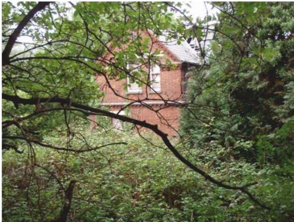
Pl. 10 Cottage rear (south-west) elevation
