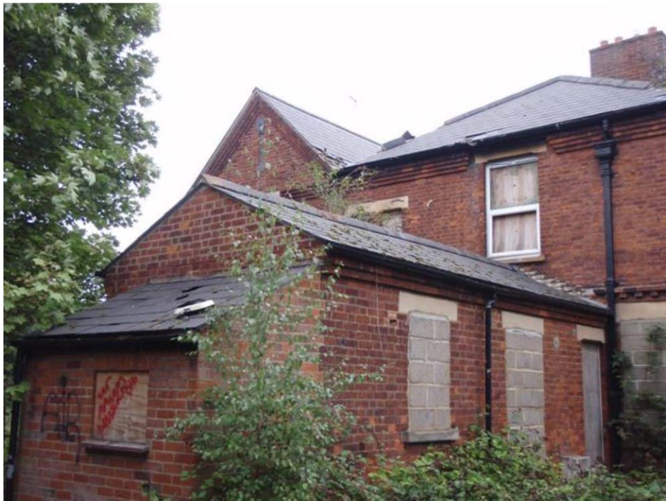
Pl. 4 Victoria House rear (south-west) elevation showing single-storey scullery and coal store and pent-roofed WC.
