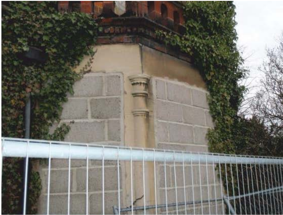
Pl. 7 Ground floor bay window west of the front door
