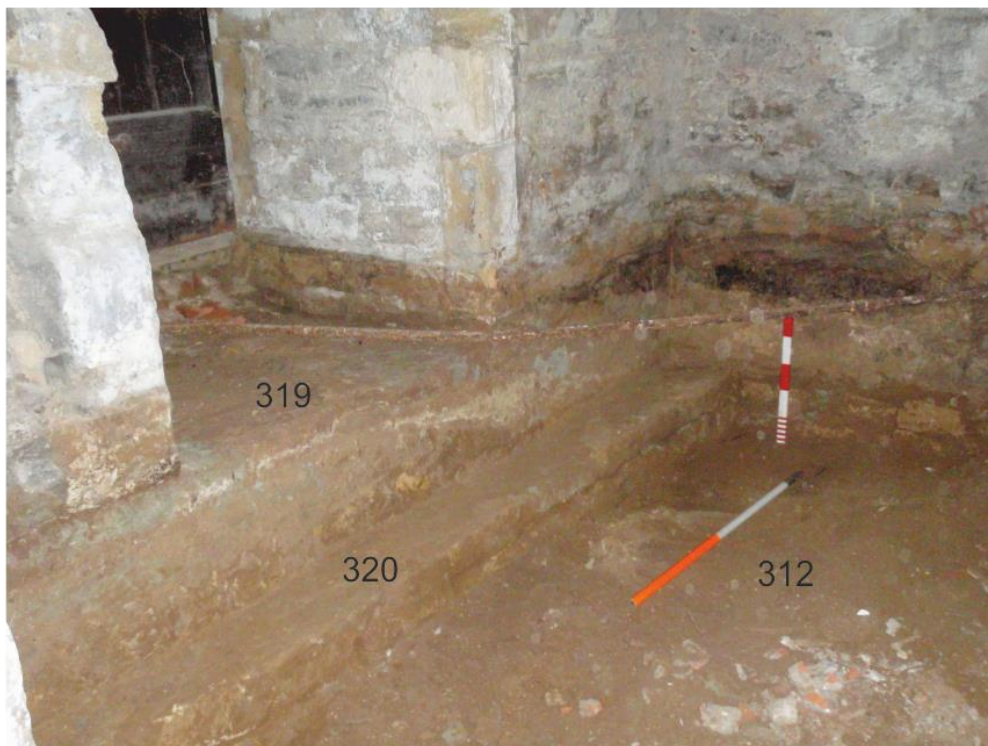
Pl. 62 Tower foundations in the south and west walls, looking south-west. Scales 1m and 0.50m
