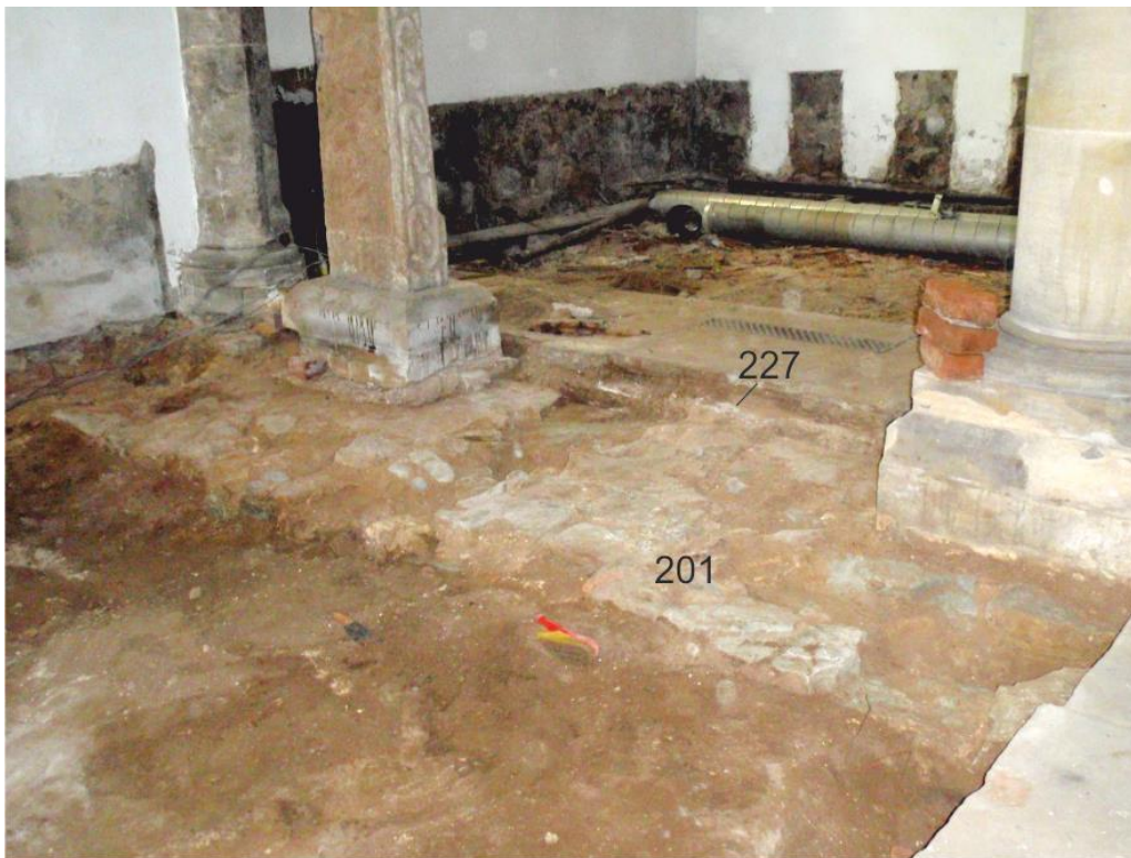
Pl. 11 General view of north-west corner of the nave after cleaning showing the nave north wall beneath the aisle arcade and the Crowle Stone, looking north-west
