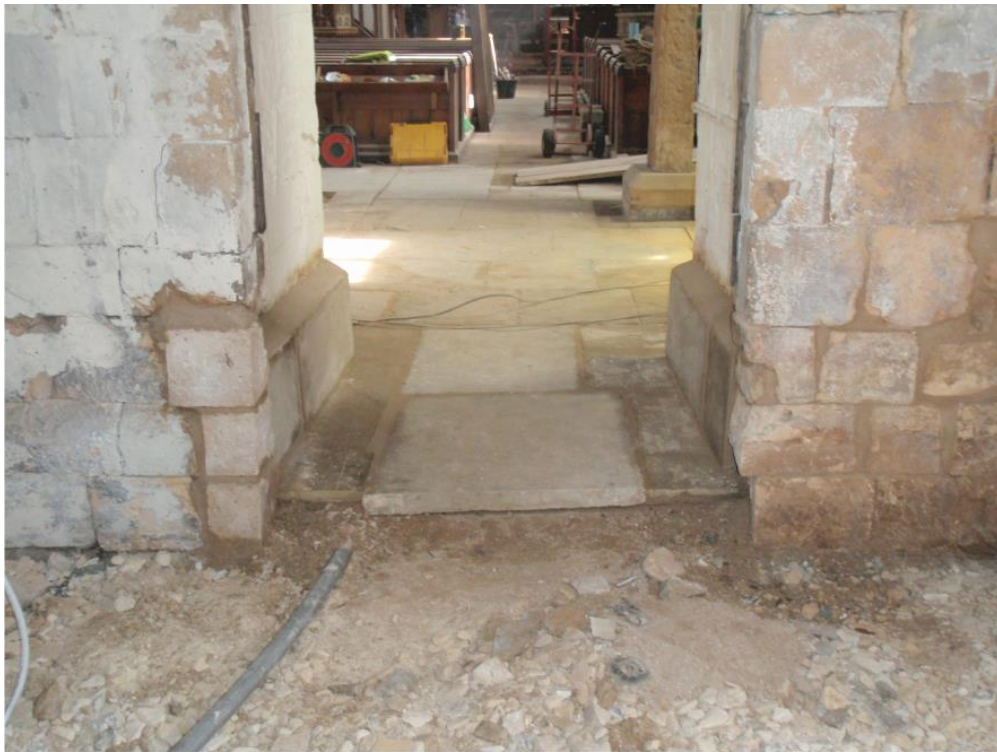
Pl. 71 Tower west door after rebuilding, looking east into the nave.
