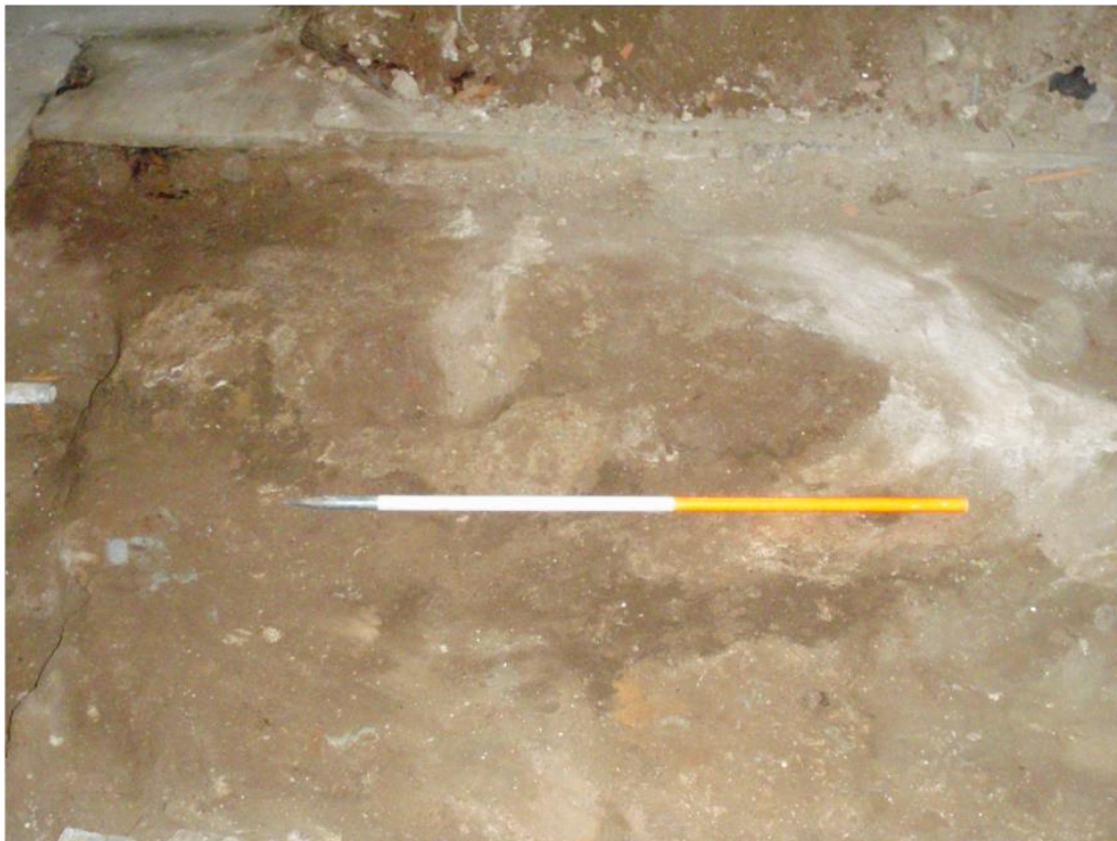
Pl. 18 Mortar patch 206, looking south. Scale 1m
