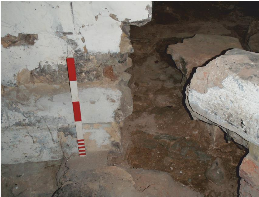
Pl. 67 Detail of north-west corner of opening showing damage caused by insertion of heating pipes, looking east. Scale 0.50m
