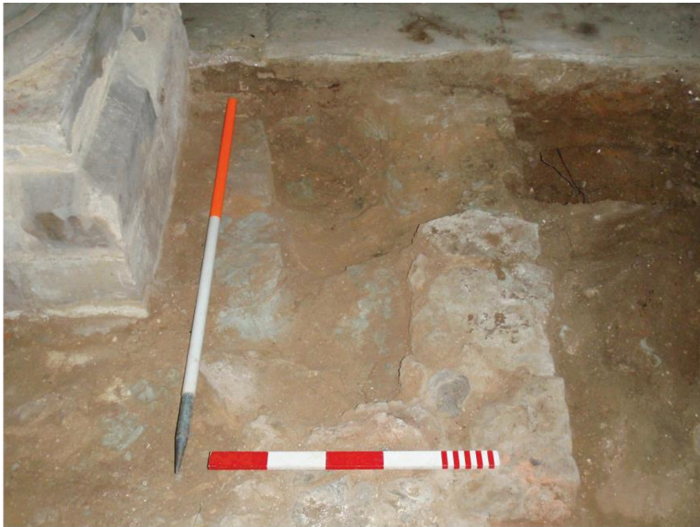
Pl. 13 Damaged area of wall 201 for pew support, looking east. Scales 1m and 0.50m
