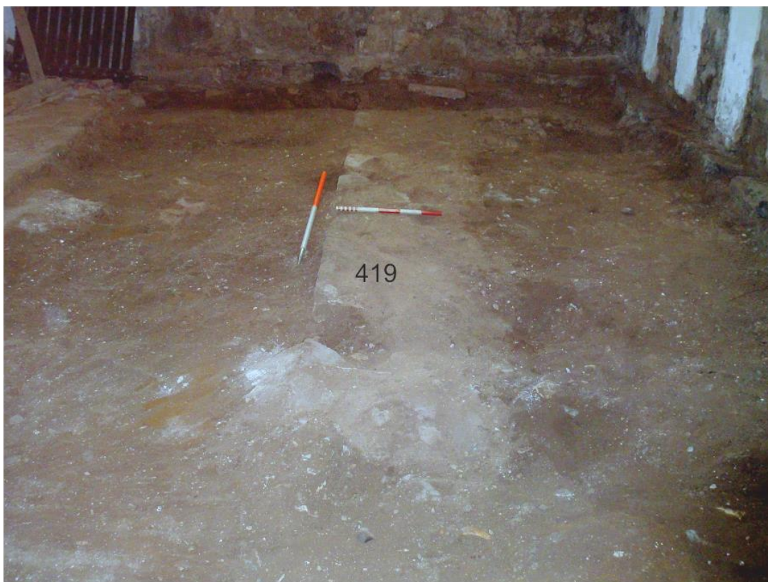
Pl. 46 Wall foundation of north wall of medieval north aisle, looking west. Scales 1m and 0.50m.
