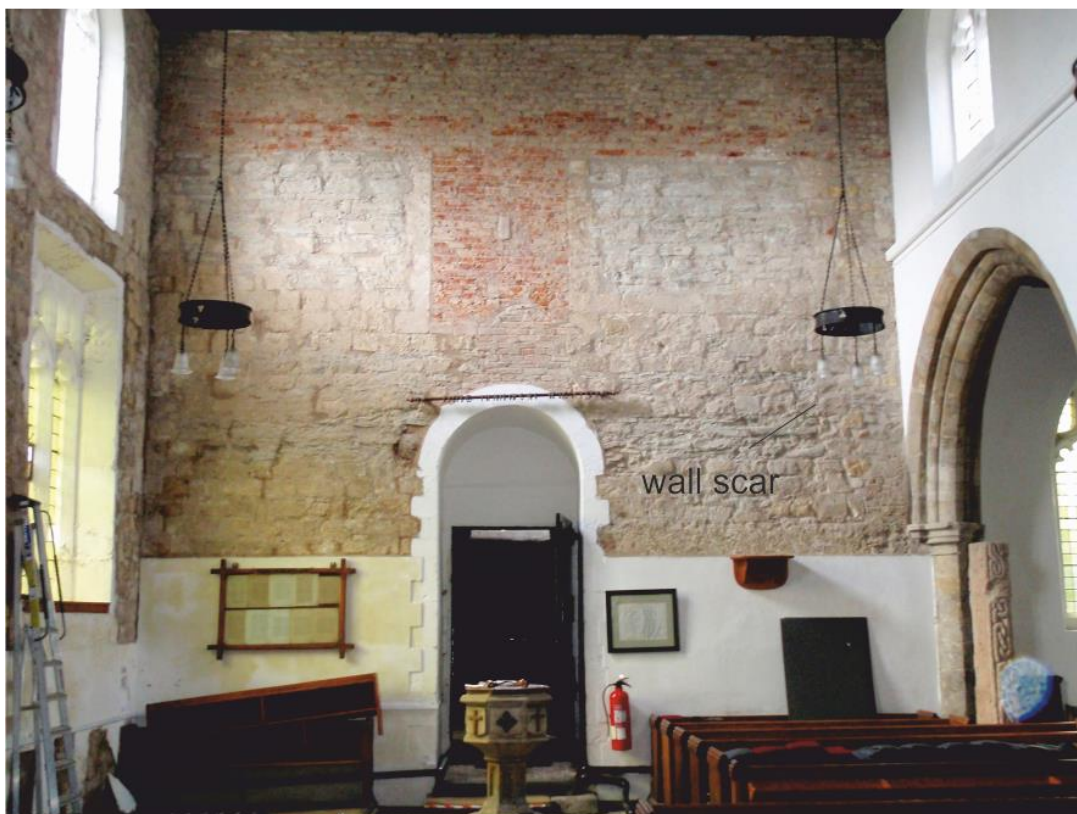
Pl. 16 Nave west wall showing wall scar for original position of the nave north wall
