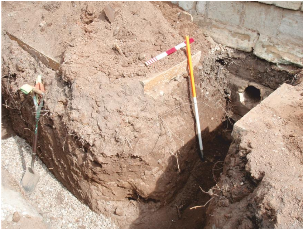
Pl. 83 Pipe trench at junction with tower west wall, looking north-east. Scales 1m and 0.50m
