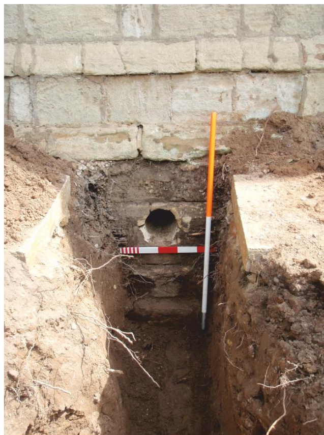
Pl. 84 Hole for service pipes in tower west wall. Scales 1m and 0.50m
