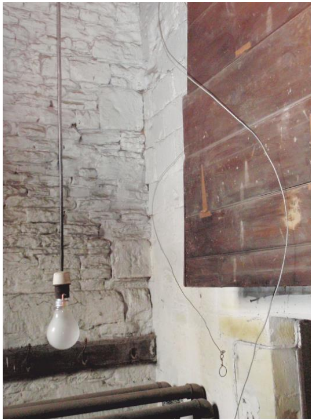
Pl. 61 Junction of the tower north wall with the earlier nave west wall, showing the contrast of ashlar blocks in the nave wall with the roughly dressed stonework of the tower wall.
