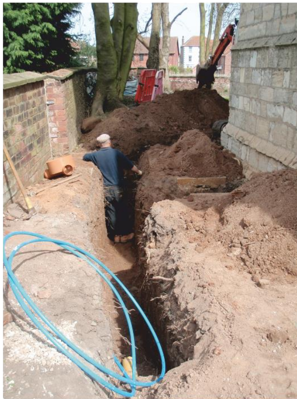
Pl. 82. Service trench on west side of tower, looking north
