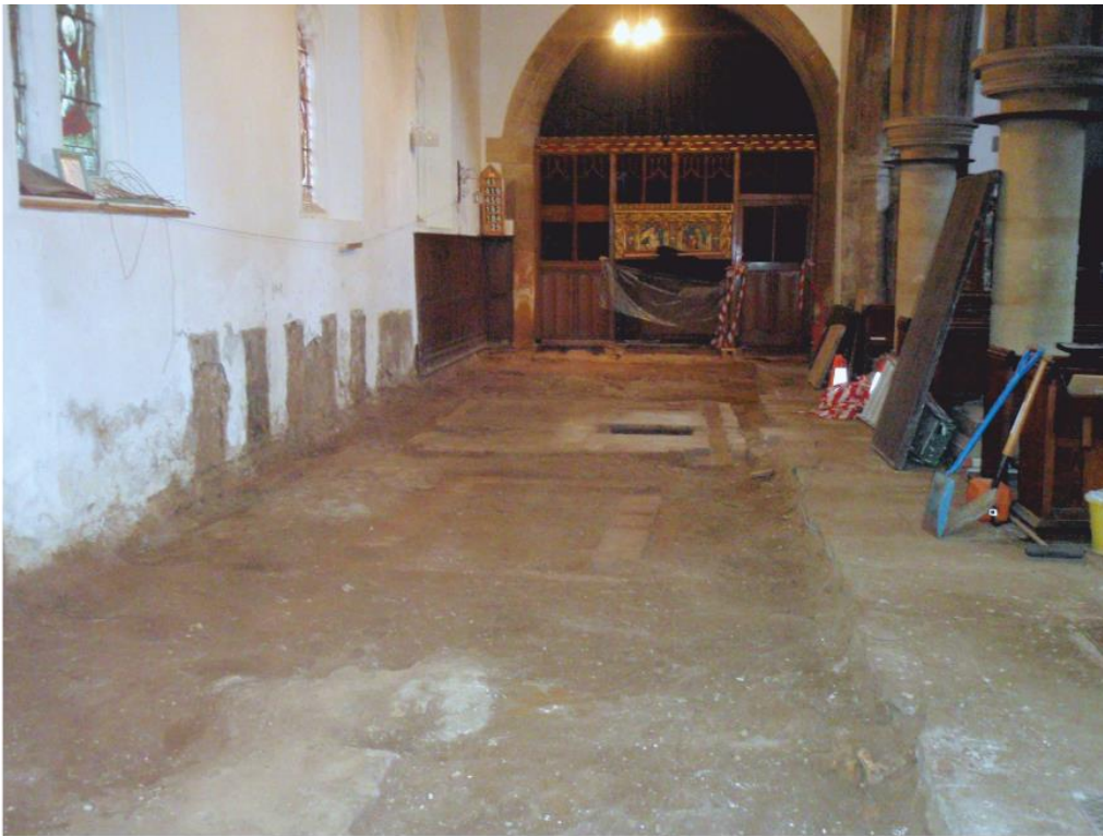
Pl. 31 North aisle after cleaning, looking east.
